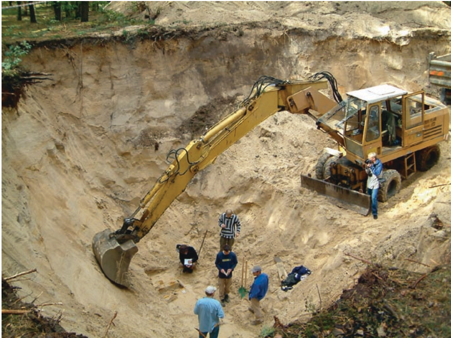
Fig. 25.4 Excavation by the authors at the site of Stalag Luft III in 2003. The excavation has reached the level of the main gallery of the tunnel “Dick”. The humic (A) and iron-stained (B) surface horizons can be seen in the back wall of the excavation, the remainder of the excavation is in glacial sands; in the excavation are assistant archaeologists Gabriel Moshenska (dark top, crouching) and Daniel Phillips (striped top, standing), and in front of them, from left to right, Larry Babits, Jamie Pringle and Peter Doyle. Visible in the excavation is the bright orange iron staining associated with the sub-gallery airline (see Fig. 25.7) (see as color plate following Index )
