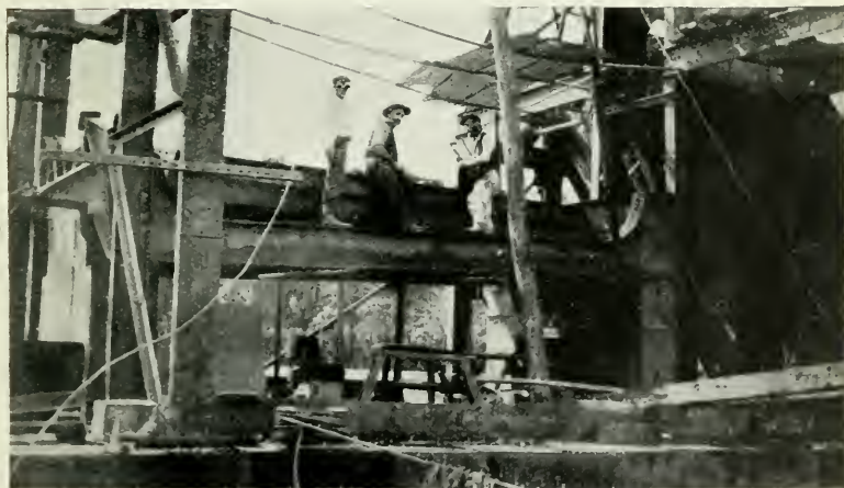
ERECTING THE DREDGE SUPERSTRUCTURE.
