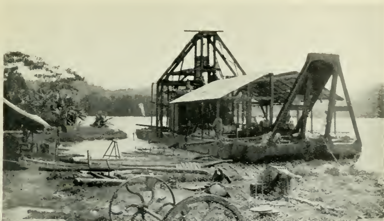
THE DREDGE NEARING COMPLETION.
