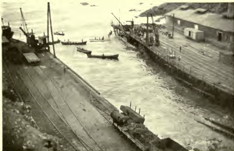
THE PORT OF MOLLENDO: MOLE AND BREAKWATER IN CONNECTION WITH THE SOUTHERN RAILWAY.
