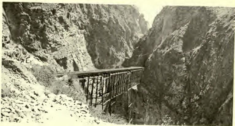
PUERTE DE CHAUPICHACA, ON THE LINE OF THE CENTRAL RAILWAY.
