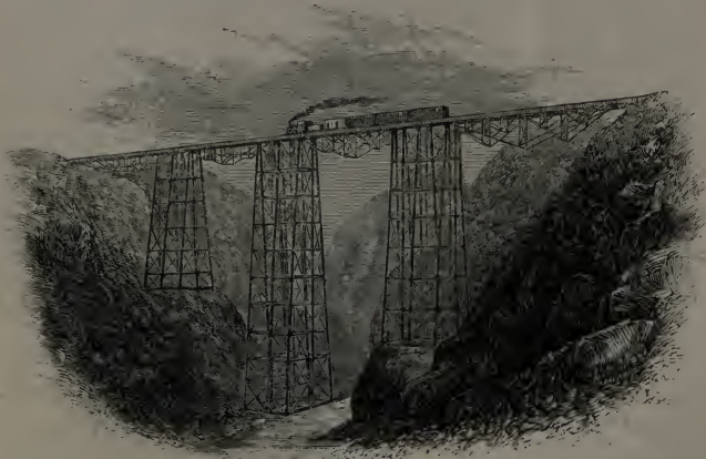
RAILWAY BRIDGE OVER VERRUGAS RIVER.
