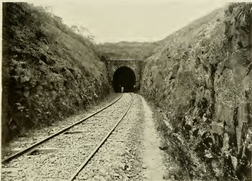
TUNNEL AT BAÑADA DE ROCHA.
