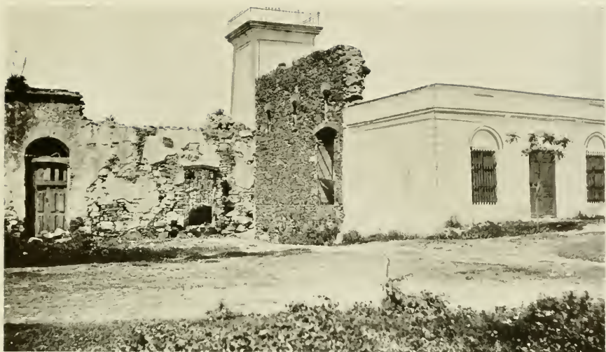
COLONIA : RUINED FORTRESS WALL.
