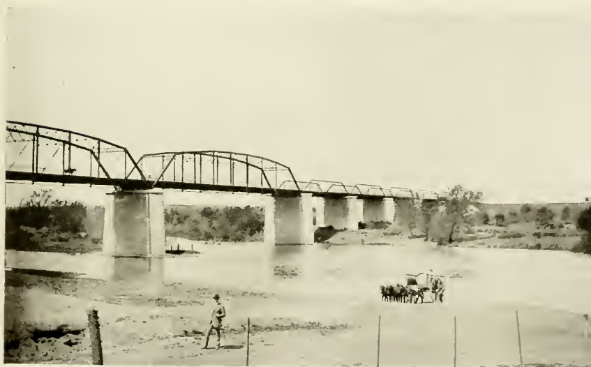
THE SAN JOSE ROAD BRIDGE.
