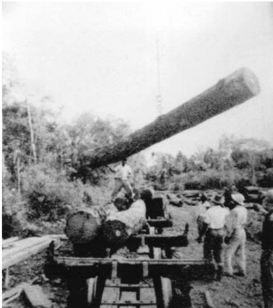
Figure 2. Mahogany log being loaded onto the narrow gauge that ran between Hillbank and Gallon Jug. (Courtesy Belize National Archives, Belmopan, Belize)
