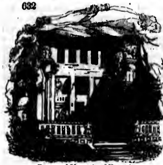
Excavated Mountain of Keeneri.
