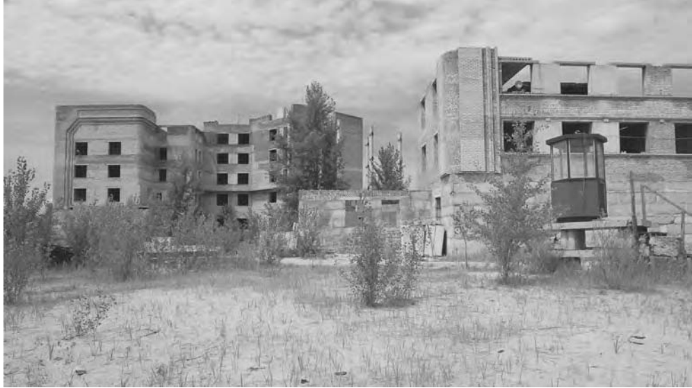
Abandoned and crumbling buildings near the Chernobyl power plant are a stark reminder of the Soviet-era disaster in the Ukraine.
