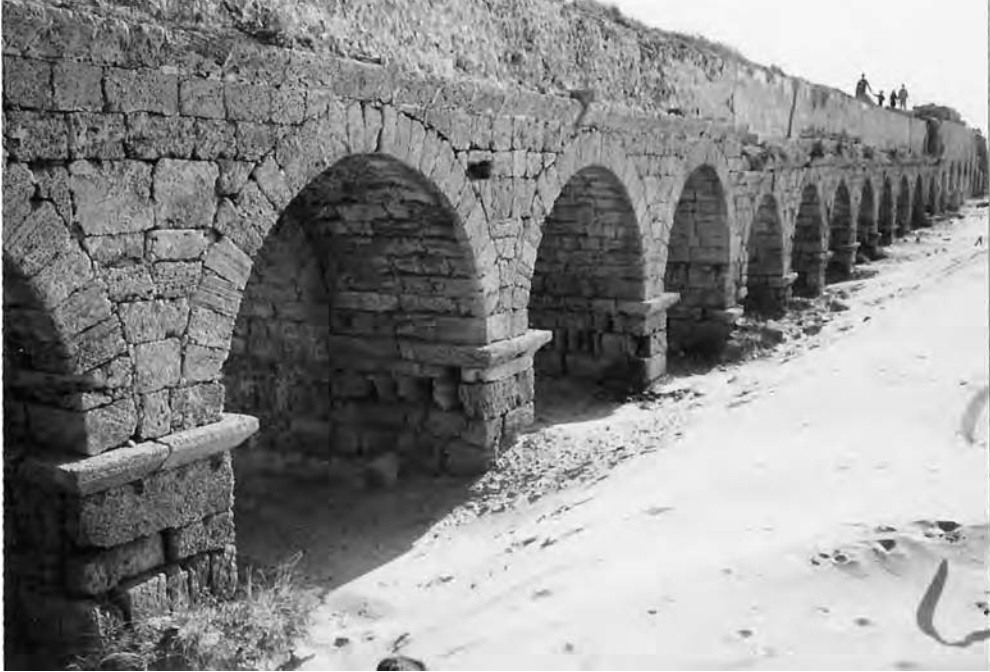
Romans constructed this aqueduct in 22 B.C.E. near Caesarea, a town now located in Israel between Tel Aviv and Haifa (photo by Paul A. Tucci).
