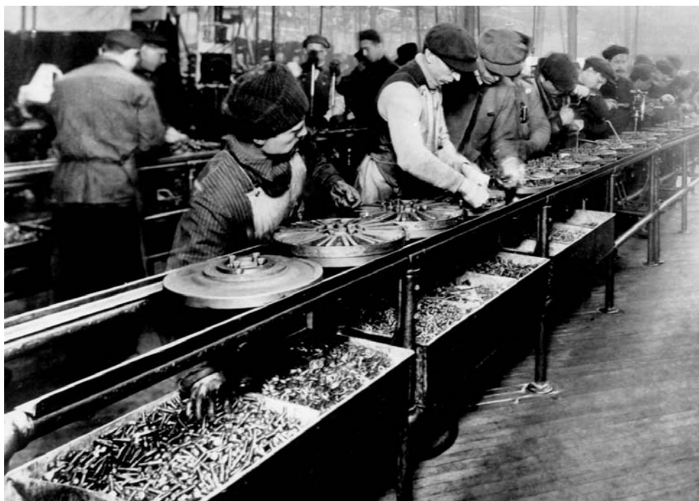
Ford workers on a flywheel assembly line, 1913. Henry Ford is credited with the creation of the assembly line, an industrial innovation that allowed cars to be produced quickly and efficiently.
