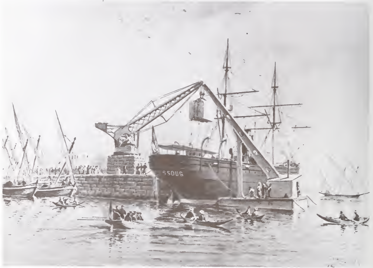
The 50-ton pedestal about to break loose over the stern of the Dessoug
