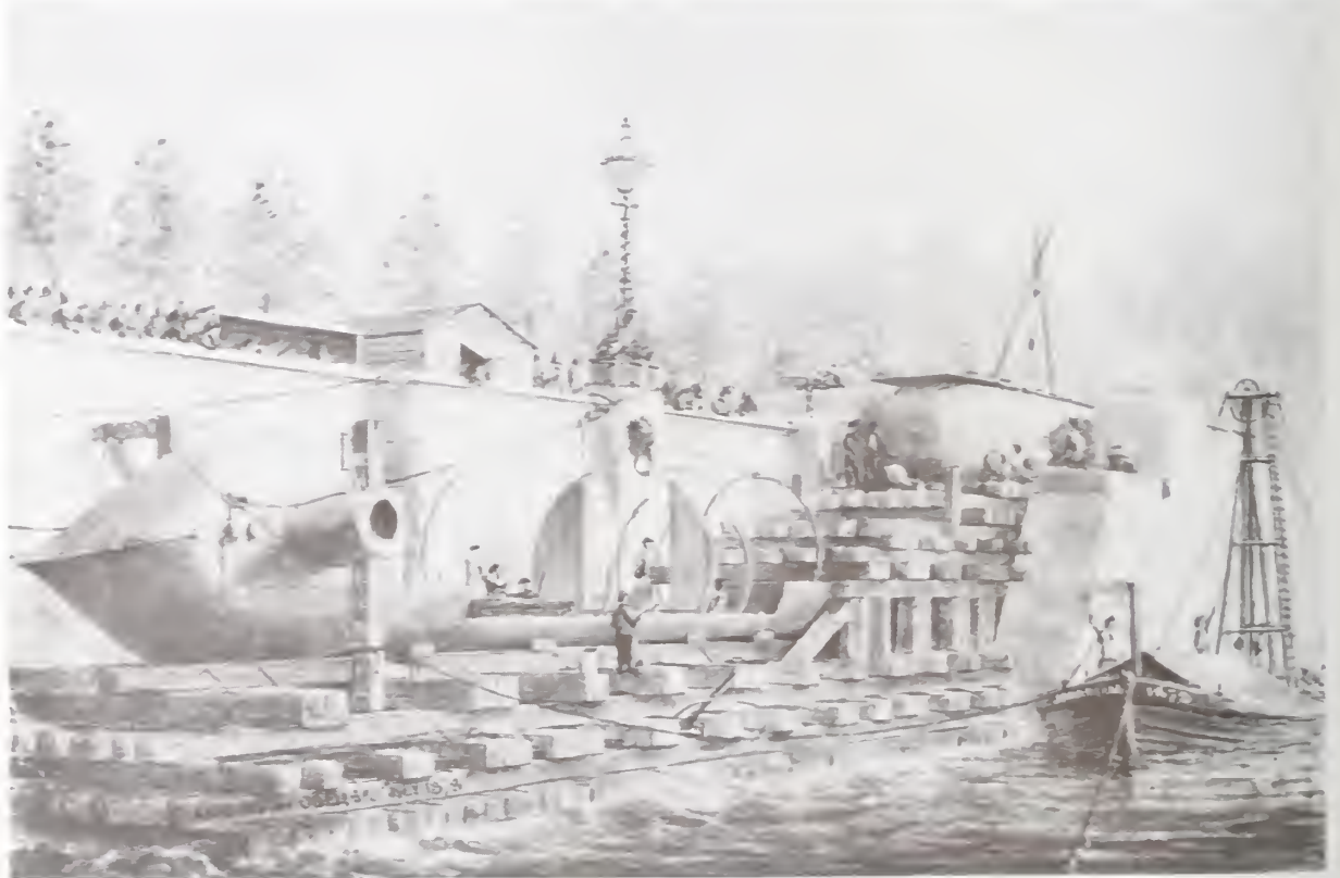
Dismantling the cylinder
