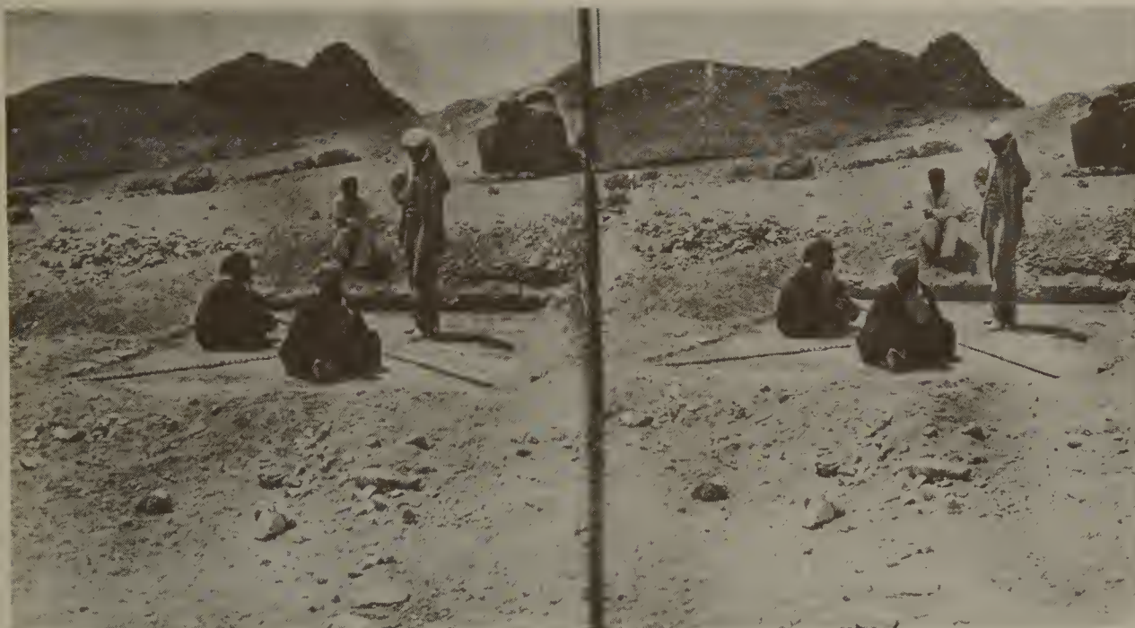
Stereographic photo taken by Piazzi Smyth of Mr. Inglis and Arab workers in the northeast socket cleared in April of 1865. The Royal Engineer surveyor went all over the floor of the socket with a spirit level and found it absolutely level.
