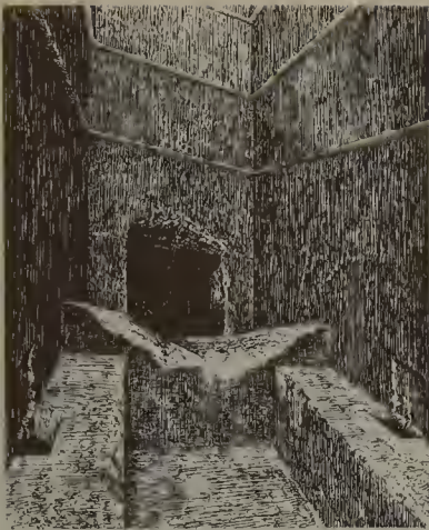
At the top of the Grand Gallery lies a huge stone step, 6 feet wide, 3 feet high, which blocks the Ascending Passage and forms a platform 8 feet deep, now badly chipped and worn.
