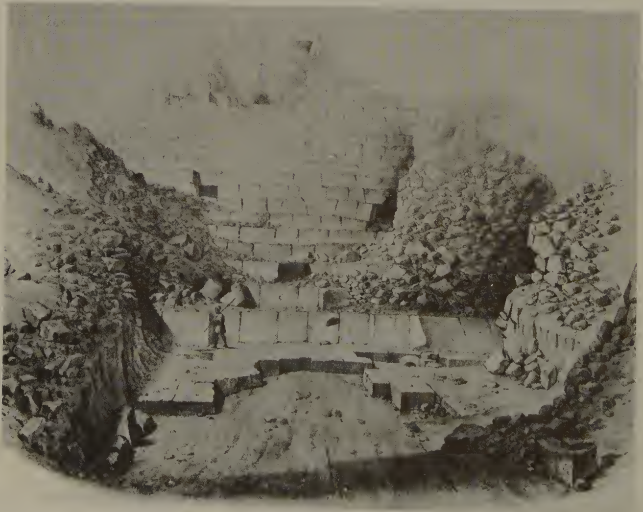
Casing stones and pavement as exposed by Howard-Vyse. Both entrances can be seen, Al Mamun's on the sixth course, and the original entrance ten courses higher.
