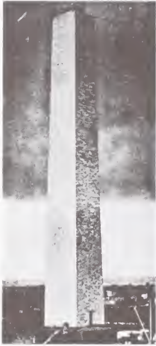
During the entire construction of the monument it settled only 4 inches. In the end, its 81,720 tons were so well distributed that a 145-mile-an-hour wind—almost three times the wind pressure that might be expected—would not topple it. A 30-mile-an-hour wind would only cause the shaft to sway .125 inches at the peak.
