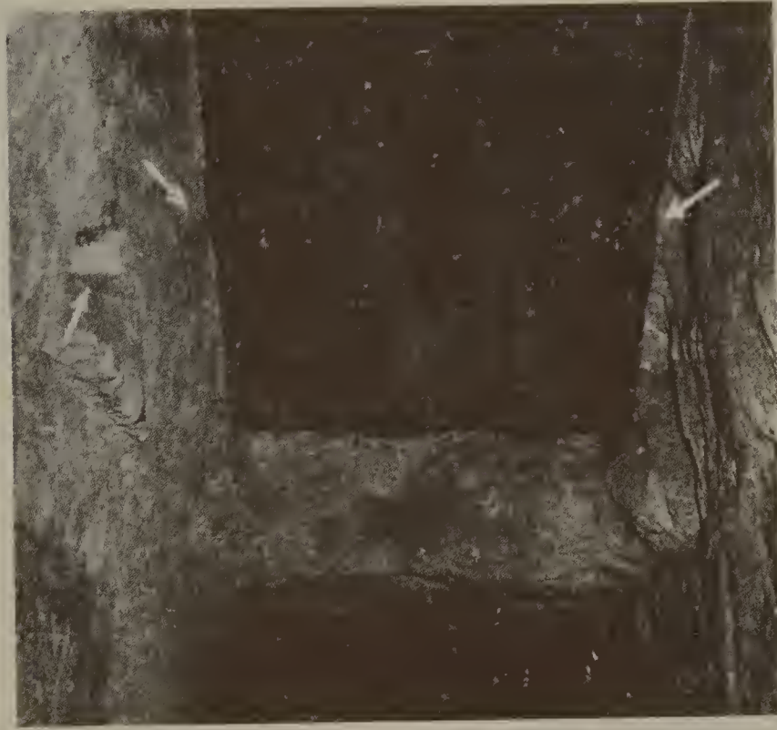
Goyon's arrows indicate slots in the granite plug for the insertion of wedges to control its downward movement.
