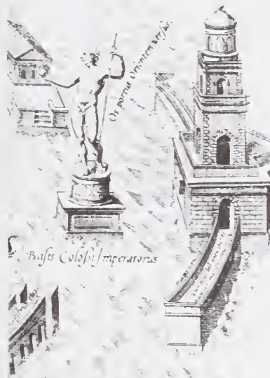
Towered docks at Rome's harbor, built by the emperor Claudius
