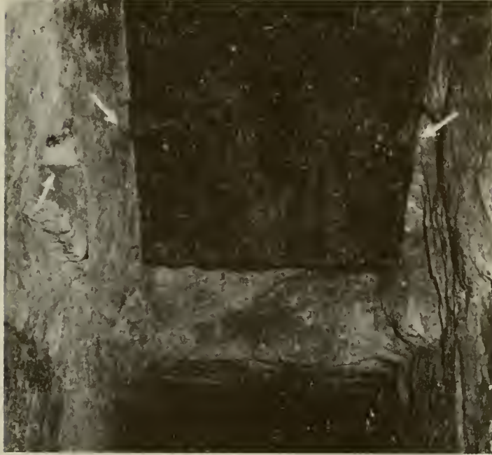
Goyon's arrows indicate slots in the granite plug for the insertion of wedges to control its downward movement.
