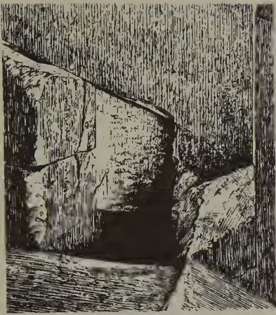
Entrance to the "well."
