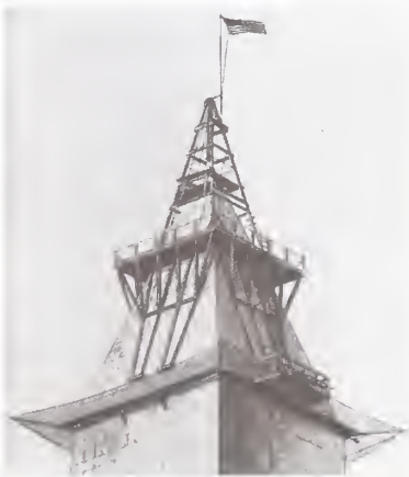
The pyramidion in place with security scaffolding and net ready for the Masonic ceremony of laying the aluminum capstone. This pyramidal capstone consisted of 3,765 cubic feet of dressed marble in 262 separate pieces which took thirty days to set. In December 1884 it was successfully raised without incident.
