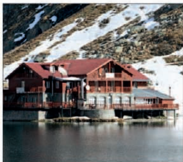
Mountain huts , or cabanas , are available on the northern side of the Făgăraș ridge, offering crackling log fires, dormitory beds and simple food. However, bikers intending to climb further south will need to carry camping equipment.
