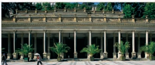
Columns of the Mill Spring Colonnade
