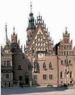
Gothic gables of the east façade of the Town Hall
