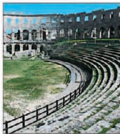
AD 81 Construction of the Roman Amphitheatre at Pula, Croatia completed (see p483)
