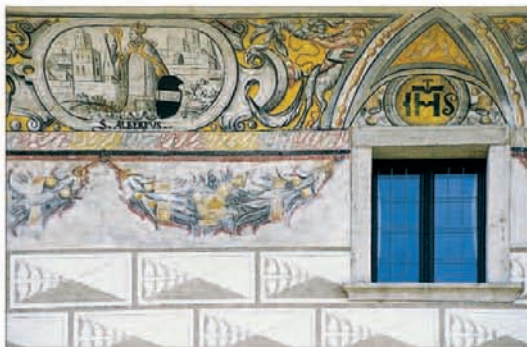
Part of the façade of the former Jesuit College in ulice Horní
