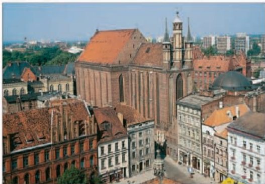
St Mary's Church, as viewed from the top of the Town Hall Tower
