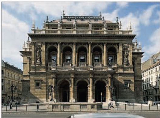
The imposing façade of the State Opera House
