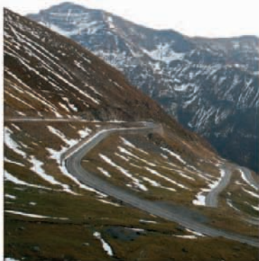
Transfăgărașan , Romania's highest road, crosses the Făgăraș Mountains and connects the regions of Transylvania and Wallachia as well as the towns of Sibiu and Pitești. The road has five tunnels; the longest is 884 m (2,900 ft).
