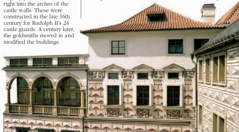
Schwarzenberg Palace in Castle Square, notable for its sgraffito decoration
