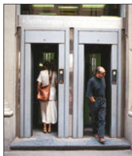
Entering and leaving a bank through an electronic double door
