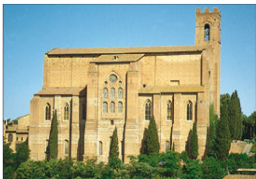
The façade of San Domenico
