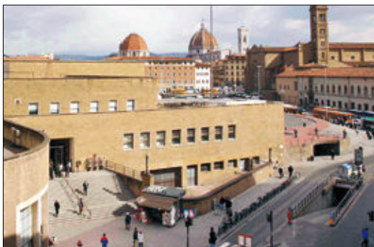
View of Santa Maria Novella railway station, Florence
