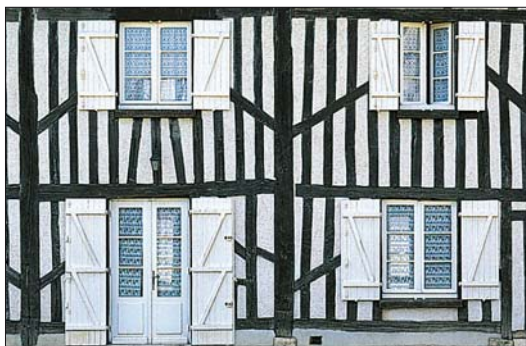
A typical, half-timbered building of La Sologne
