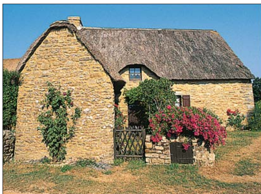
A traditional thatched house in the Brière regional park
