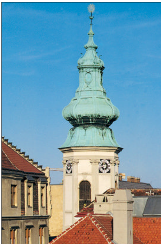
Moulded copper cupola over the tower of the Annakirche
