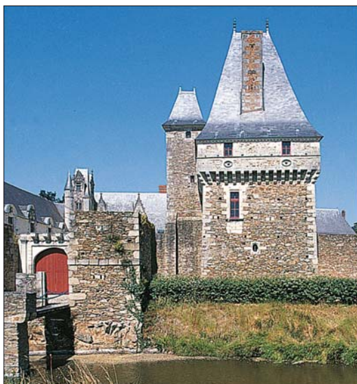
The machicolated entrance tower at the Château de Goulaine
