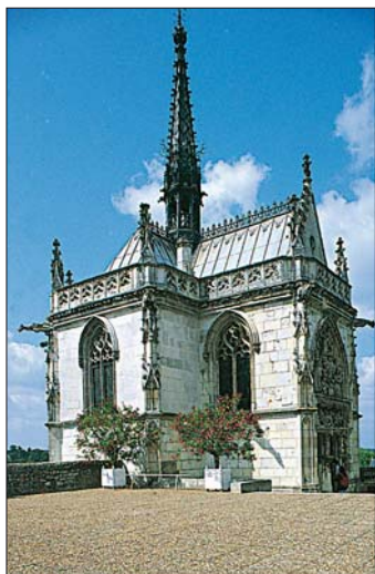
The late-Gothic Chapelle St-Hubert, with its highly ornate roof and spire
