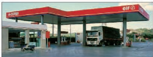
Petrol station run by the Cepsa chain
