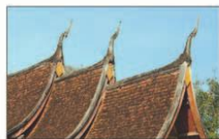
So faa are roof finials that point upward, often in the shape of a naga (serpent).
