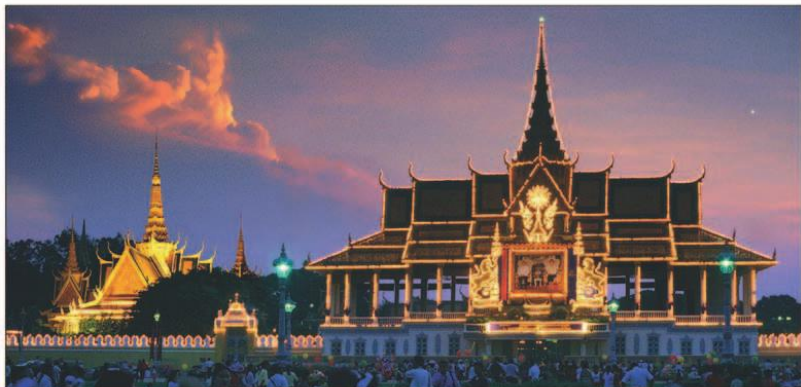
View of the elegantly lit exterior of the Dancing Pavilion at night
