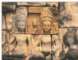
Restoration in progress at the Terrace of the Leper King
