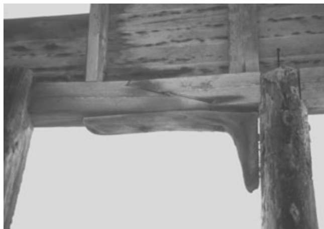
Figure 4.12 Re-used ship's timbers in an open barn on the Turks and Caicos Islands. The heavy transverse beam is part of a keel, showing a hook scarph. Roman numerals (XIX) identify the mating pieces. Below is a small knee. (Photo: Colin Martin)
