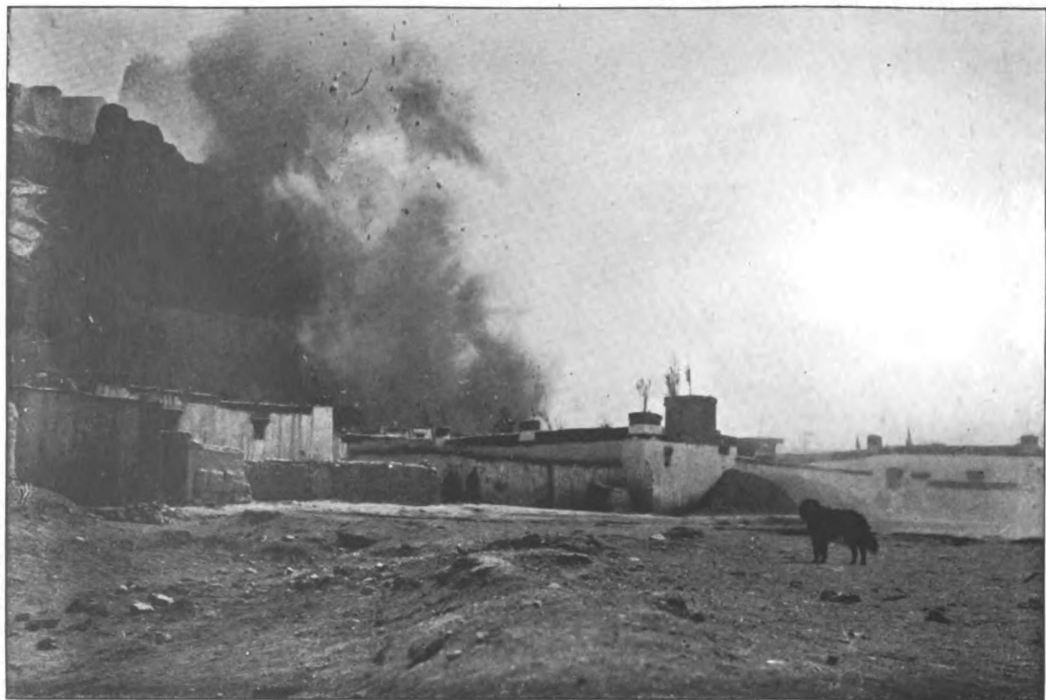
BLOWING UP OF GYANTSE FORT GATE
