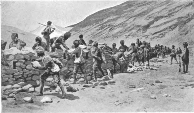
DISMANTLING LOOP-HOLED WALL AT KANGMAR
