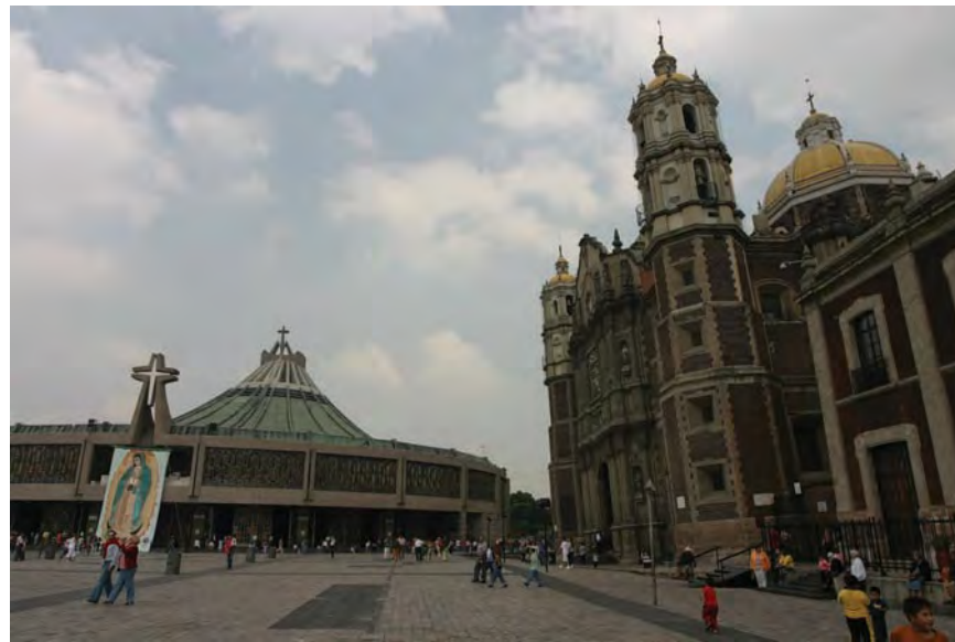
● Figure 10.1.5 Mexico City's subsidence is dramatically evident at the Shrine of Our Lady of Guadalupe, where the massive cathedral (right) has sunken sharply inward toward the plaza.
