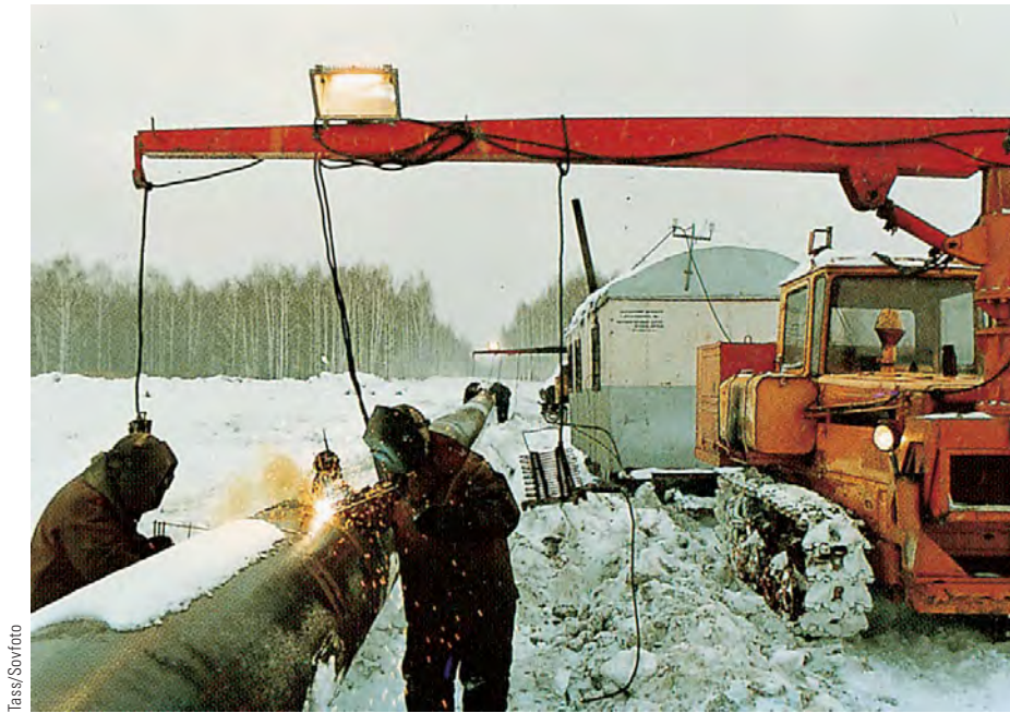
• Figure 5.1.14 Laying an oil pipeline in Russia's Northern Lands. Immense quantities of steel have been required for thousands of miles of oil and gas pipelines that have been built in Russia and the Near Abroad since World War II.
