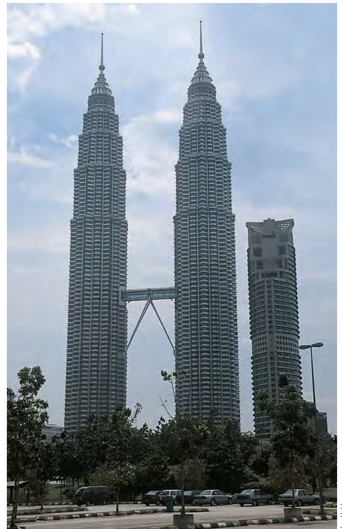
• Figure 7.2.3 Modernity and prosperity characterize some nations in Southeast Asia today. At 1,462 feet (446 m), the twin Petronas Towers in Kuala Lumpur were until 2005 the tallest buildings in the world.
