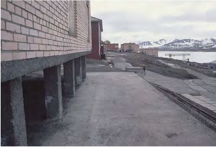
• Figure 5.5 In the High Arctic, buildings must be erected on pilings so that they do not melt the permafrost below. This is the Russian coal-mining settlement of Barentsburg in Norway's Svalbard (Spitsbergen) Archipelago.
