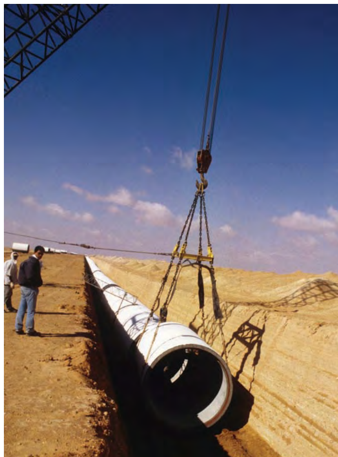
• Figure 6.1.14 Laying pipe for Libya’s Great Manmade River.
