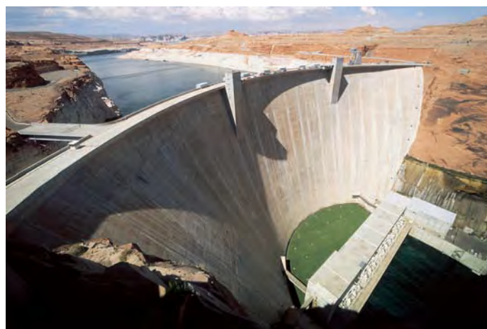
● Figure 11.2.23 The Glen Canyon Dam, just upstream from the Grand Canyon, was constructed in the 1950s. Note the low water level in this 2005 photo. A full reservoir would cover the white strip of bank that extends behind the dam.
