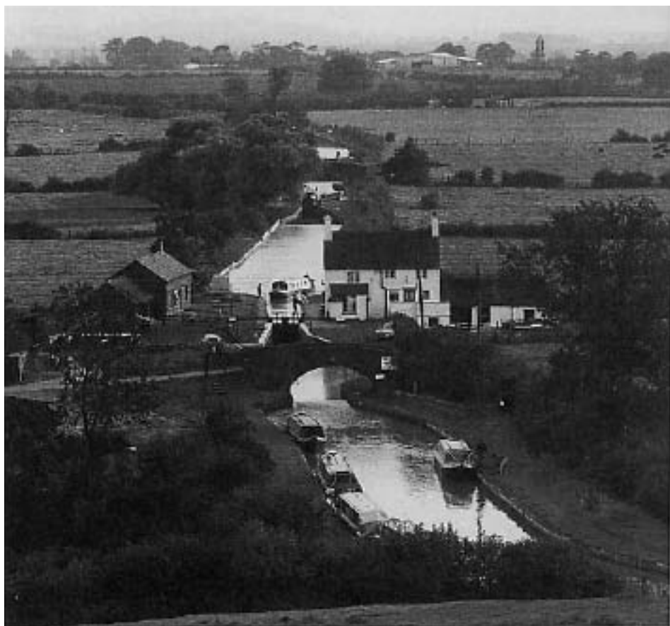
Oxford Canal lock, Warwickshire, England. The construction of canals, an endeavor begun in the 17th century, continued through the 18th century, serving as a realization of the Baconian ideal of mastery over nature. (Courtesy New York Public Library)
