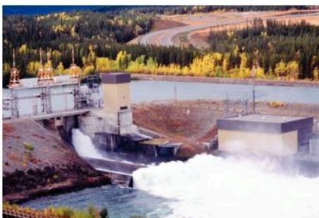
▲ Figure 18.4.3 Flowing water can be used to generate electricity
