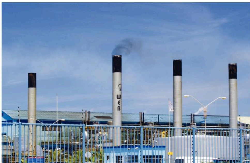
▲ Figure 17.2.5 Desalination plant at Aruba
