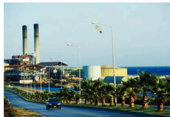
▲ Figure 14.4.4 Desalination plant
