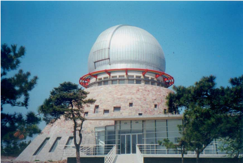
Fig. 1. The main building for the NEO telescope.
