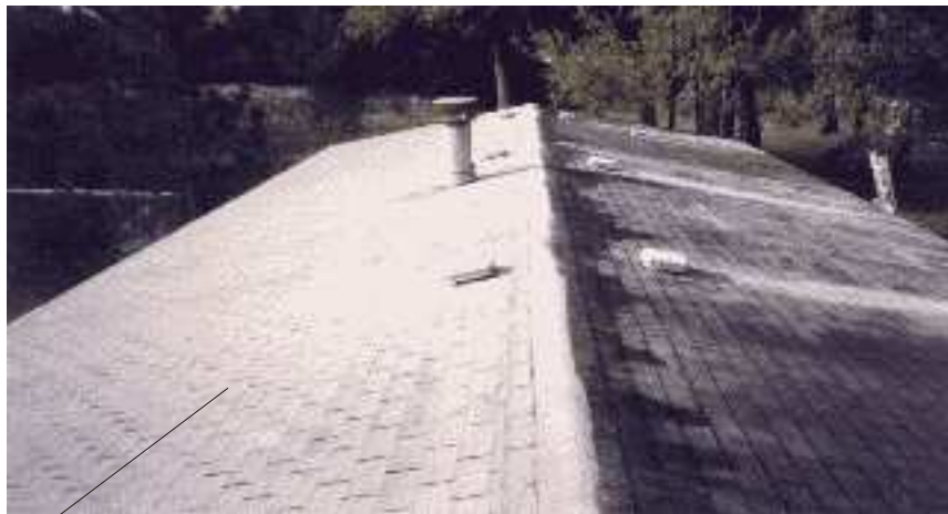
Side Not cleaned, Infected with Mold
