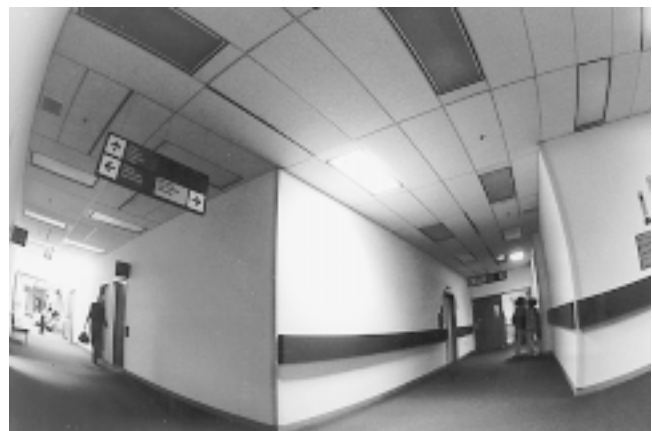
Fig. 1 Stupid delamping Some of these hospital corridors are much brighter than necessary, while others have long unlighted areas. Nobody planned this work, and nobody checked it.
