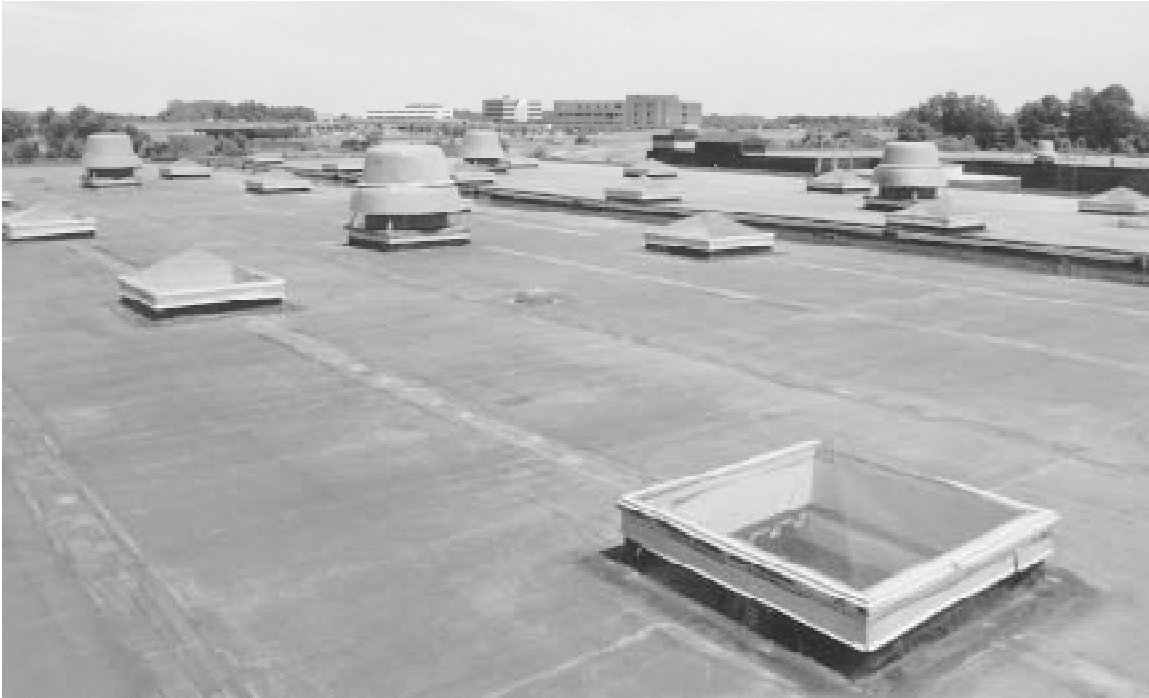
Fig. 6 Good skylight sizing and layout This shows the small fraction of roof area that is needed for typical illumination levels. These skylights are for a gymnasium, and the repetitive layout provides uniform illumination within the space. See Figure 1 of Measure 8.3.2 for the inside.
