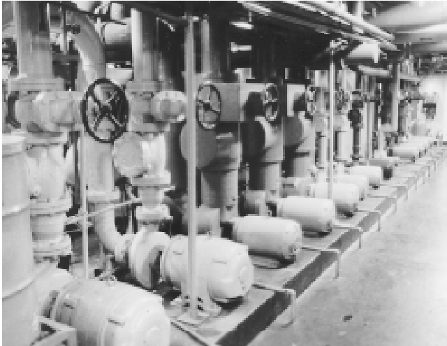
Fig. 1 Pump row of a large hotel All these pumps are in duplicate sets. Only one of each needs to be running. A transfer switch for each pair is a cheap, foolproof way to avoid unnecessary operation.
