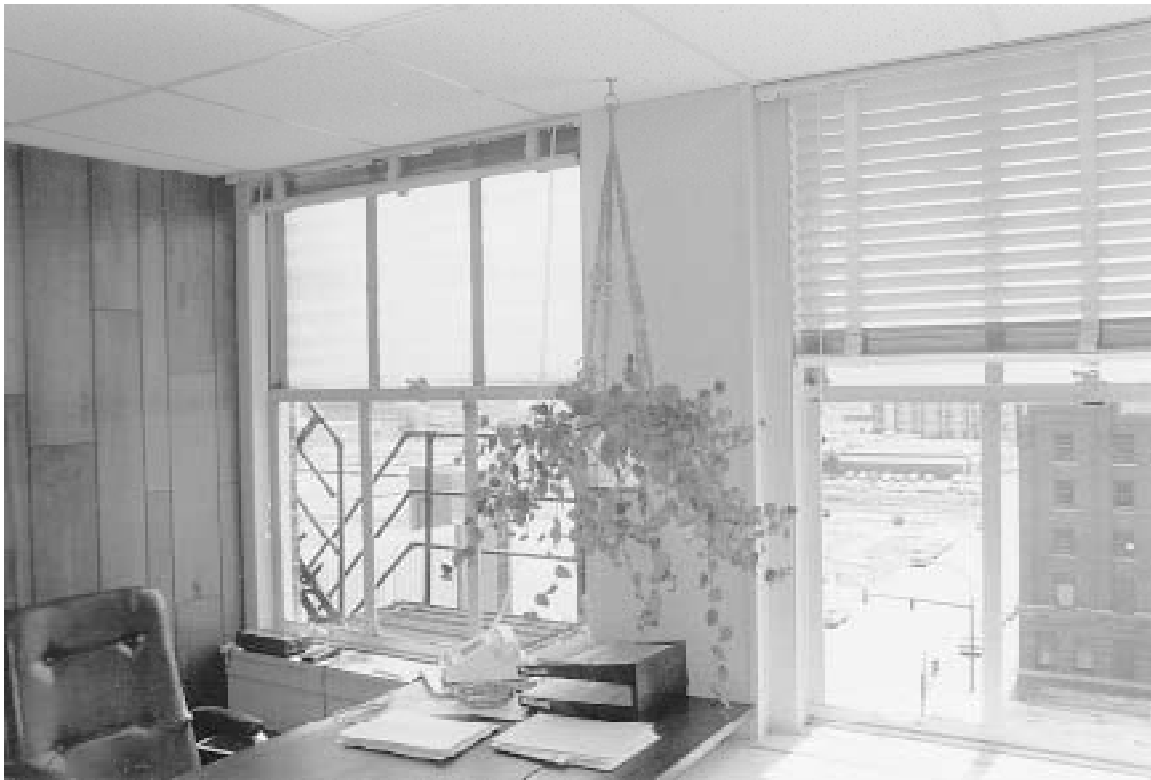
Fig. 2 A lesson from the real world about window diffusion The orientation of activities with respect to the windows is a crucial factor in using window diffusers. In this office, the upper panes of the double-hung windows are made of diffusing glass. The diffuser to the side of the chair provides good illumination for the desk. However, the diffuser in front of the desk causes glare, so it has been covered with a venetian blind.
