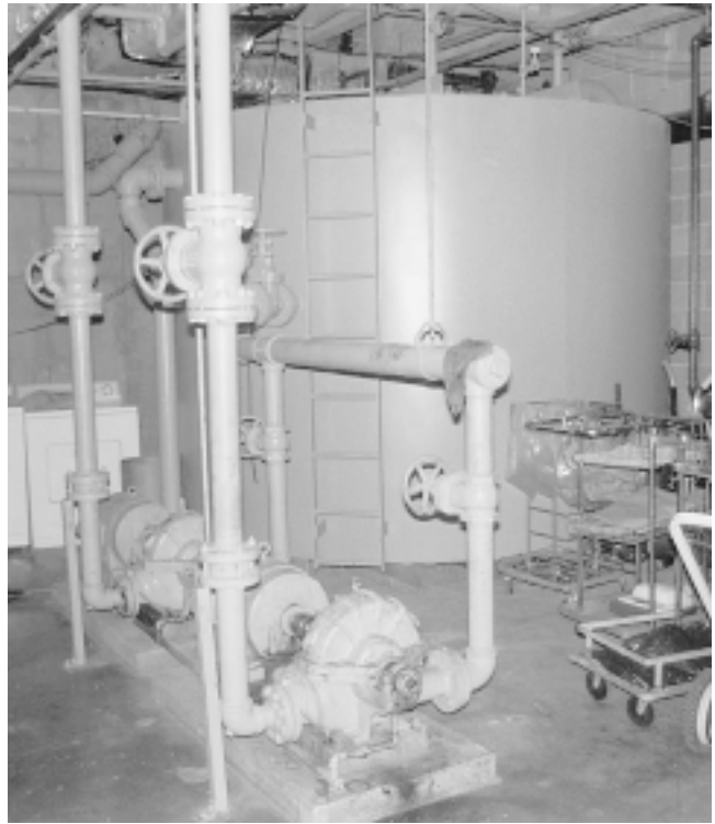
Fig. 4 Failing to exploit city water pressure In this large hotel, city water is delivered to the vented tank in the background. All the city pressure is lost. The large pumps in the foreground must operate continuously to provide pressure within the building.
