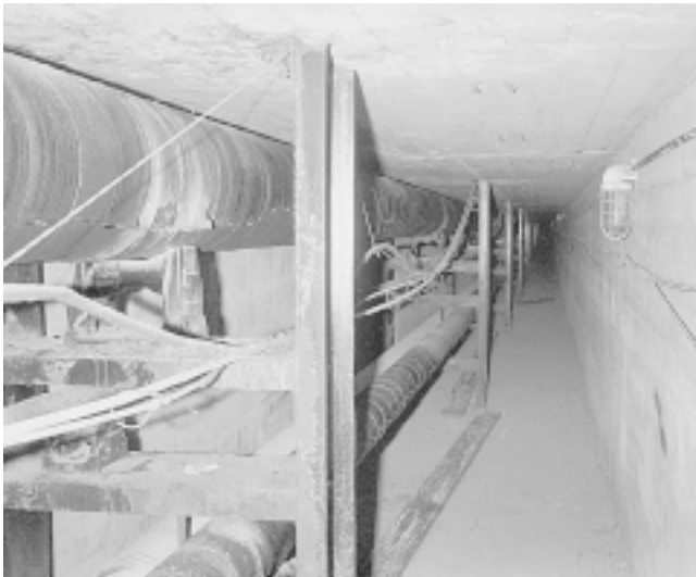
Fig. 2 An ideal environment for heating system insulation If the pipe is warm, the insulation will remain dry regardless of the humidity in the tunnel. However, this is a challenging environment for chilled water pipe insulation, especially if hot and cold pipe run in the same tunnel.
