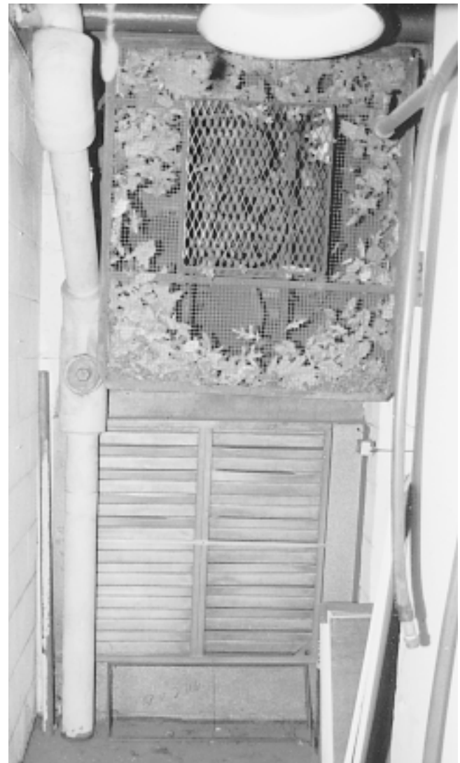
Fig. 2 A collection of combustion air problems This air intake for a small boiler is very large. However, it has an intake fan that upsets the air-fuel ratio of the atmospheric burner. The bottom louvers of the intake have been closed, and the top is being clogged by leaves.
