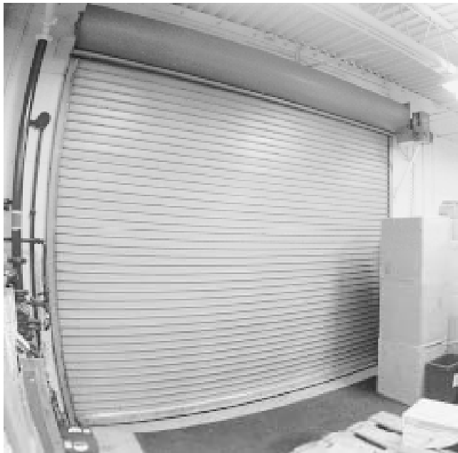
Fig. 3 Roll-up door The main virtue of this type of door is compactness. It can be motorized easily. The large number of segments make it impossible to insulate well. Some models seal against infiltration fairly well, and some do not.
