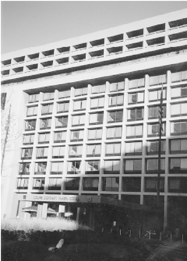
Fig. 1 Why it is tricky to sense cooling load Some spaces on this face of the building are in deep shade, while the rest are exposed to strong solar gain. To turn off the chillers that cool this zone, sensors must be located where they will detect a cooling load in any part of the zone.
