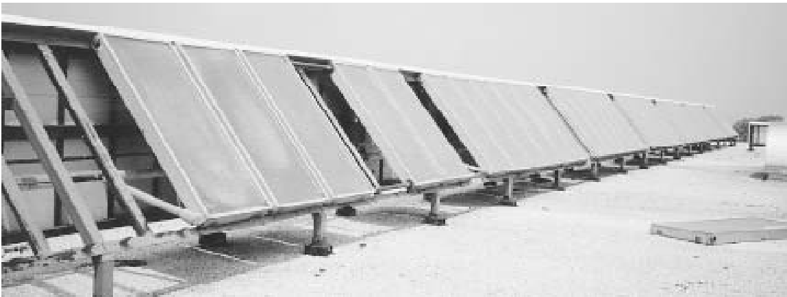
Fig. 1 An array of flat-plate solar collectors This installation shows typical dimensions and mounting of flat-plate collectors. Sadly, it also illustrates the poor design and maintenance that is given to this basically simple technology. Individual collectors had to be removed because no access was provided for maintenance of the connecting joints. These are subject to rapid wear because of the large thermal expansion coefficient of aluminum and the large temperature cycles in daily operation. The system was eventually abandoned because of avoidable freeze damage.
