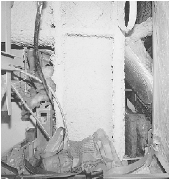
Fig. 2 Air leakage superhighway This is the scene behind the opaque portions of the curtain wall of a new glass box office building. The insulation was joined by tape. The tape quickly fails, causing the insulation to collapse. Air cooled by the exterior surface of the curtain wall freely circulates to the interior of the building, rendering the insulation useless. Shoddy practice like this is common in glass box buildings.
