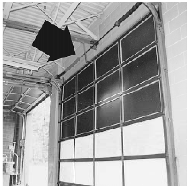
Fig. 1 Common door operator problem The arrow points to the link between the door operator and the top of the door. When the door starts to open, the link pulls horizontally, whereas the door can only move vertically. This creates a strong bending force on the center of the top panel. You can avoid this problem while using the same operator by using two long links between the operator and the sides of the door.
