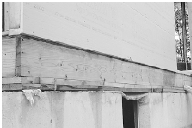
Fig. 4 Foundation plate, from outside A layer of insulation material is used to seal the gap between the concrete wall and the rim joist. Although sold commercially for the purpose, this is the wrong type of material for the job.
