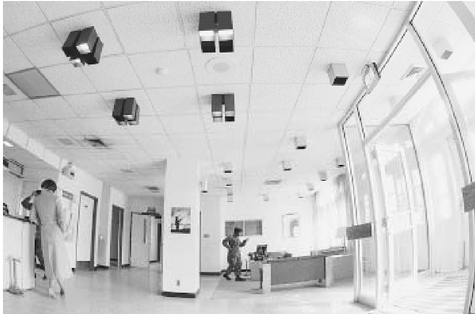
Fig. 3 Downlight abuse in a military barracks Downlights are utterly inappropriate for this environment. At least the floors are polished, so some light gets into the space. These fixtures are so ineffectual that nobody notices that many of the bulbs are burned out. The remaining ones are just wasting energy, because the glass front is providing plenty of daylight. A few fluorescent fixtures and some basic controls would illuminate this space for less than ten percent of the present cost.
