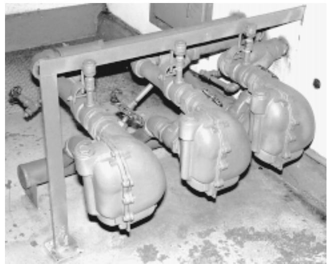
Fig. 3 Typical F&T traps The chubby shape provides space for the float ball to swing up and down. The thermostatic element is on the upper left.
