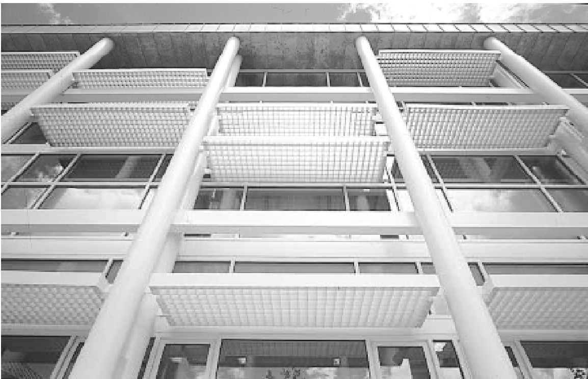
Fig. 9 Egg crate louvers The egg crates block sunlight from all directions. They are supported by the columns, rather than being attached to the wall. This rather massive construction and the irregular placement of the louvers may have been motivated by an appearance concept as much as by sunlight control.
