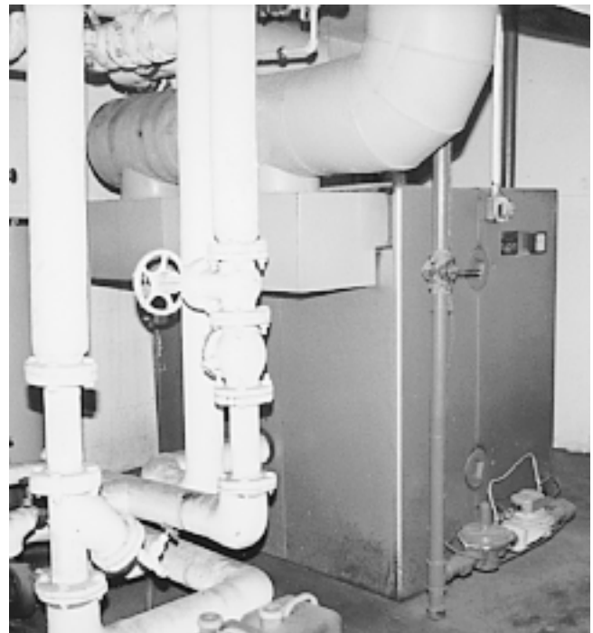
Fig. 1 A flue damper installation challenge This boiler has atmospheric burners, several flue gas outlets, and an integral draft hood. Installing a flue damper here would require a lot of sheetmetal work.
