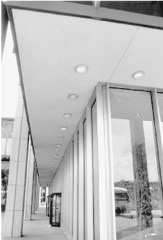
Fig. 1 Lights turned on in the middle of the day These lights are turned on because the switch is installed at some remote location where the lamps cannot be seen. Photocontrol is the most reliable and least expensive control method for this situation.
