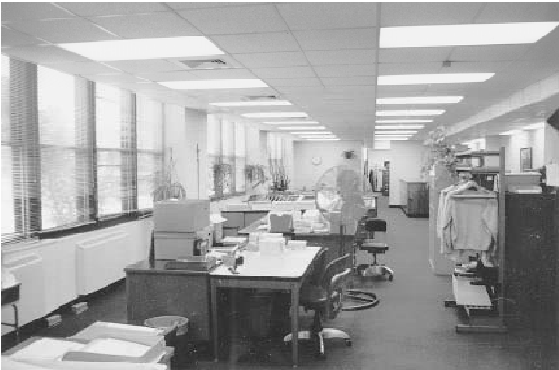
Fig. 2 Easy savings This government office has a high level of illumination for a few desks and work tables, some filing cabinets, and a lot of empty space. Perhaps 80% of the energy cost of lighting this space could be eliminated with easy changes. Most of the fixtures could be eliminated or delamped. Adding some inexpensive controls would adapt the space to occupancy and exploit the ample daylighting that is available. Task lighting would further reduce the remaining energy consumption.
