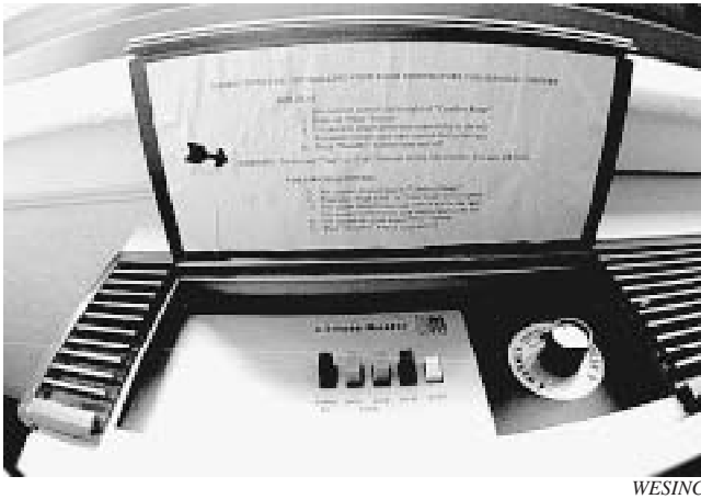
Fig. 1 Hotel room conditioning unit placard These instructions are located in the right place, but they are difficult to read.
