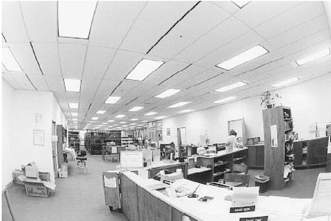
Fig. 4 Task lighting challenge No. 3 This credit union office has fluorescent lighting in a tall ceiling, which is illuminating nothing at this moment. There are a few desks and work tables, some shelves, and a counter for the public. The arrangement of the space, and even its basic use, will probably keep changing. How would you provide efficient and pleasing lighting for all the activities, now and in the future?
