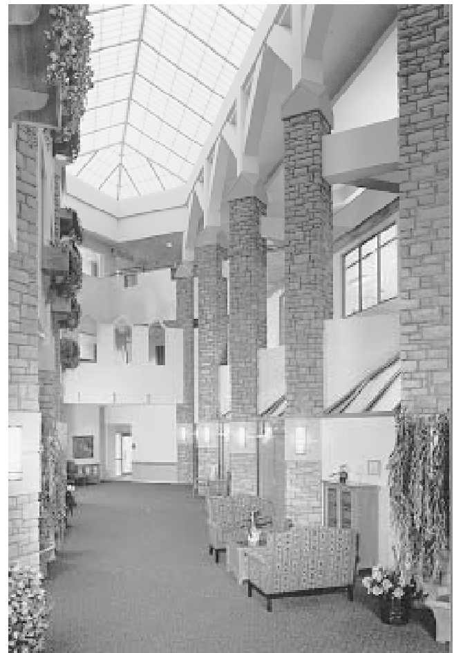
Fig. 7 Translucent roof with relatively low glare potential The translucent roof provides daylighting for several levels. Glare is a major issue in this building because the occupants are elderly. The potential for trouble is minimized by the elevation of the translucent surface well above the line of sight and by the nature of the activities, which allow the occupants to choose their direction of gaze.
