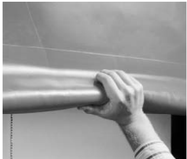
Fig. 6 Yielding edge This model of roll-up door uses a lower edge that is filled with gravel. The gravel also provides weight for closing the door by gravity. A common alternative is a “reversing edge,” which has a contact switch that causes the motor to open the door. Some doors have a lower edge made in segments, with links that yield when the edge is struck.
