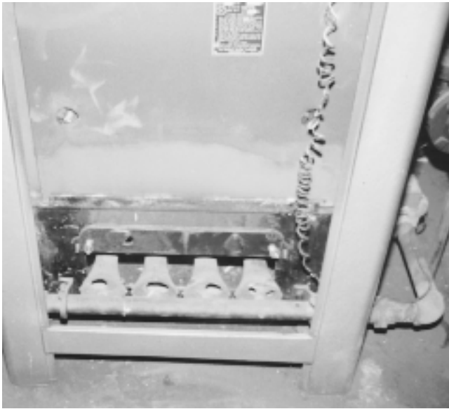
Fig. 1 Atmospheric gas burner The primary air to each venturi is adjusted on this furnace by rotating a plate with holes in it. As you can see, the settings are random, wasting energy and increasing air pollution.
