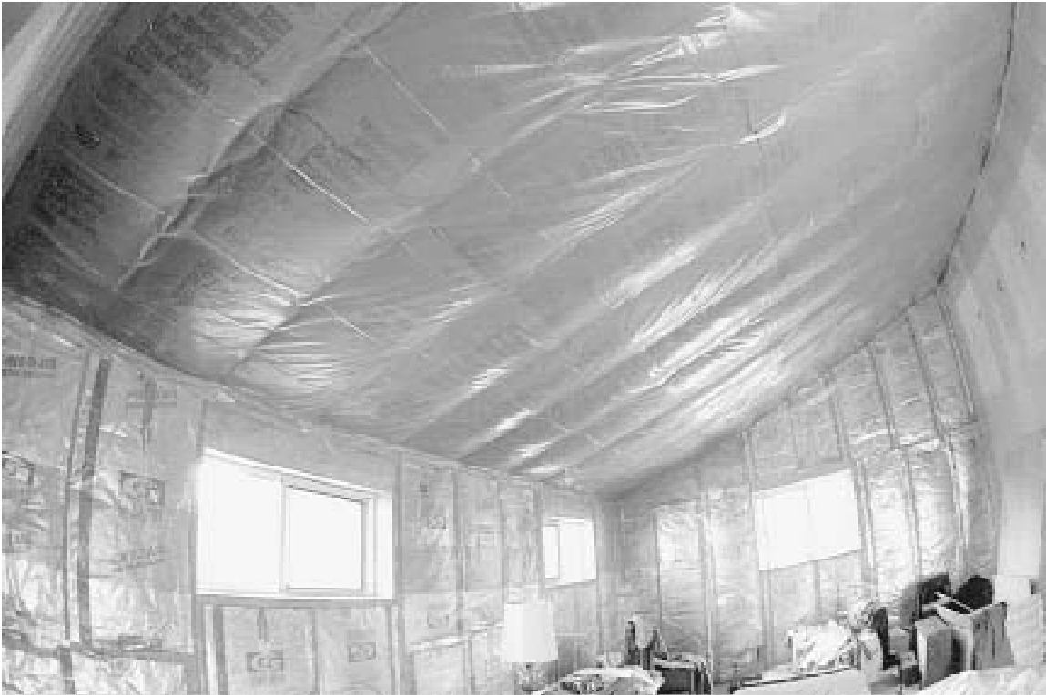
Fig. 2 Perfectly installed insulation and vapor barrier This large room has wood stud walls and a wood rafter cathedral ceiling. Glass fiber batt insulation has been inserted snugly into the stud and rafter spaces, leaving no gaps. The tabs on the paper backing of the insulation are overlapped and closely stapled to the edges of the studs and rafters. A vapor barrier of 0.008" thick polyethylene sheet is stapled over the insulation. The vapor barrier is overlapped several feet at all joints. Plenty of excess plastic material is left in all corners. This slack keeps the plastic from being torn when the wallboard is installed. The vapor barrier is stapled to the window frames, preventing air leakage around the windows.
