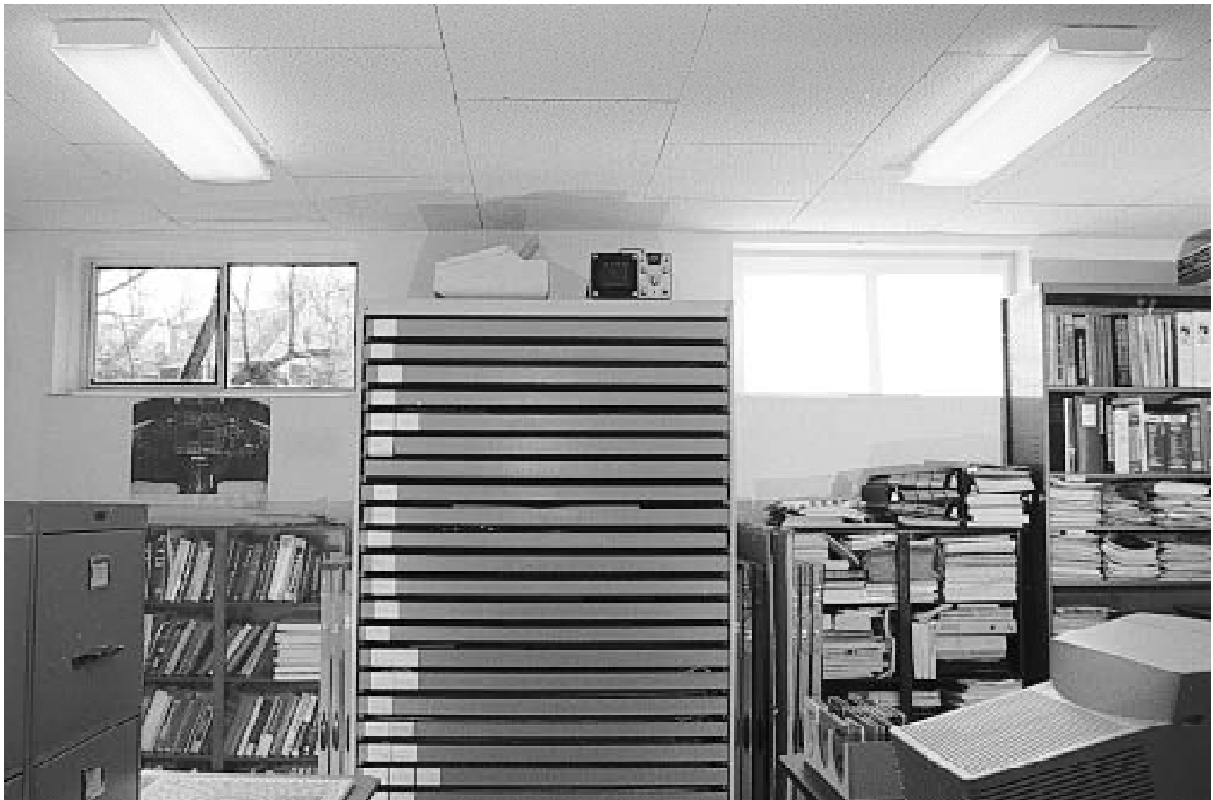
Fig. 1 How window diffusers behave In this demonstration, sunlight is shining on two clear windows of an office. A milky white plastic diffuser is installed inside the window at right. The light fixtures are turned on for comparison. The diffuser causes a considerable amount of glare, the intensity of which cannot be conveyed by the photograph. In contrast, the scene outside the clear window is not bright enough to create glare. From this point of view, the surface of the diffuser appears considerably brighter than the surfaces of the fluorescent light fixtures. Notice the amount of light scattered by the diffuser on the ceiling. This aids daylight penetration. The ceiling should be highly reflective to exploit this.
