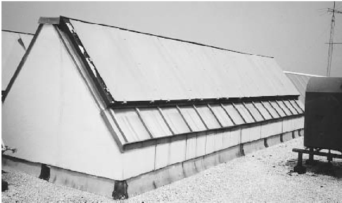
Fig. 4 Skylights are not the same as daylighting Just making glazed holes in the roof does not create satisfactory daylighting, as this abandoned and covered skylight on a classroom building testifies. The problem was excessive glare.
