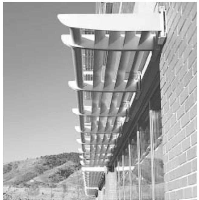
Fig. 14 Shading louvers attached to wall by brackets
