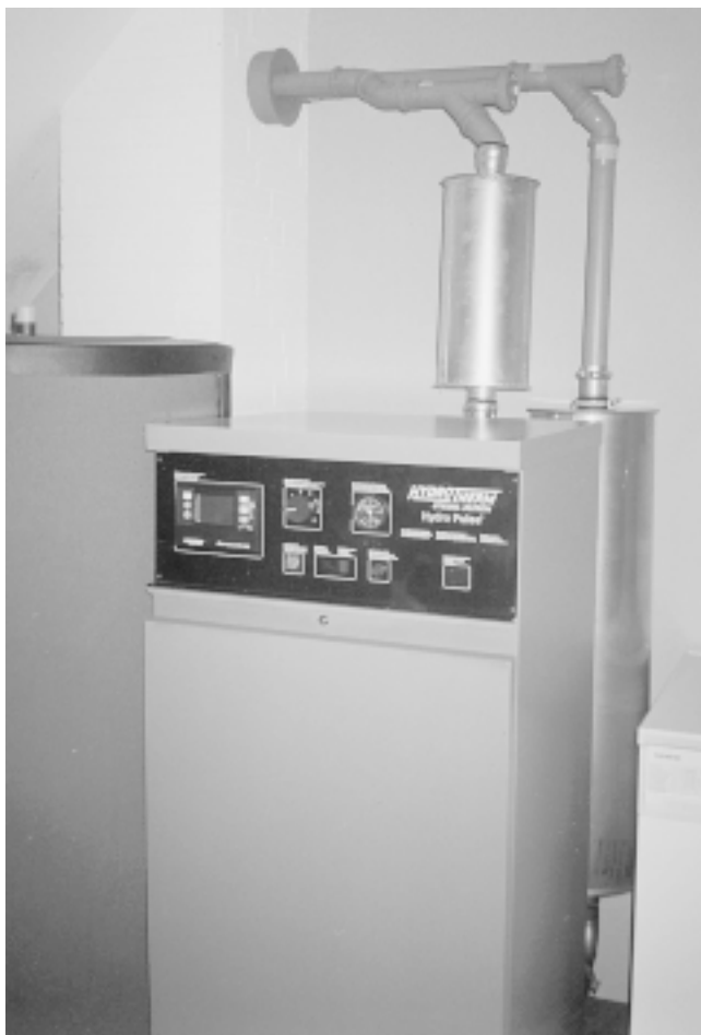
Fig. 2 High-efficiency water heater The exhaust is so cool that plastic pipe is used for the flue. This model uses pulsed combustion, an unusual feature of one manufacturer. The small muffler in the combustion air intake pipe and the very large muffler in the exhaust pipe minimize the noise.
