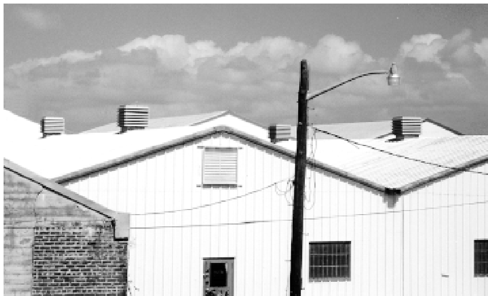
Fig. 1 Reflective paint provides most of the cooling of these buildings These buildings have metal roofs and walls, which makes it important to paint them with a fairly heavy coat of non-conducting paint. These buildings, located in a sunny climate, have good exhaust stacks, but they are too far apart. Continuous ridge vents would be better. The ventilation inlet louver on the end of the gable lacks sufficient open area.
