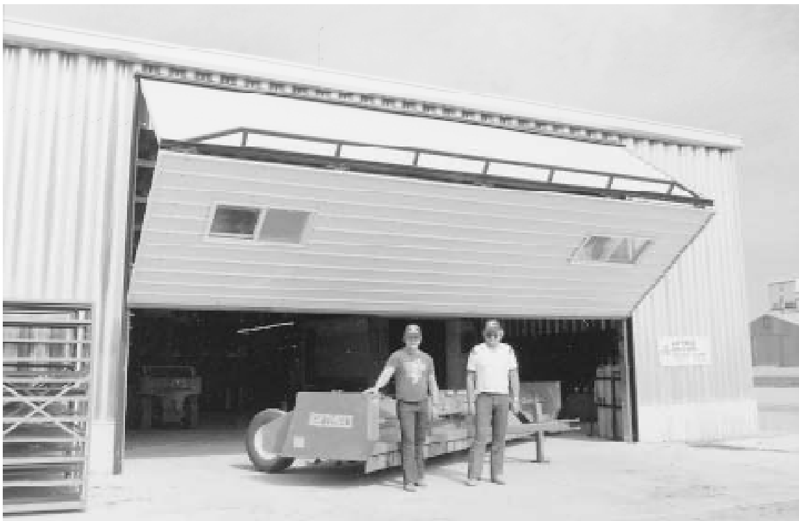
Fig. 2 Bi-fold door Almost all vertically opening panel doors consist of two panels, as shown here. A truss is needed at the bottom edge to resist bending from the weight of the panel. This model also has a truss at the center, which protects against wind loads when the door is closed. It is easy to install windows or a person door in the panels.
