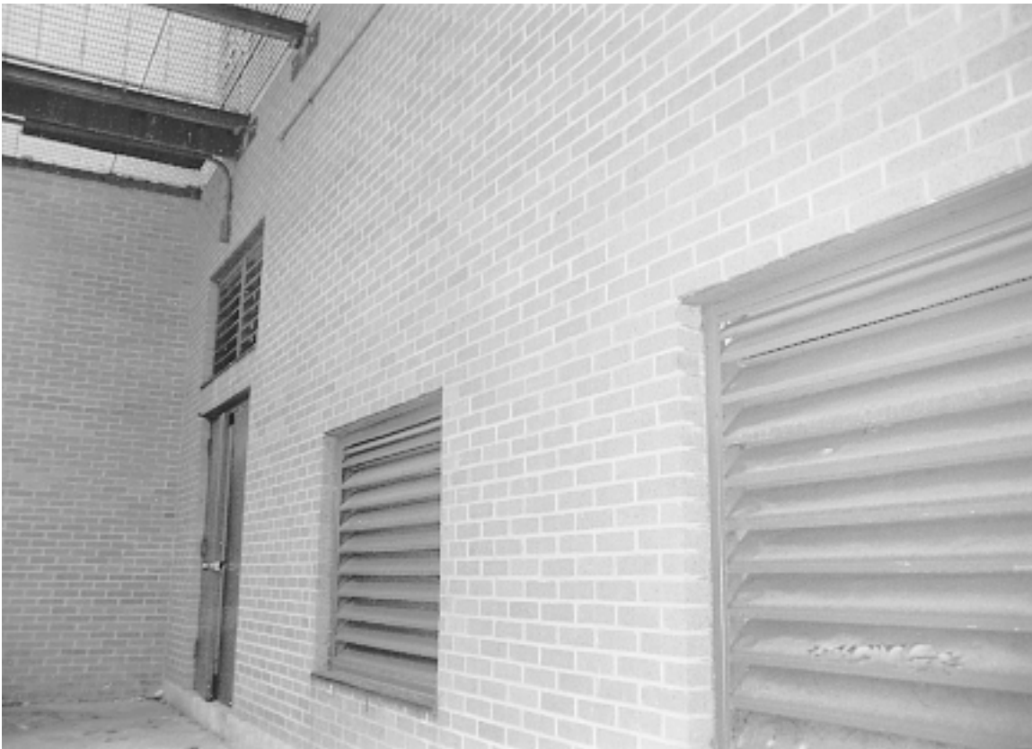
Fig. 1 Outside air intakes below grade Vehicle exhaust fumes from the adjacent street readily enter here, along with grass clippings, lawn chemicals, etc. Note the leaves accumulated behind the louver at right. On the positive side, easy access to the pit makes it easy to clean out. The large area keeps the entering air velocity low, which minimizes the tendency to pick up debris. Still, it would be better to install these intakes on the roof.
