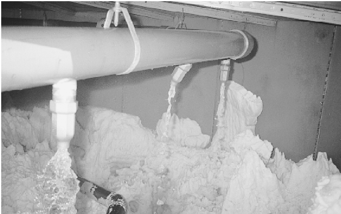
Fig. 18 Separated slurry system ice storage tank The returning chilled water is sprayed into the ice tank for cooling. The irregularity of the ice pile suggests that water distribution is less than ideal.
