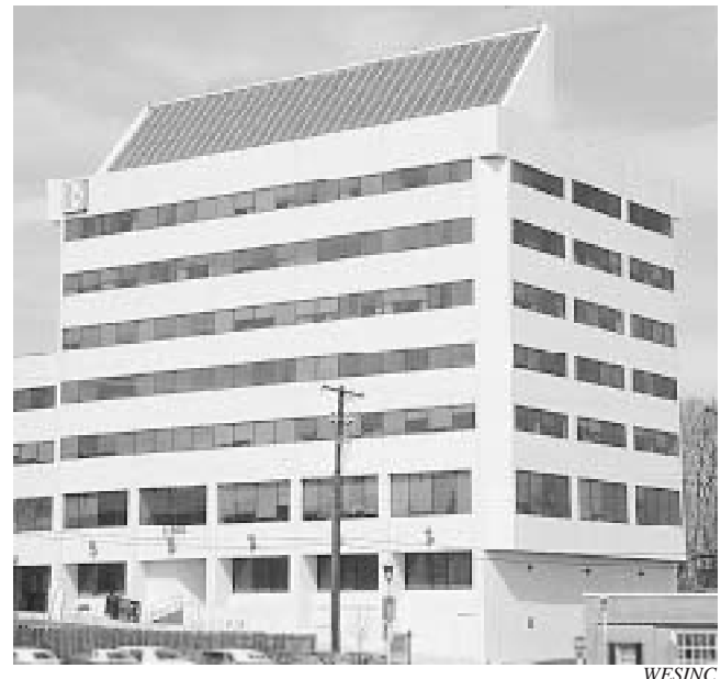
Fig. 4 Typical space heating and domestic water heating application for solar energy This array is nicely integrated into the architecture of the building. It even faces in the correct direction, unlike many solar installations.
