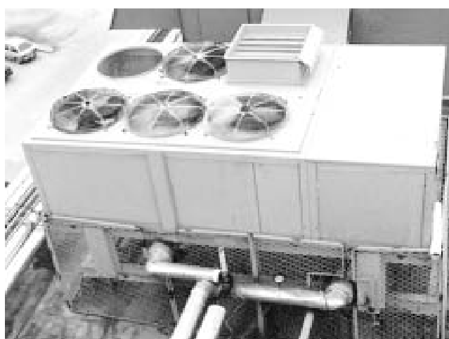
Fig. 3 What is wrong with this condensing unit? A fan failed and was never replaced. This allows air to enter through the hole and bypass the condenser coils. Efficiency and capacity are suffering seriously. A thermostatically controlled damper is installed to maintain a minimum condensing temperature. It will create the same problems if it is not working properly, or if the damper blades do not close fully.
