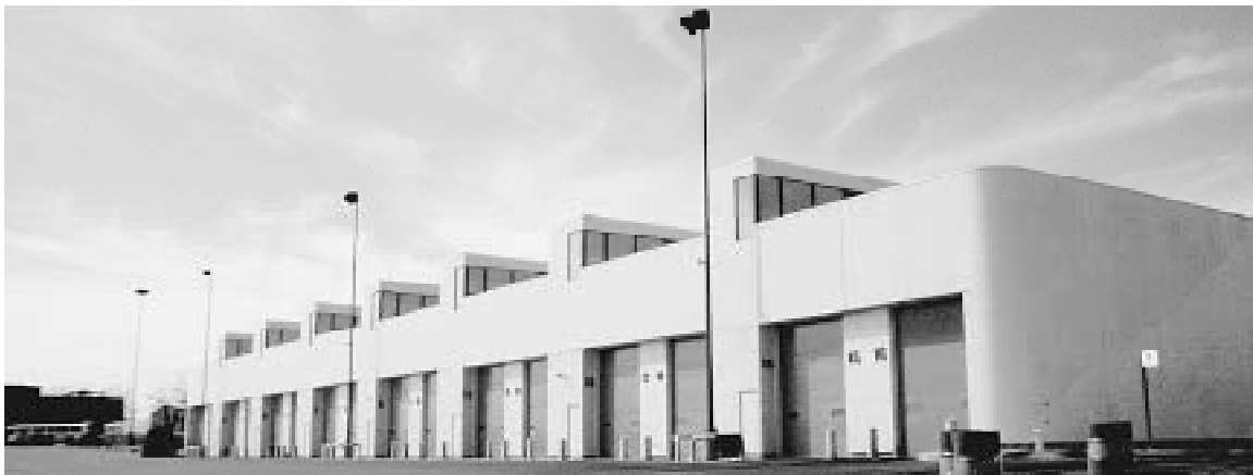
Fig. 5 Inefficient skylight orientation The skylights on this bus garage face north. This avoids glare problems and excessive solar heat gain, but it provides little light in relation to the heat loss from the glazing. Overhead equipment keeps much of the daylight from penetrating into the space.
