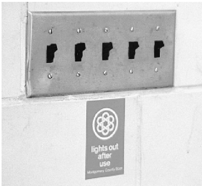
Fig. 3 Useless placard This sticker tells us to turn off the lights. So, now what? These switches are in an obscure location. Which spaces do they control? Which fixtures does each switch control? How do we know if there are other people still in the space?
