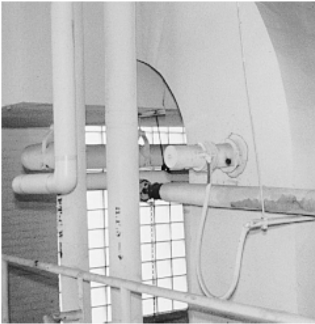
Fig. 1 Smoke opacity monitor This is simply a bright lamp that shines across the flue toward a light sensor on the other side.
