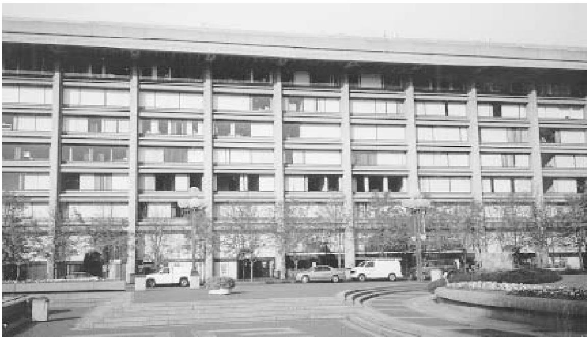
Fig. 5 Windows are not the same as daylighting If direct sunlight can enter a space at any time, the occupants will shut out sunlight entirely, as we see here. The situation is not helped by the vertical blinds, which are an unsatisfactory method of modulating sunlight. There is a nice view, but the occupants can't enjoy it, except on the top floor, which is shaded by a deep overhang. This vast amount of glazing serves little useful purpose, and it increases heating and cooling costs considerably.
