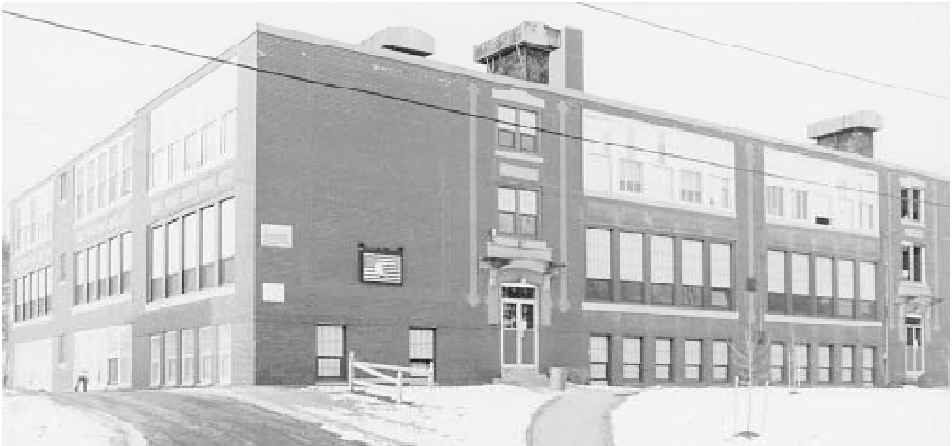
Fig. 4 The exterior of Figure 3 . The windows on the first and second floors have been retrofitted. The windows on the third floor remain. The appearance is changed from aged to slightly industrial.
