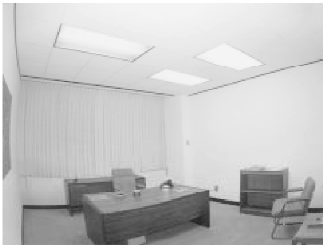
Fig. 1 One desk does not need twelve fluorescent lamps This small office has three 4-lamp fixtures. The right front fixture creates serious veiling reflections at the desk. The right rear fixture cannot illuminate the desk properly because it is behind the viewer’s body. Both could be eliminated. The fixture on the left will provide ample illumination. The office has a large window, which could provide daylighting. This would require reorienting the desk and improving the window treatment.
