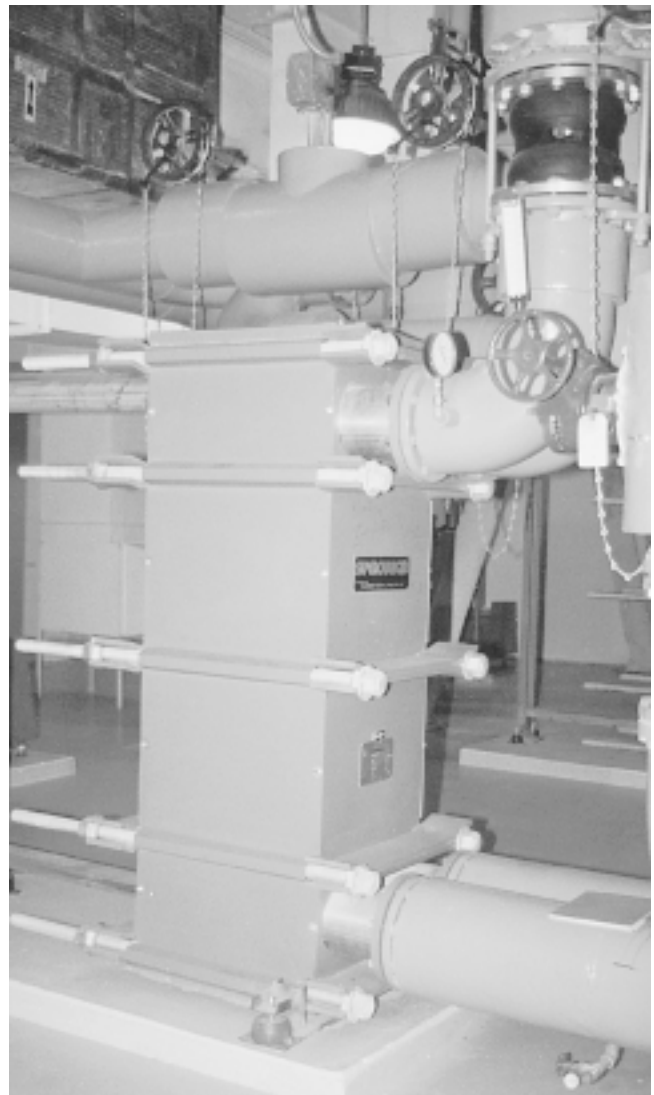
Fig. 3 Heat exchanger for waterside economizer system This plate heat exchanger is very compact, but expensive. It reduces the efficiency of both the waterside economizer and the DX cooling systems.
