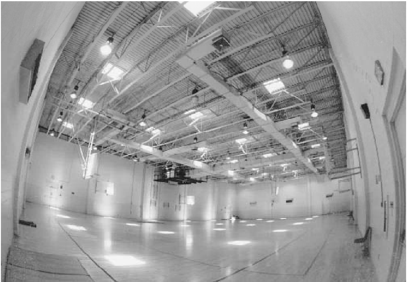
Fig. 1 Potentially good daylighting rendered useless by lack of diffusers The skylights for this gymnasium are clear. Therefore, direct sunlight creates bright spots on the polished floor which are blinding to players and spectators. Note their reflections on the walls and ceiling. Because this daylighting is useless, the electric lights are turned on. The fixtures here are HID. They require a long time to brighten, so they are left on, despite the fact that the gymnasium is usually vacant.
