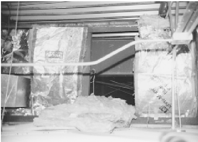
Fig. 5 Irresponsible insulation job This batt insulation in a big, new office building was simply suspended by the paper backing sheet, and adjacent batts were taped together. The batt in the middle has fallen down already, and the rest will follow within a few years.
