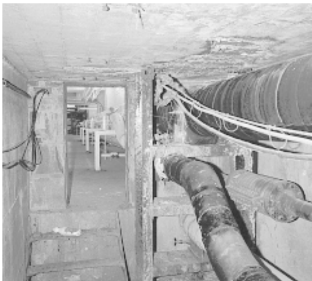
Fig. 1 Door to steam tunnel This steam tunnel opens into the lower level of a barracks. There would be less heat loss from the steam pipe, and the barracks would remain cooler, if the door were kept closed. All it takes is a sign.
