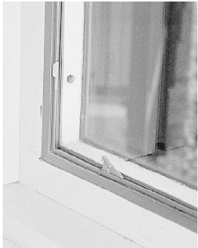
Fig. 2 Corner of window with interior removable glazing The inner pane is held in place by the clips. The hole at left vents the space between the panes to the outside. These windows were installed as part of the original construction. Nowadays, in new construction, you would select a sealed double-glazed window. However, this arrangement shows the features that are important when retrofitting interior supplemental glazing.
