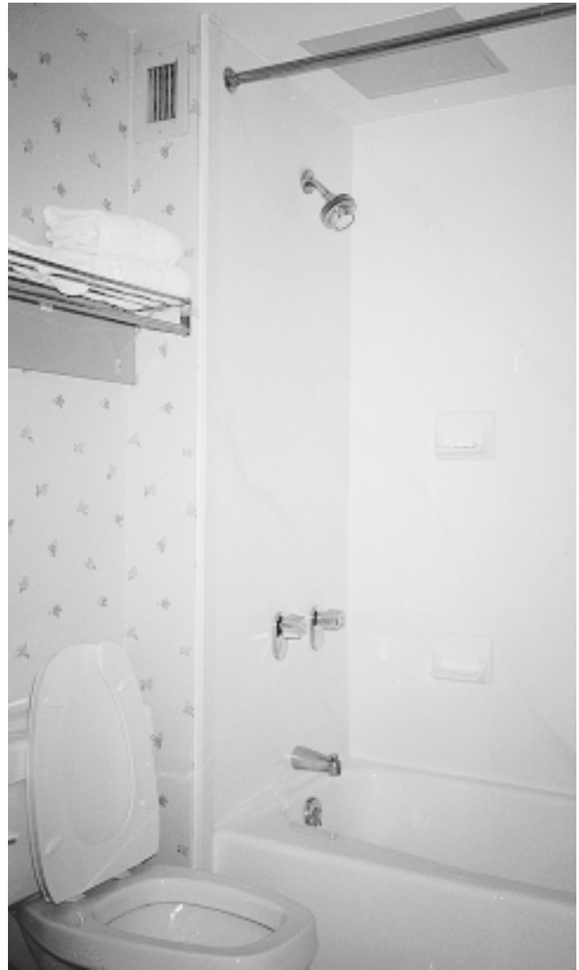
Fig. 1 Anyone can understand how to use these shower valves This conventional type is simplest, cheapest, easiest to maintain, easiest to use, and probably safest. Put a high-efficiency shower head in here, and this will be an ideal shower installation.
