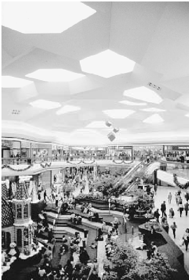
Fig. 1 Effective skylights in a shopping mall The percentage of ceiling area is about right for the type of illumination needed. Light distribution is good. The diffusing skylights are installed at the tops of tapered recesses, minimizing glare.
