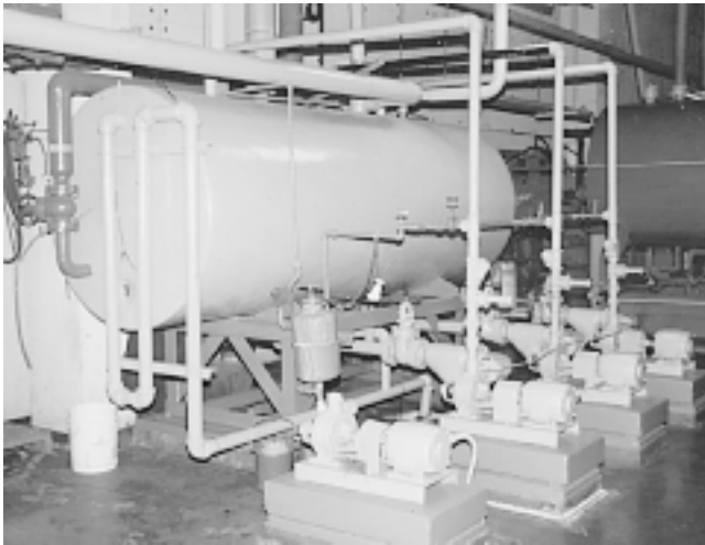
Fig. 5 Boiler water system for a large office building The tank is the main condensate receiver. The three pumps to the right are individual feedwater pumps for three boilers. The pump in front injects water treatment chemicals into the feedwater.
