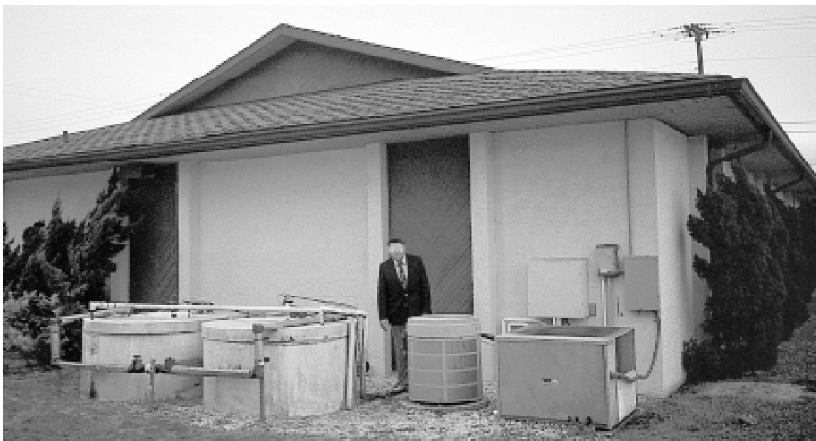
Fig. 11 External-melt cooling storage system using direct-expansion coils The partially buried, round tanks are filled with spiral copper evaporator tubing. The compressor and condenser units are on the right. This system serves a small professional building.
