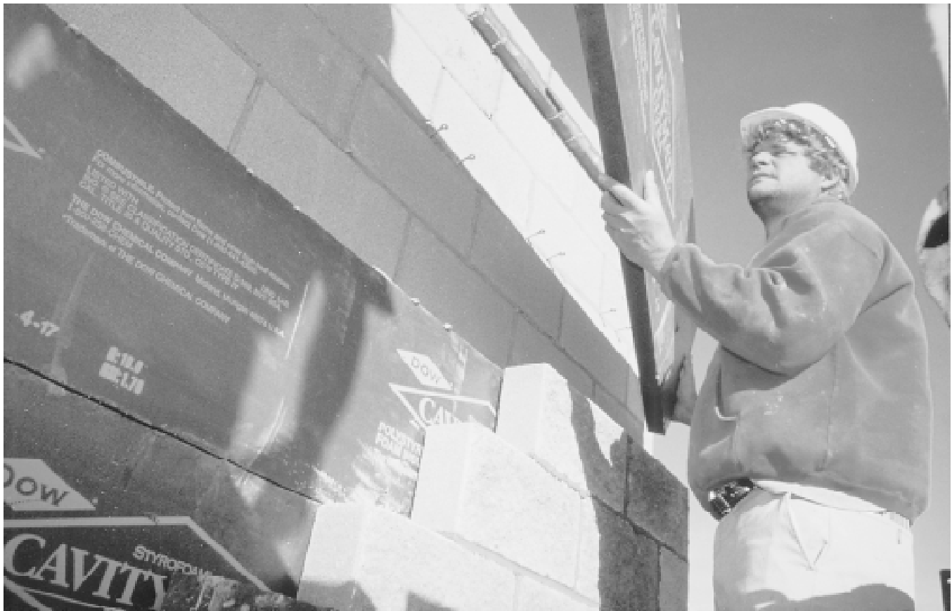
Fig. 2 Rigid board insulation inside a wall cavity Using rigid board insulation may be the most reliable way to install insulation inside a masonry wall. The big challenge with rigid insulation is avoiding convection paths between the boards, and between the boards and the wall. Note the eyes installed in the mortar joints for holding the boards snugly against the wall. This requires good workmanship.
