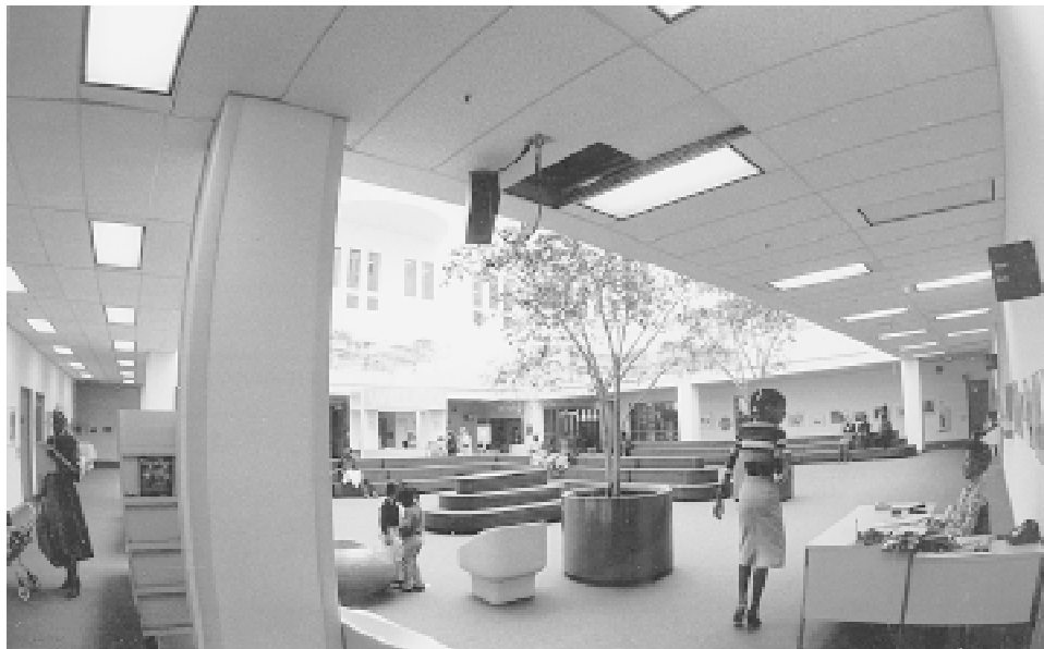
Fig. 4 Area surrounding a large, brightly lighted atrium This area deserves several photocontrols. The inner and outer rows of light fixtures should have separate control. And, each side of the atrium should have separate control.
