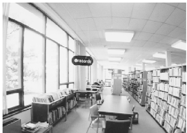
Fig. 2 Daylighted reading area in a library The row of light fixtures adjacent to the windows is a prime candidate for photocontrol.
