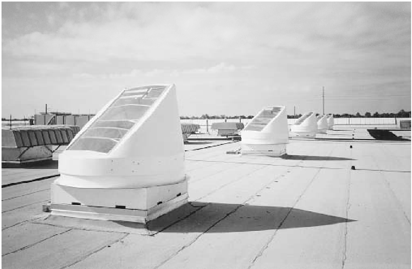
Fig. 14 Sun tracking light pipes The rotating head contains mirrors that reflect direct sunlight straight down the pipe, minimizing losses. However, sun trackers may be less effective than simple light pipes for collecting sunlight from a diffuse sky.
