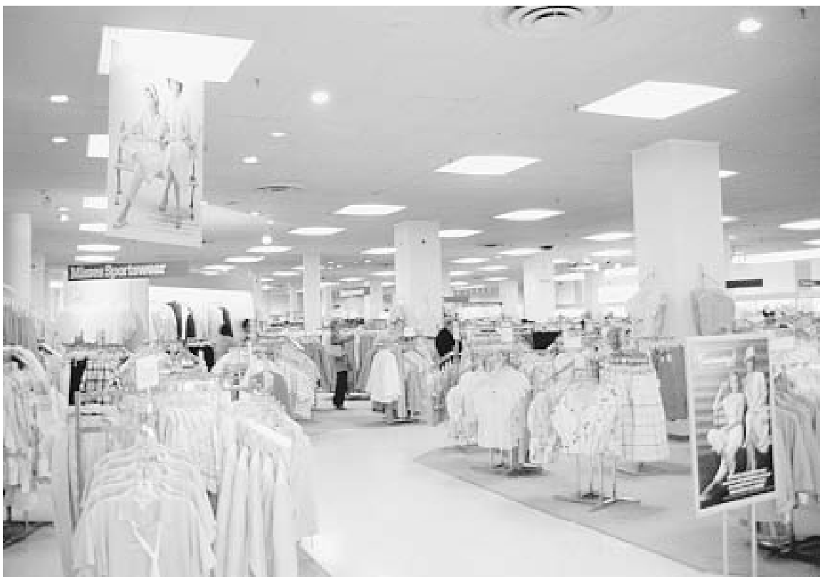
Fig. 5 Task lighting challenge No. 4 Lighting is a fundamental part of merchandising in this department store, and it is a major part of the store's operating cost. The present lighting is a combination of fluorescent fixtures and incandescent downlights located in a repetitive pattern, without regard to the location of the merchandise or the traffic flow. How would you save lighting energy here while improving the merchandising appeal of the lighting?
