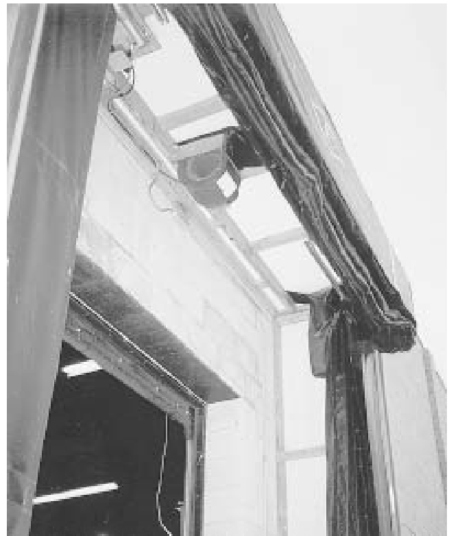
Fig. 4 Inflatable seal deflated The small fan at the top of the unit provides all the pressure that is needed for effective sealing.
