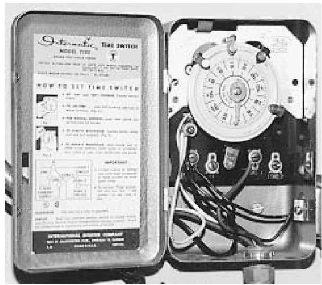
Fig. 1 Classic electro-mechanical timeclock This type is now obsolete for most applications. It is too inflexible, and it loses time with each power interruption. However, it was simple to understand and set. This unit has good instructions.
