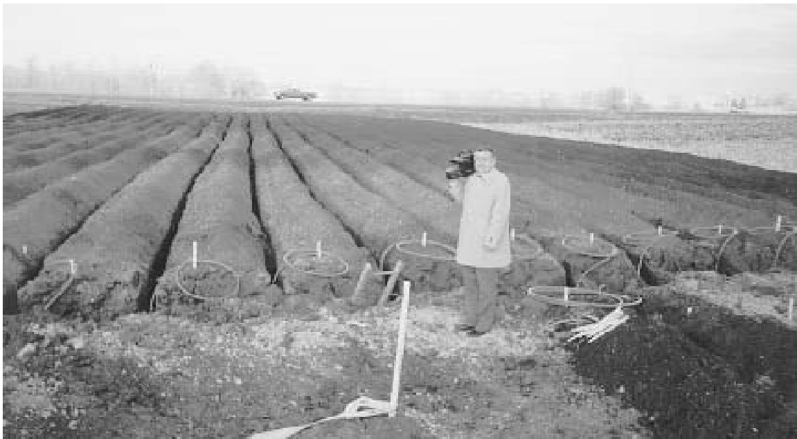
Fig. 1 Horizontal soil heat exchanger field This field is being installed to serve as the heat source and heat sink for a church in Minnesota. The climate here would not allow efficient operation of an air-source heat pump. Obviously, a large amount of open space is required. Loose soil makes it too expensive to bury the pipe at a depth that would provide the best efficiency.
