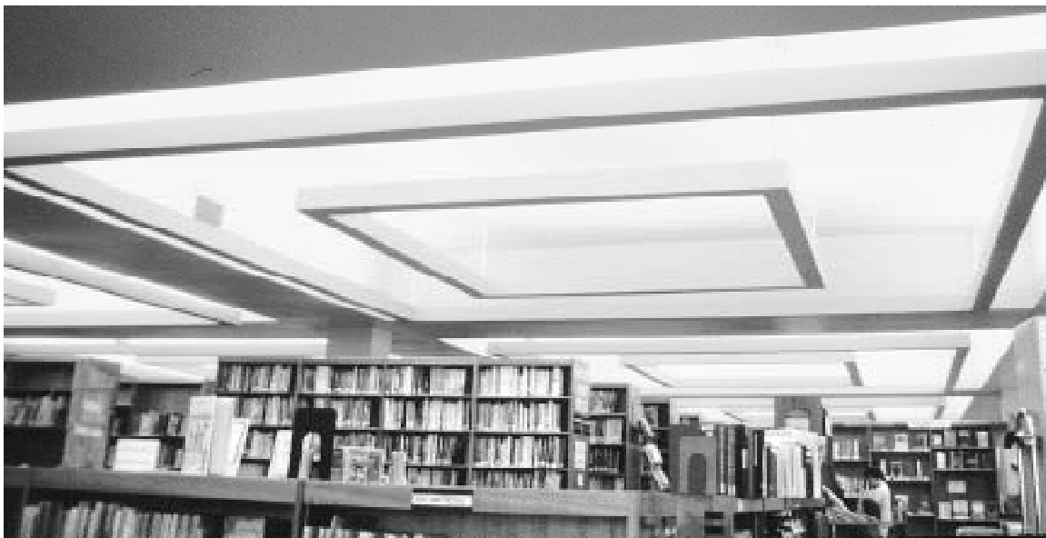
Fig. 1 Lighting power is highly dependent on surface colors here. Before light gets to any book in this library, it has to reflect from a ceiling surface at least once, and probably several times from ceiling, wall, floor and furniture surfaces. A slight reduction of surface reflectivity greatly reduces light loss.
