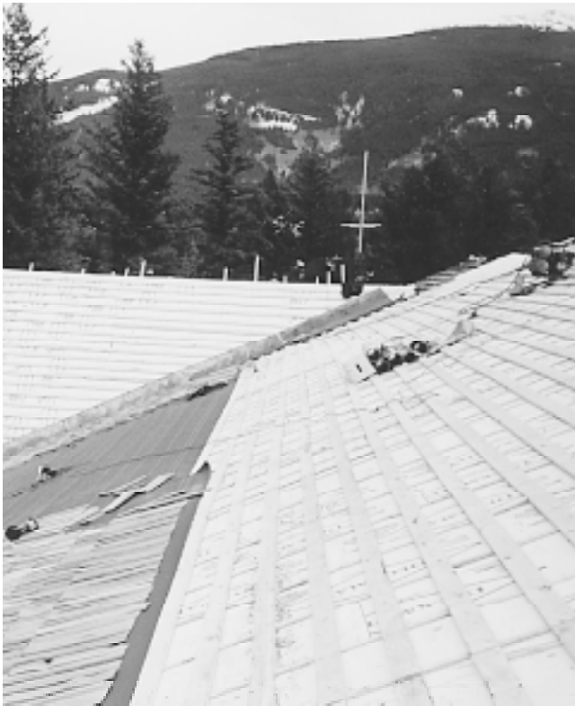
Fig. 2 Rigid insulation applied to a sloped roof Foam board insulation is applied under cedar shingles, allowing any desired amount of insulation value to be combined with a rustic appearance. With this common method of installation, any water that leaks through the shingles will be trapped by the horizontal battens, channeling the water between the joints of the insulation boards and through the nail holes into the underlayment.
