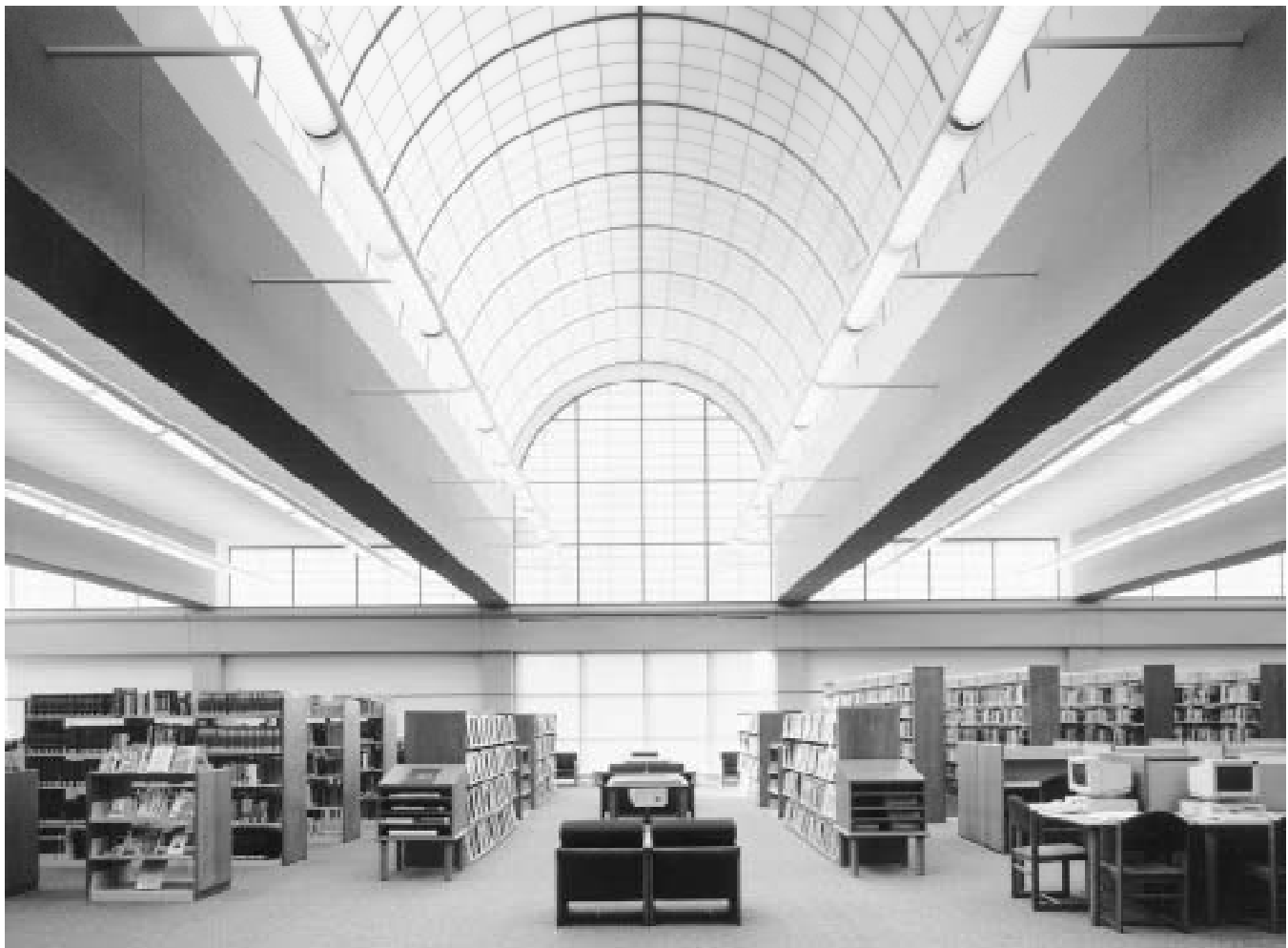
Fig. 2 Translucent panel construction for a library Reading is a particularly challenging application for daylighting. The translucent roof section provides effective illumination for a relatively narrow central area that is limited by the tall joists that run underneath it. The translucent wall sections require careful selection to avoid glare problems. We hope that the lights are normally turned off with this much daylight.
