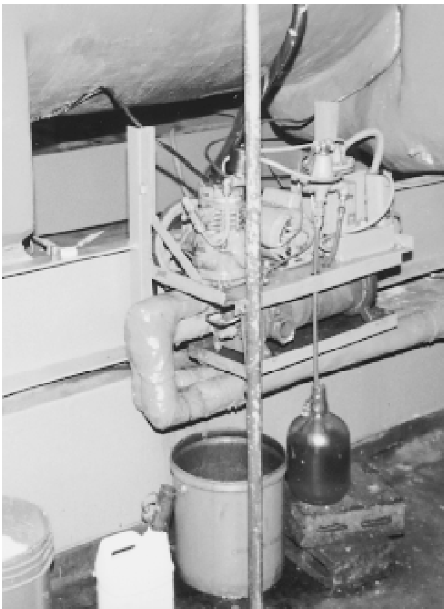
Fig. 1 Purge unit on chiller with low-pressure refrigerant This older purge unit discharges non-condensable gases through the jug of refrigerant oil on the floor. Bubbles in the oil show that air is leaking into the chiller. Refrigerant ejected by the purger dissolves in the oil, so it does not form bubbles.
