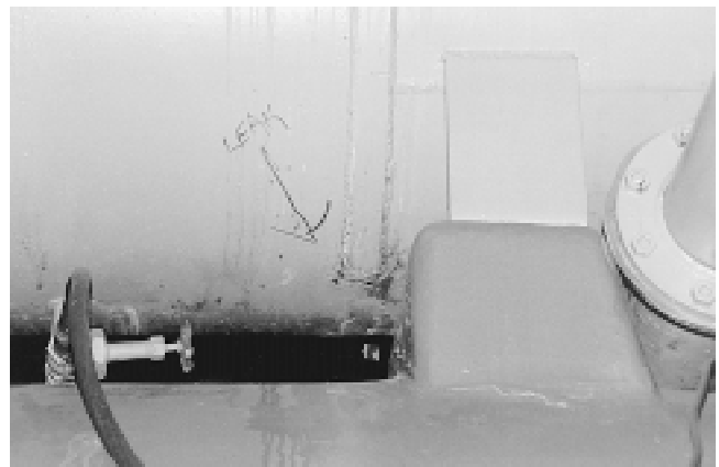
Fig. 2 Leakage at an original weld of an old chiller
