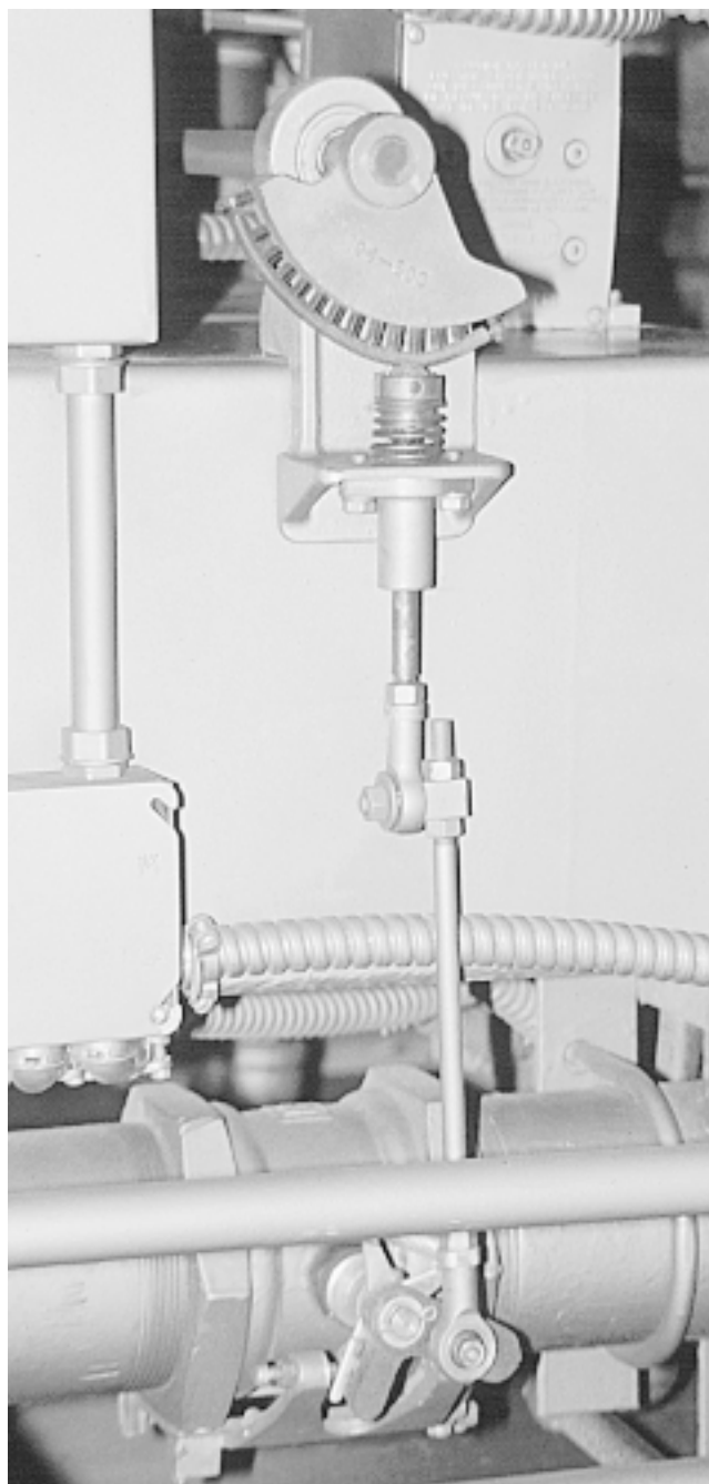
Fig. 4 Typical cam on jackshaft air-fuel linkage The shape of the cam determines the air-fuel ratio at all boiler loads. The shape can be adjusted by turning the screws that you see between the cam body and the curved spring that rides on the plunger. This is a tedious job.
