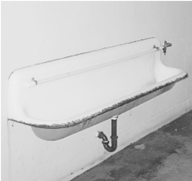
Fig. 4 Old communal urinal that flushes continuously This is a serious water waster. A valve actuated by a personnel sensor should be installed in the water line.
