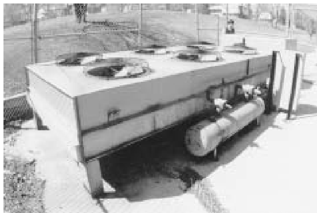
Fig. 2 Air-cooled condensing unit This unit serves a medium size public library. Being low to the ground makes it vulnerable to debris. It should be inspected from underneath and from above. The concrete slab and the surrounding fence help to keep it clean.
