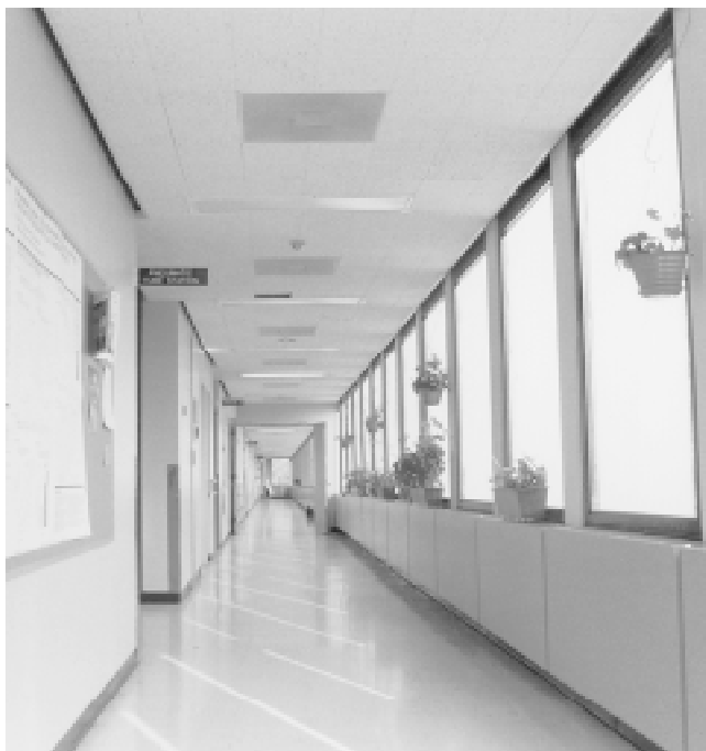
Fig. 1 Daylighted corridor This is an ideal application for photocontrol of lighting. Daylight provides ample illumination under most daytime conditions. The light fixtures are fluorescent, with multiple lamps, so they can even be switched in stages for a more gradual response.
