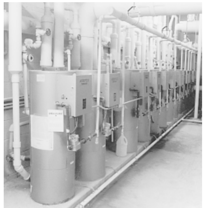
Fig. 1 A battery of condensing boilers for a large library Each boiler operates at a fixed output that optimizes its efficiency. Flue gas condensation provides high individual efficiency. Small increments of size adapt efficiently to all load conditions. The low flue gas exit temperature allows flues to be made of plastic pipe and to exhaust from an adjacent side wall.
