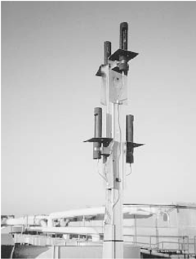
Fig. 3 Zone cooling load sensors Each sensor simulates the combined load from outside air temperature and solar radiation. The four sensors are oriented to determine the load for each face of an office building. These provide only an approximation. A sensor located at one point cannot simulate the load at each point on the face of a building.
