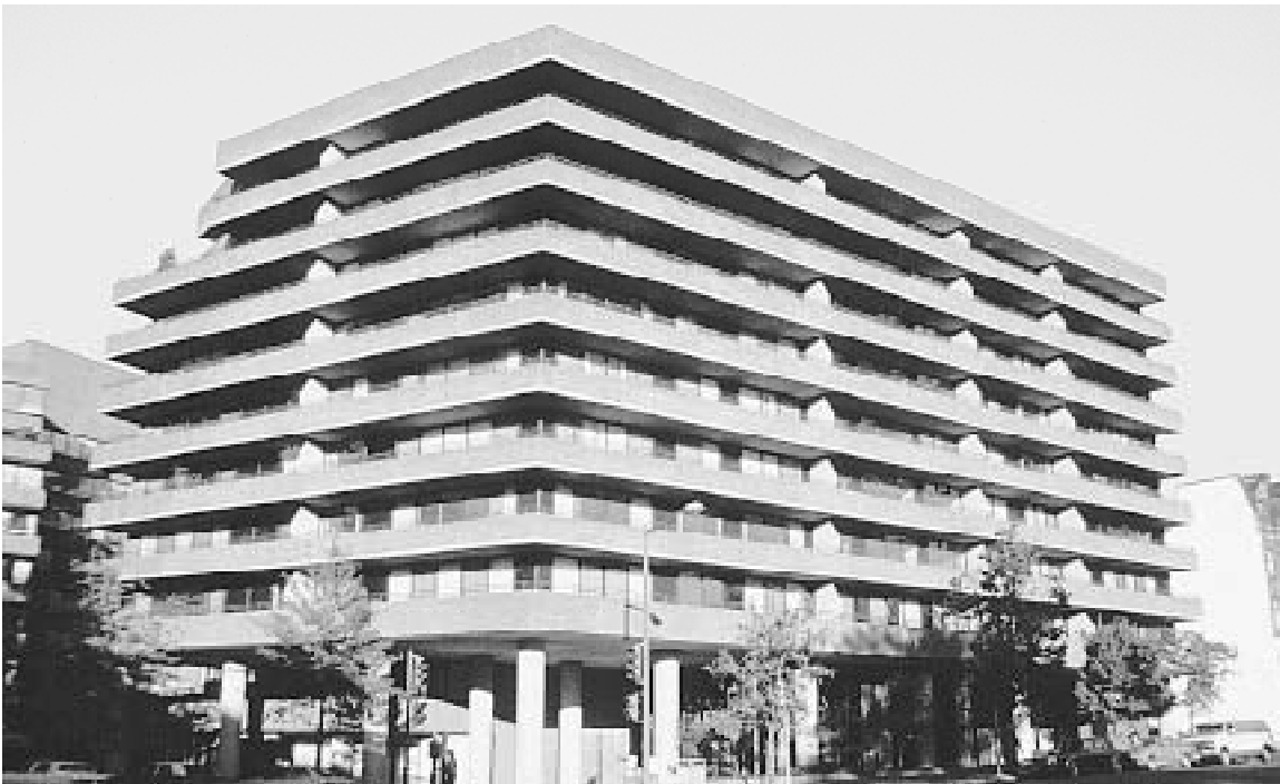
Fig. 1 Horizontal shelves These can be every effective for reducing cooling load on the south side of a building. As seen here, sunlight gets under the shelves on other orientations. These also serve as balconies, a nice touch that is rare in office buildings. They make window washing much easier, protect the glazing, and protect the surroundings from falling glass.
