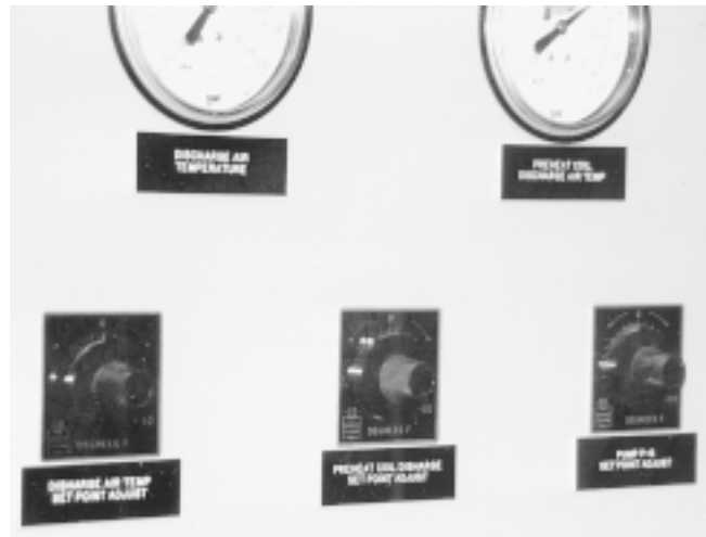
Fig. 3 Air handling system temperature controls These settings can have a major effect on system energy consumption. In single-zone and reheat systems, do not raise the preheat coil discharge temperature higher than needed to avoid freezing and stratification.
