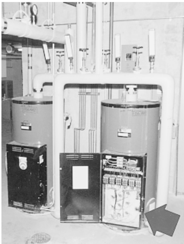
Fig. 1 Interruptible water heating The arrow points to a small relay that the electric utility installed to interrupt the operation of the water heaters during periods of high electrical load. In return, the utility offers the electricity for the heaters at lower prices.
