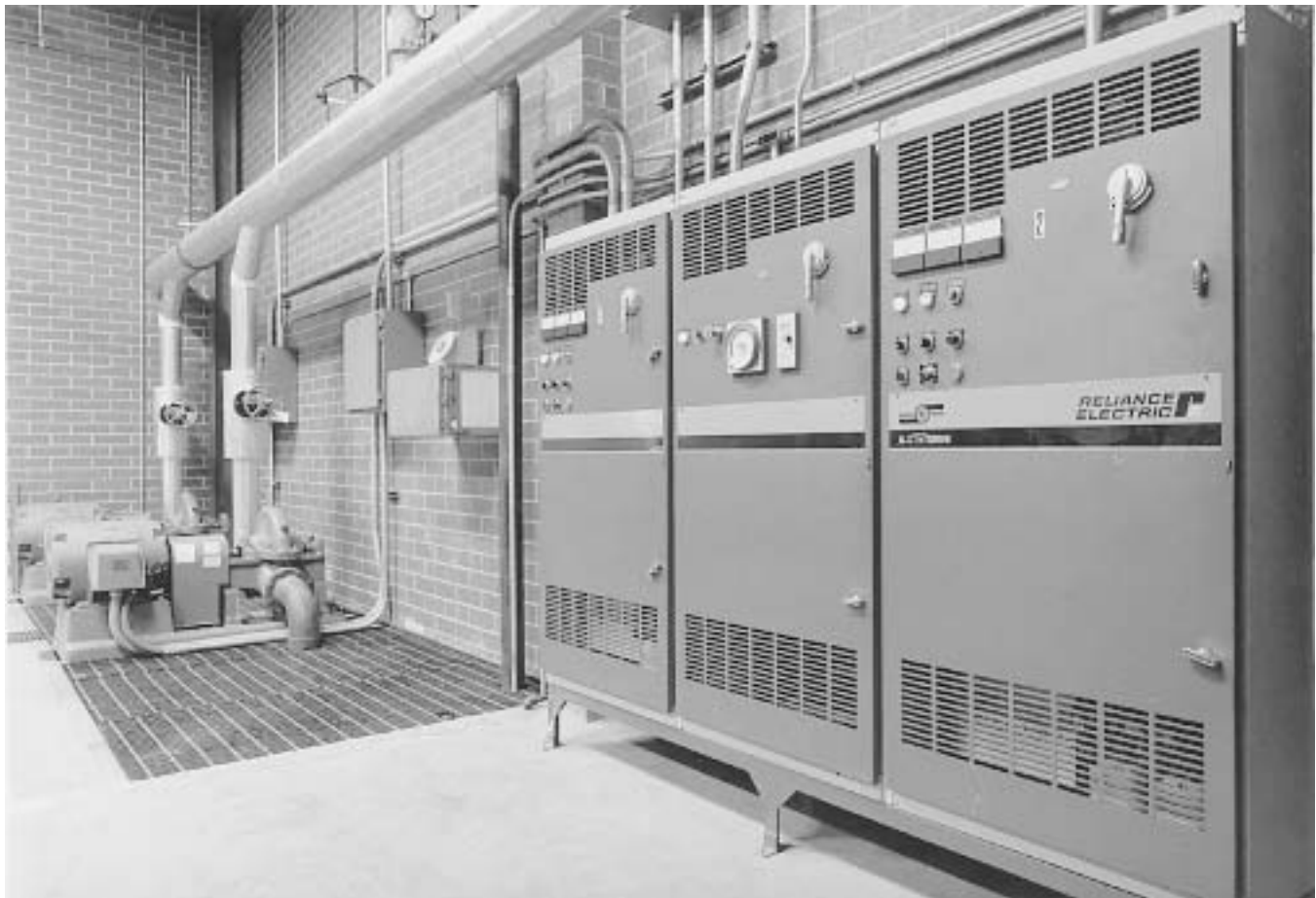
Fig. 3 Variable-frequency drives for large pumps The cabinets are full of solid state electronics and electrical filters. There are no moving parts, and little audible noise. The drives can be installed anywhere with respect to the location of the equipment. The size of the cabinets is roughly proportional to the power of the motors being driven.
