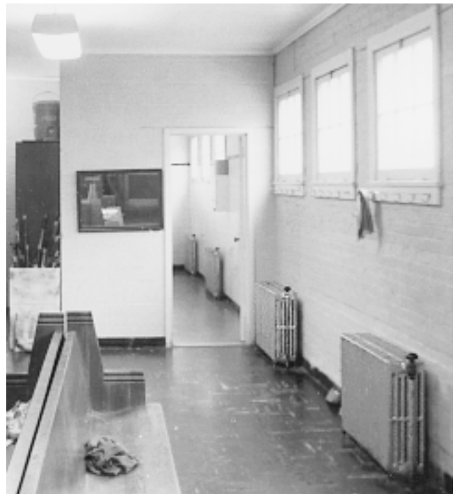
Fig. 2 Group of radiators For good space temperature control, all these radiators could be controlled collectively by installing conventional control valves and a single space thermostat.
