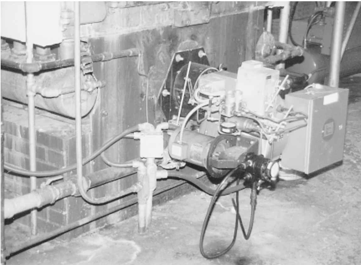
Fig. 10 A modern burner retrofitted to an old brick-set watertube boiler Whether this is a prudent upgrade depends on the efficiency and condition of the boiler. Matching a modern burner to an old boiler involves a number of issues that affect efficiency and reliability.
