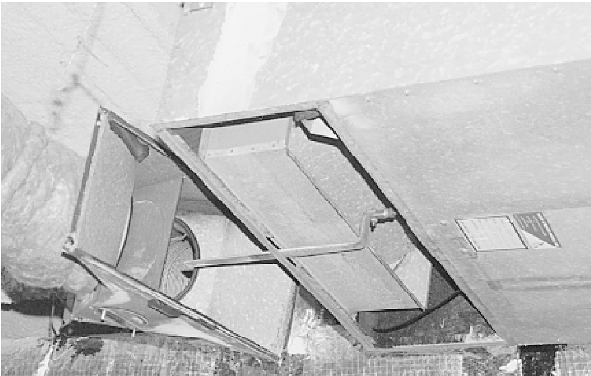
Fig. 2 Mixing vane in dual-duct terminal unit This is the unit shown in Figure 1, looking into the ends of the chilled air and heated air ducts. The air is proportioned by a simple vane that swings between the two duct openings, so that the total flow remains approximately constant. The amount of energy wasted by air mixing is enormous, often much larger than the conditioning load of the space.
