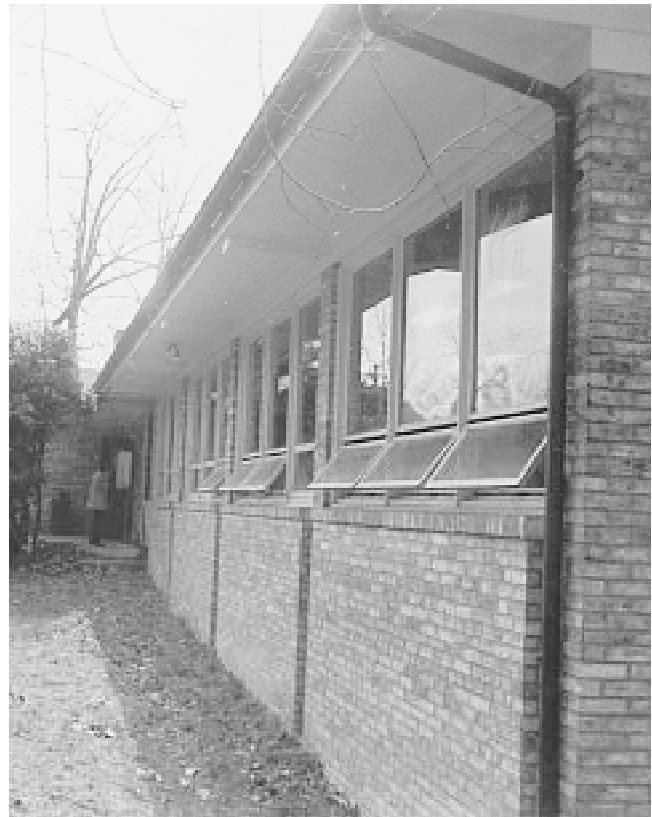
Fig. 5 Roof overhang The shadow pattern shows that the roof overhang of this library is effective in keeping direct sunlight out of the windows. The open windows show that natural ventilation is cooling the building, assuming that the air conditioning has been turned off.
