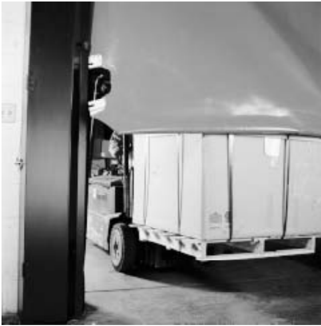
Fig. 5 Breakaway feature Most quick-acting doors protect themselves against major impacts by breaking free of the frame. The design of the door should allow it to be replaced in the frame quickly when this occurs.
