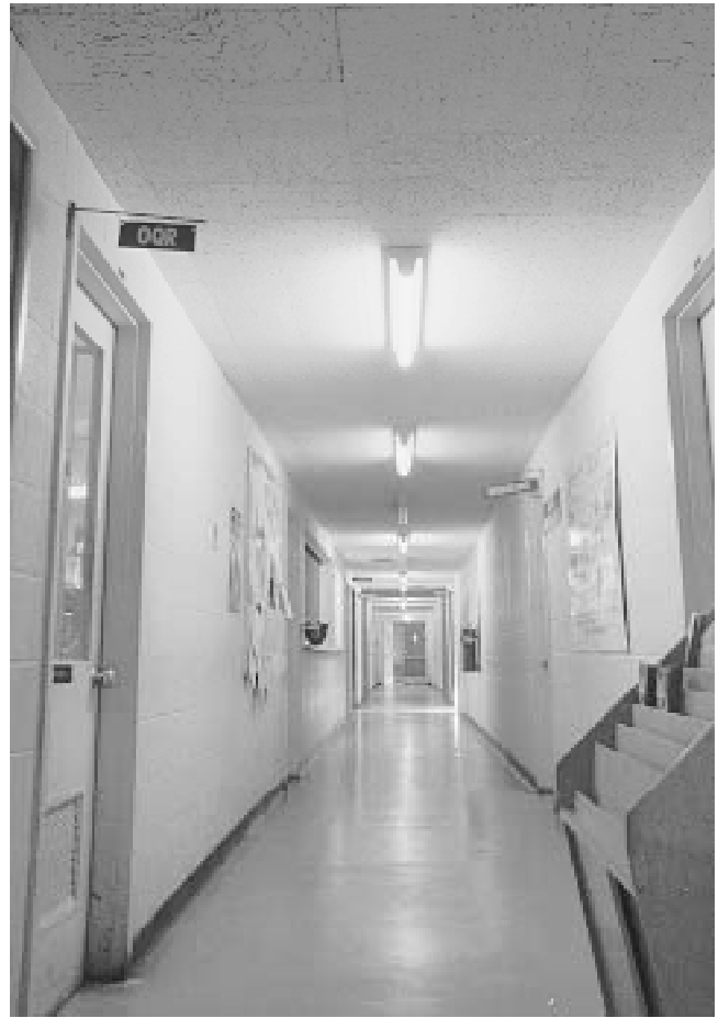
Fig. 2 Fixture orientation matters as well as location This scene shows clearly that a long fixture emits light mostly perpendicular to its axis. Rotating the fixtures 90 degrees will distribute light along the corridor more uniformly. To avoid the glare that would result, it is also necessary to suspend short glare shields from the ceiling, halfway between the fixtures. The same principle applies to tunnels, walkways, etc.
