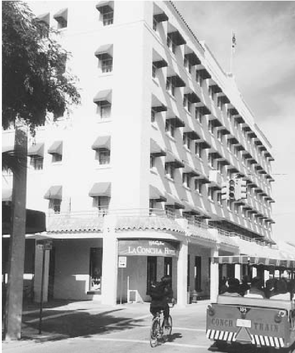
Fig. 17 Awnings Canvas awnings provide effective shading for the rooms of this hotel in a warm, sunny climate. The wall to the right faces east. As you can see from the shadows, the narrowness of the awnings allows some direct sunlight to enter the windows. This could be minimized by tapering the sides of the awnings outward. The awnings provide an important decorative accent for this plain rectangular building. However, fabric has a rather short service life.
