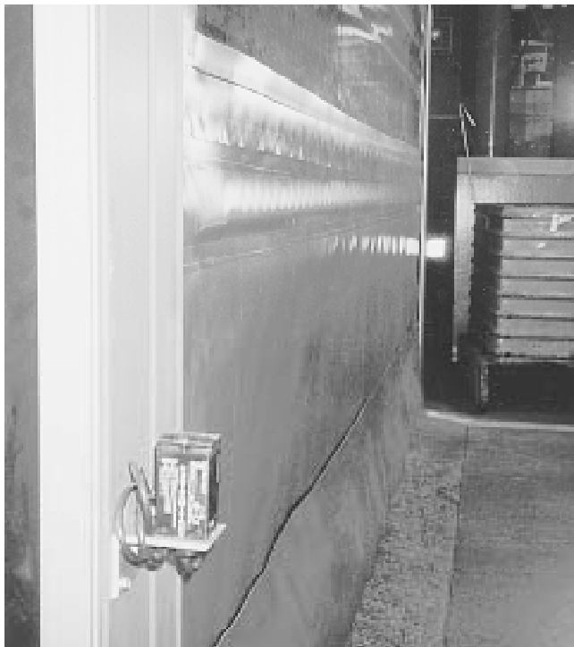
Fig. 7 Light beam safety switch This safety device holds the door fully open as long as the light beam is interrupted.
