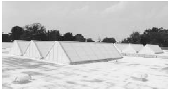
Fig. 8 Large skylight arrays These illuminate areas of a public library with relatively low ceilings. The areas immediately beneath the skylights receive too much illumination and heat gain in bright daylight, while the light is unable to disperse to the rest of the space.
