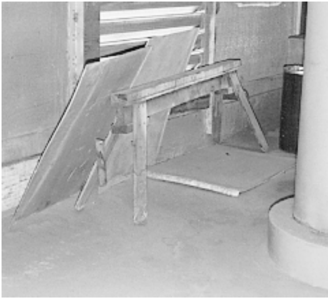
Fig. 1 Blocked combustion air intake This air intake to a large boiler plant was blocked to keep the cold outside air from causing discomfort inside the plant.
