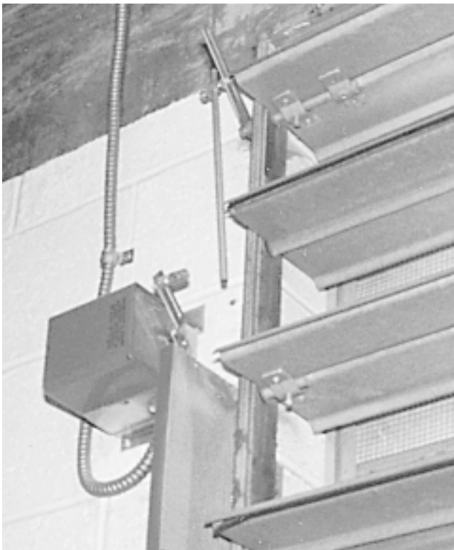
Fig. 3 Common damper problem For some reason, damper manufacturers have not yet figured out how to keep a simple rod connected reliably. Therefore, you have to keep checking.
