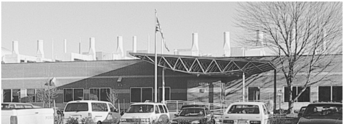
Fig. 3 High-velocity exhaust stacks These exhaust stacks on a laboratory building reduce recirculation into the building. This method cannot completely eliminate recirculation. If the exhausted air is cooler than the surrounding air, it will fall back to the surface. Under such conditions, wind is needed to carry away the exhaust.
