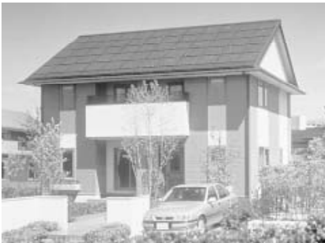
Fig. 6 Residential photovoltaic system Photovoltaic cells cover one side of the roof of this house in Japan. The system provides enough power for the average needs of the house, but batteries are needed to match the generation of power to the time of use.
