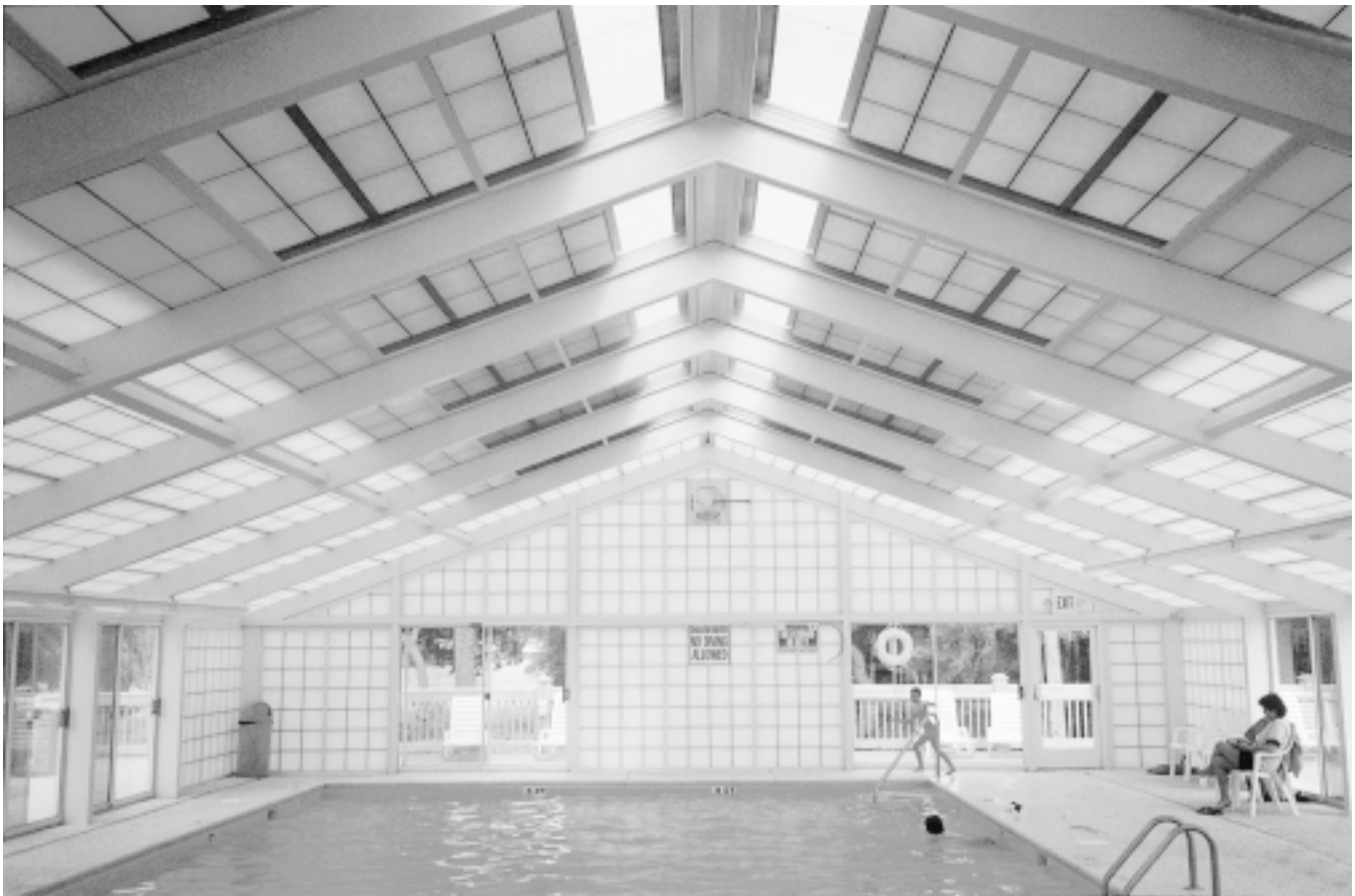
Fig. 3 Swimming pool enclosure This swimming pool at an all-year campground uses an intelligent combination of translucent insulated panels, clear glazing, and venting. Notice that the upper portions of the roof can slide back to provide venting and daylight.
