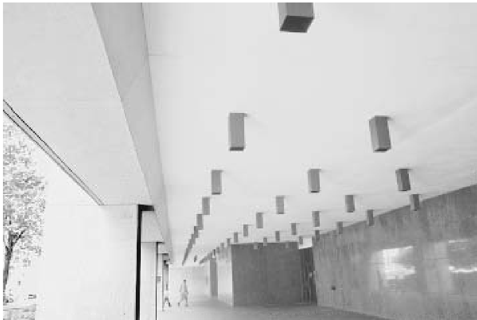
Fig. 4 Downlight abuse in a university building entrance This forest of downlights is intended to provide security for the entrance to an urban classroom building. Most of the light that escapes from the highly absorbing fixtures is lost in the dark stone floor. About three small surface-mounted HID lamps would provide vastly better illumination, at a small fraction of the energy and lamp replacement cost.
