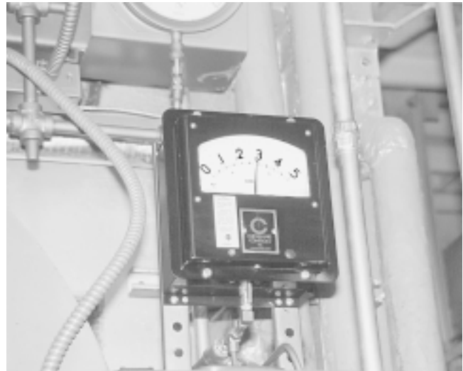
Fig. 4 An air casing pressure gauge This is on a large boiler with a forced-draft fan. Draft is just as important in big boilers as in small boilers.
