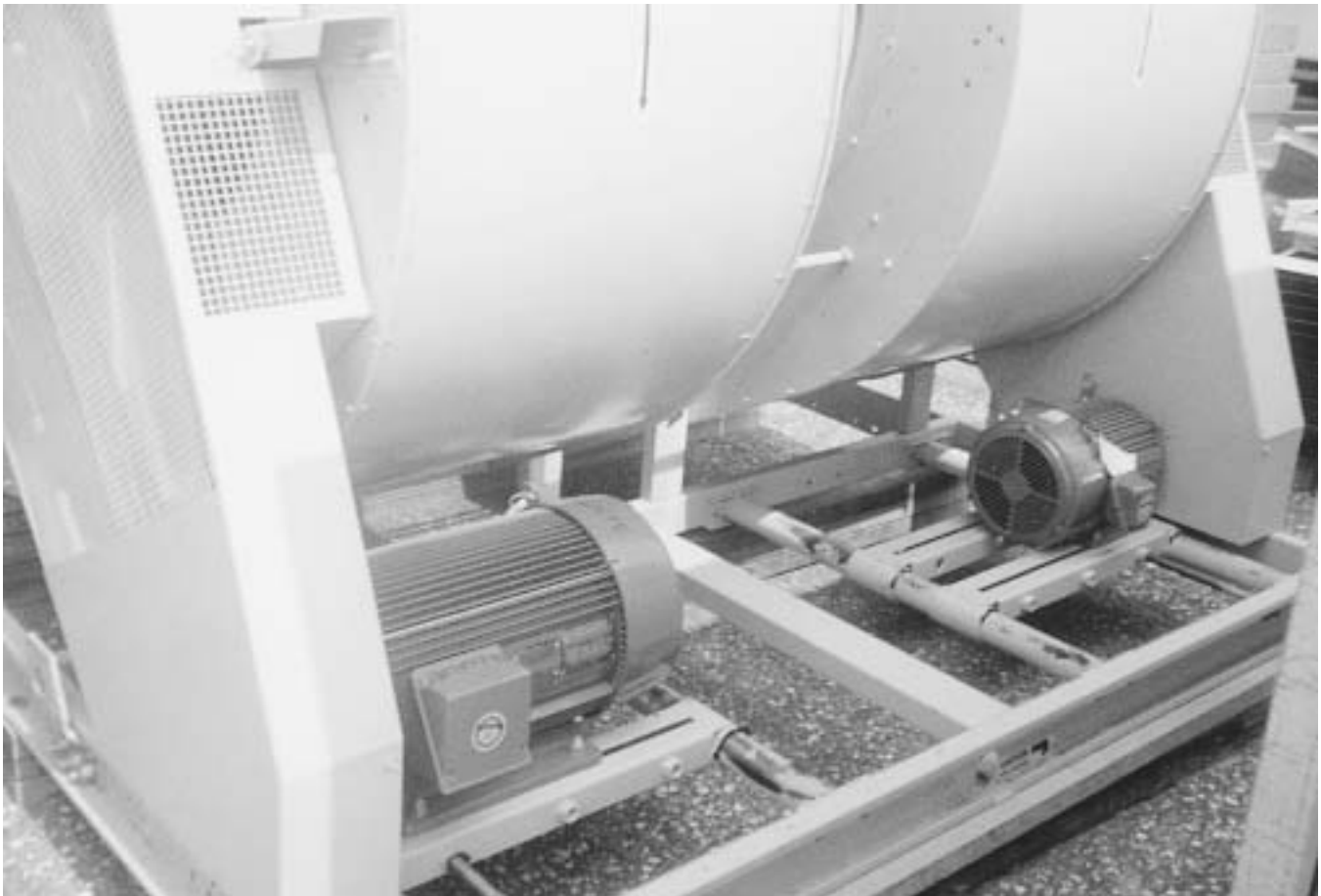
Fig. 2 Two-motor fan drive for a cooling tower The two centrifugal fans are driven by a common shaft. The larger motor drives the shaft from the left side, for high speed operation. The smaller motor drives the shaft from the right side, for low speed operation. Each motor is connected to the shaft by drive belts, allowing any possible combination of two speeds to be selected. When each motor operates, the other idles. Multiple-motor drives can be used for many applications. The motors are entirely standard, and no special drive equipment is required.
