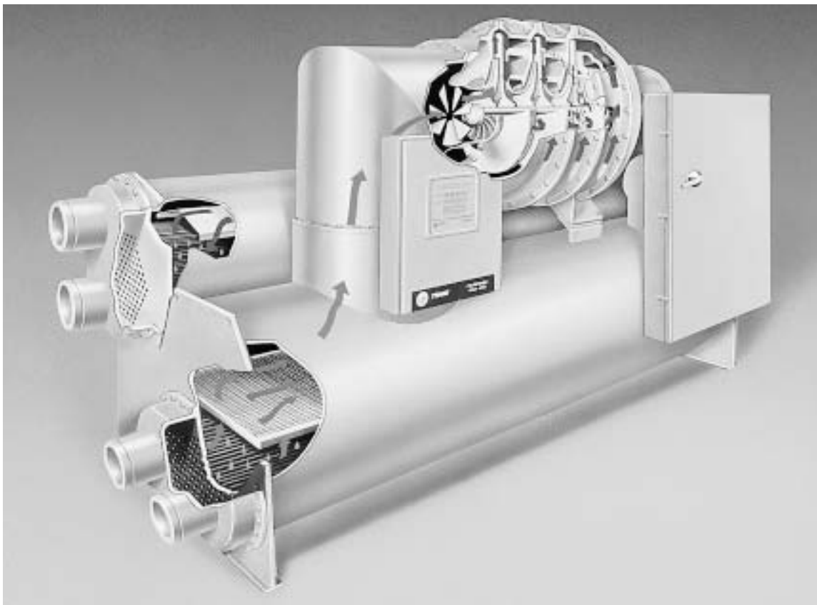
Fig. 2 Packaged water chiller The machine packages all the primary elements of a cooling system together. This model has a three-stage centrifugal compressor. The cooling output of the machine is controlled by throttling the flow of gas into the compressor with an inlet vortex damper. The evaporator, at bottom, is flooded with refrigerant. Tubes for chilling water are immersed in the refrigerant. The refrigerant evaporates under the reduced pressure of the compressor suction, chilling the water. The vapor is compressed to a hot gas by the compressor, and is discharged to the condenser in the rear. Cool water from a cooling tower flows through the tubes in the condenser, absorbing heat from the hot gas and condensing it. The warm refrigerant liquid drops down into the evaporator through an orifice. Upon exposure to the lower pressure in the evaporator, a portion of the warm refrigerant liquid evaporates, cooling the remaining liquid to the saturation temperature that corresponds to the evaporator pressure. The cycle continues as long as the compressor runs.
