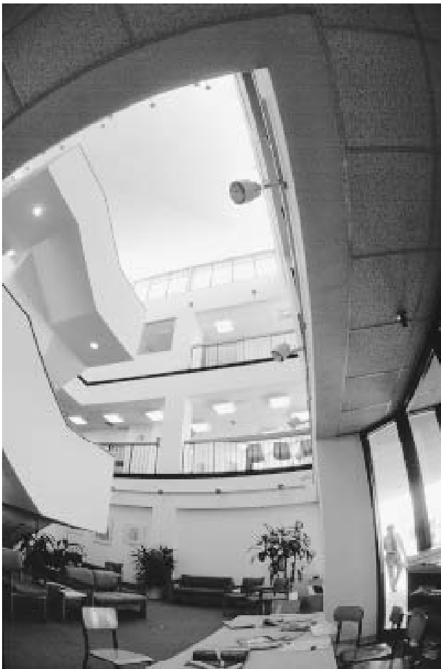
Fig. 10 An expensive daylighting installation that saves no energy A lot of useful space in this office building was given up to create an atrium illuminated by a large skylight. However, note the electric lights that are turned on everywhere around the perimeter of the atrium. These attempt to equalize the illumination levels of the shaded areas with the sunlit areas. Someone probably won a design award for this.
