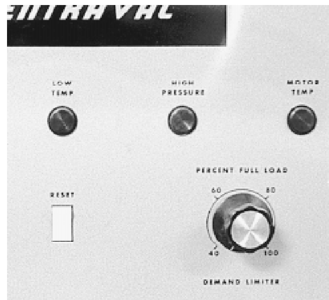
Fig. 1 "Demand limiter" This control limits the maximum output of the chiller. It is called a demand limiter because it is intended to limit electricity demand charges. You can also use it to shift the cooling load among chillers.
