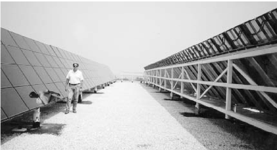
Fig. 5 Large photovoltaic system This is part of an array of many similar rows of photovoltaic cells that cover the roof of a large classroom building. The array provides a peak capacity of about 100 kilowatts, which is one fourth of the peak load on the building. The system supplements power provided by a public utility. The panels are light, thin, easy to mount, and easy to connect together.
