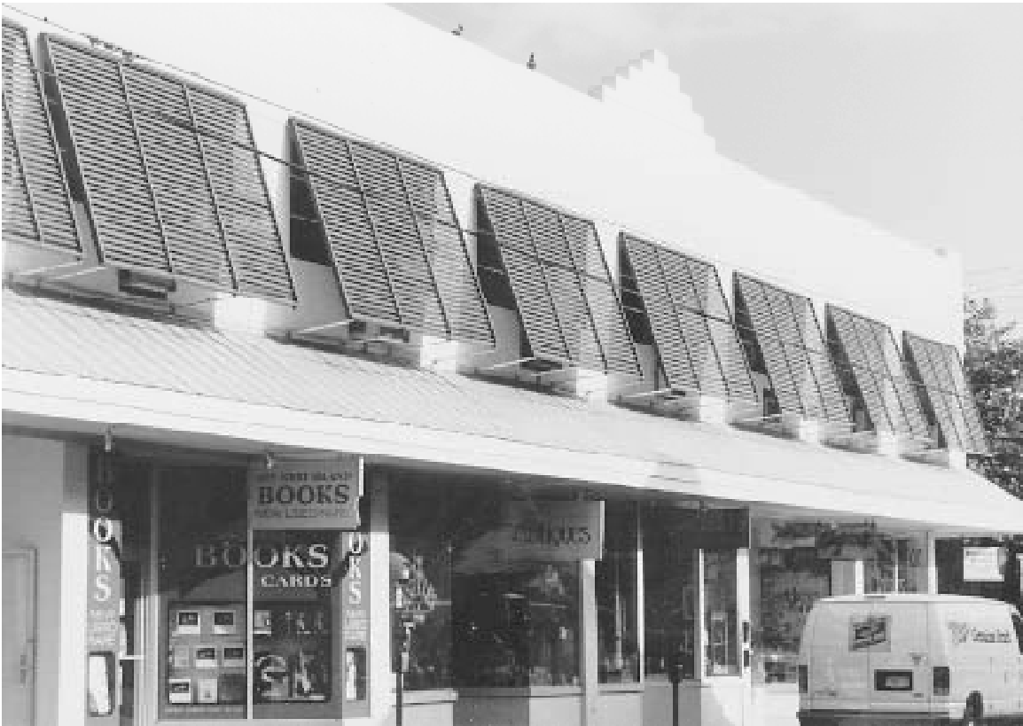
Fig. 12 Louvers installed as awnings These simple louver assemblies on the south side of a modest commercial building provide effective shading, along with a moderately good view of the street below. They have been lengthened to hide air conditioners installed below the windows.
