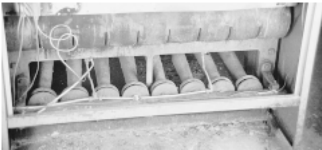
Fig. 2 Another atmospheric gas burner On this furnace, the primary air for each venturi is adjusted by a disk that moves along a threaded rod, providing fine adjustment.
