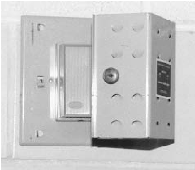
Fig. 3 Opaque thermostat cover This is better than a transparent cover, but it still tells occupants that they cannot control their temperature. These are frequently knocked off the wall. Why does this cover have a sticker that tells occupants how to set the temperature?
