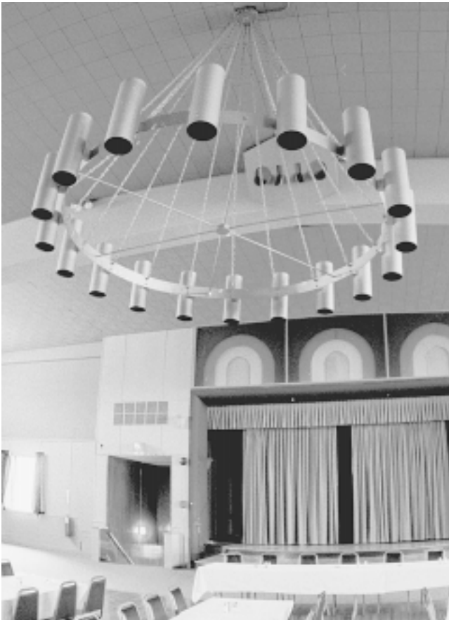
Fig. 2 Quirky chandelier This unattractive chandelier has the energy waste of 18 downlights, and equally bad light distribution. Replacing the cylinders with globes or some other open type of lamp mounting would make it much more effective.
