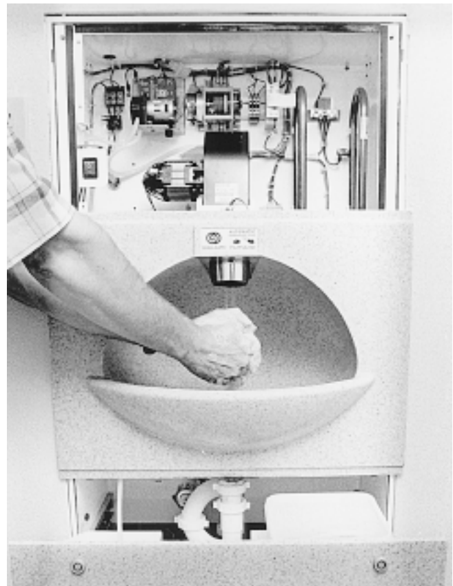
Fig. 3 Automatic hand washing station This basin includes a soap dispenser, faucet, and hot air dryer, all operated automatically. The covers are removed to show the equipment inside.
