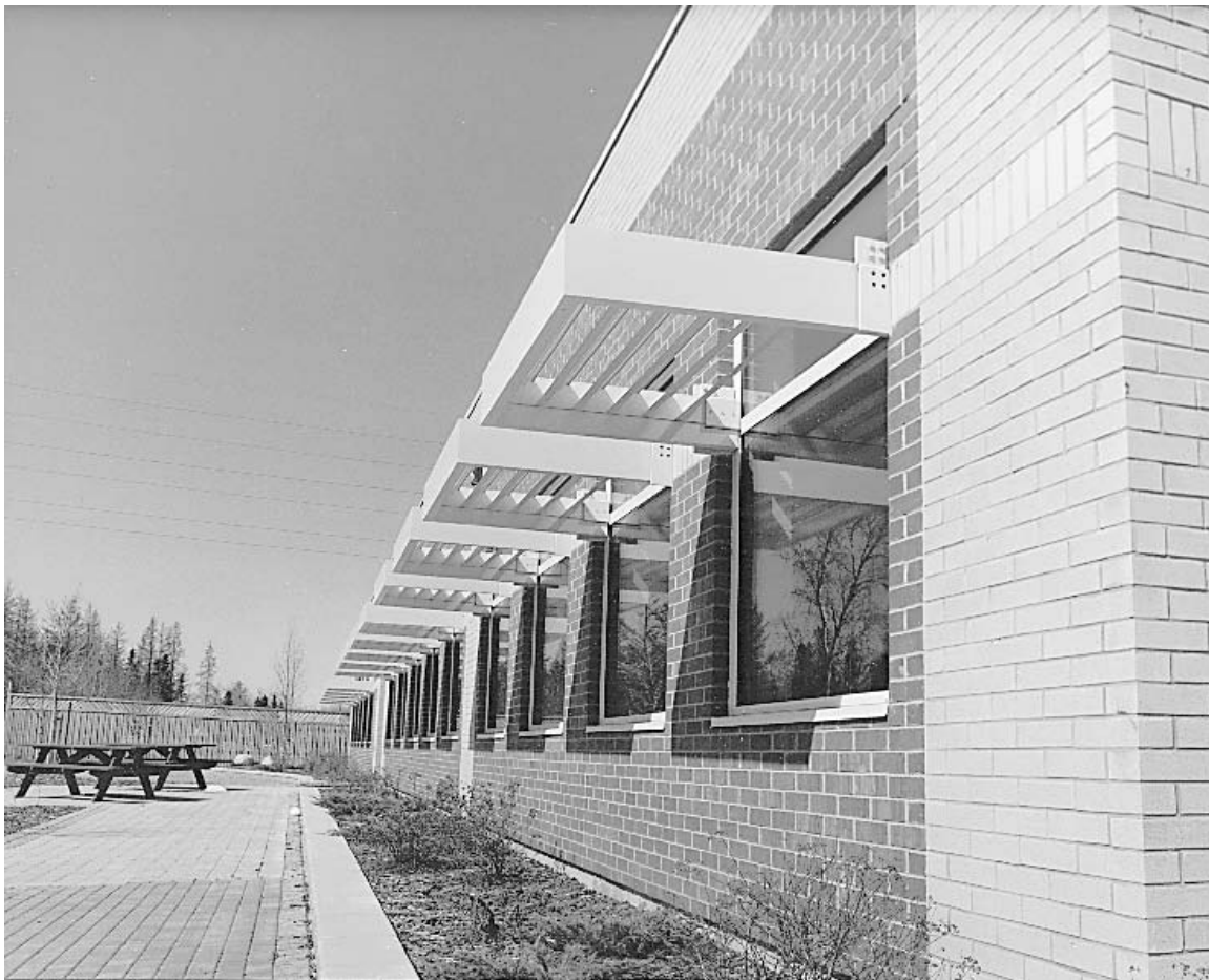
Fig. 4 Exterior shades that work with light shelves These are unusual because they are installed below the tops of the windows, at the same height as the light shelves. Their purpose is to keep direct sunlight from entering the portions of the windows below the light shelves. The shadow pattern shows that the shades would be more effective if they were installed as a continuous unit. Exterior shades can increase daylighting by reflecting more light into the top portions of the windows. This design fails to exploit that opportunity.
