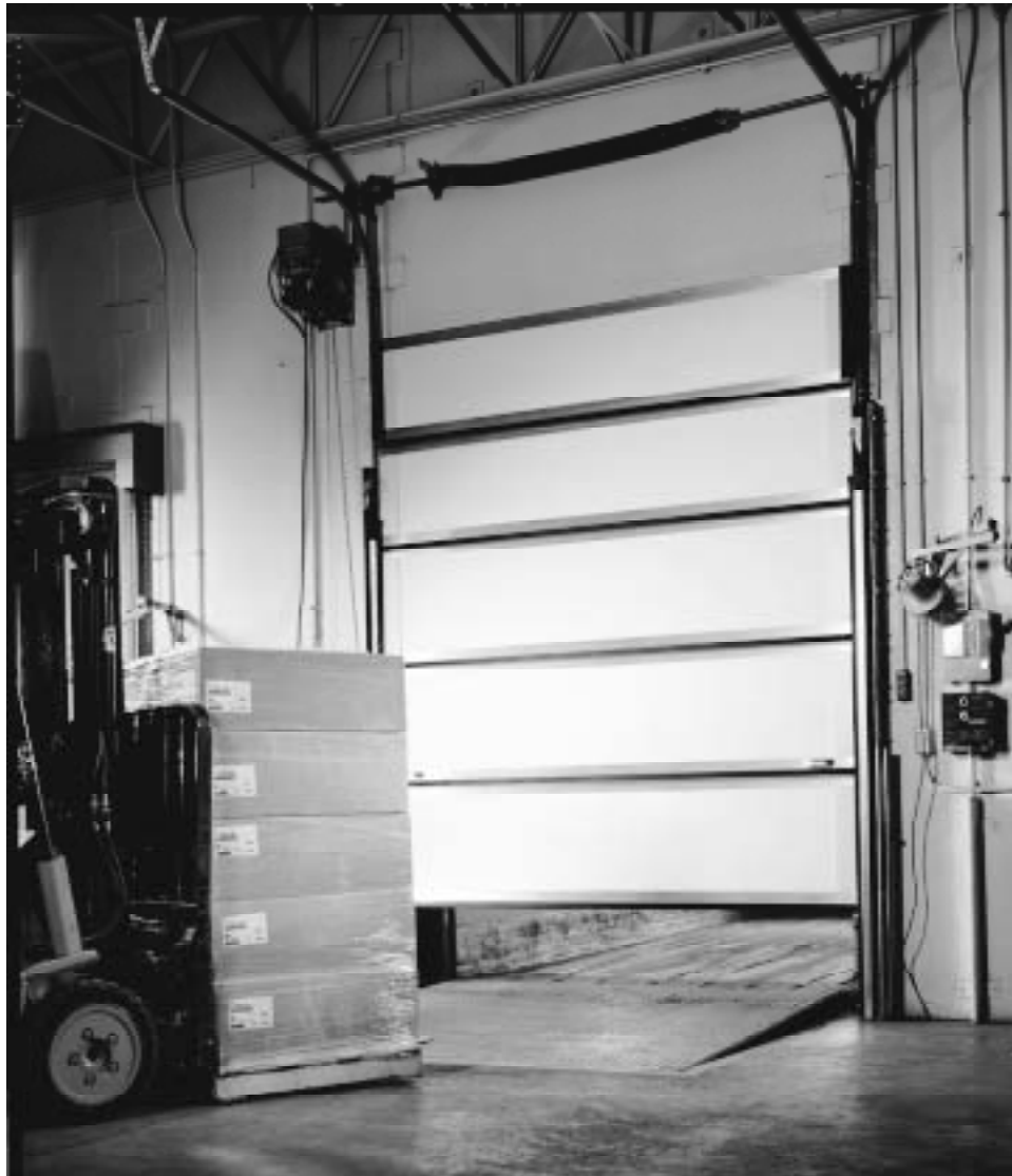
Fig. 4 Overhead sectional quick-acting door This is a variation of the common garage door. In addition to a powerful motor, the main differences are lighter weight, effective seals on all sides, and breakaway panels. The panels can be insulated.
