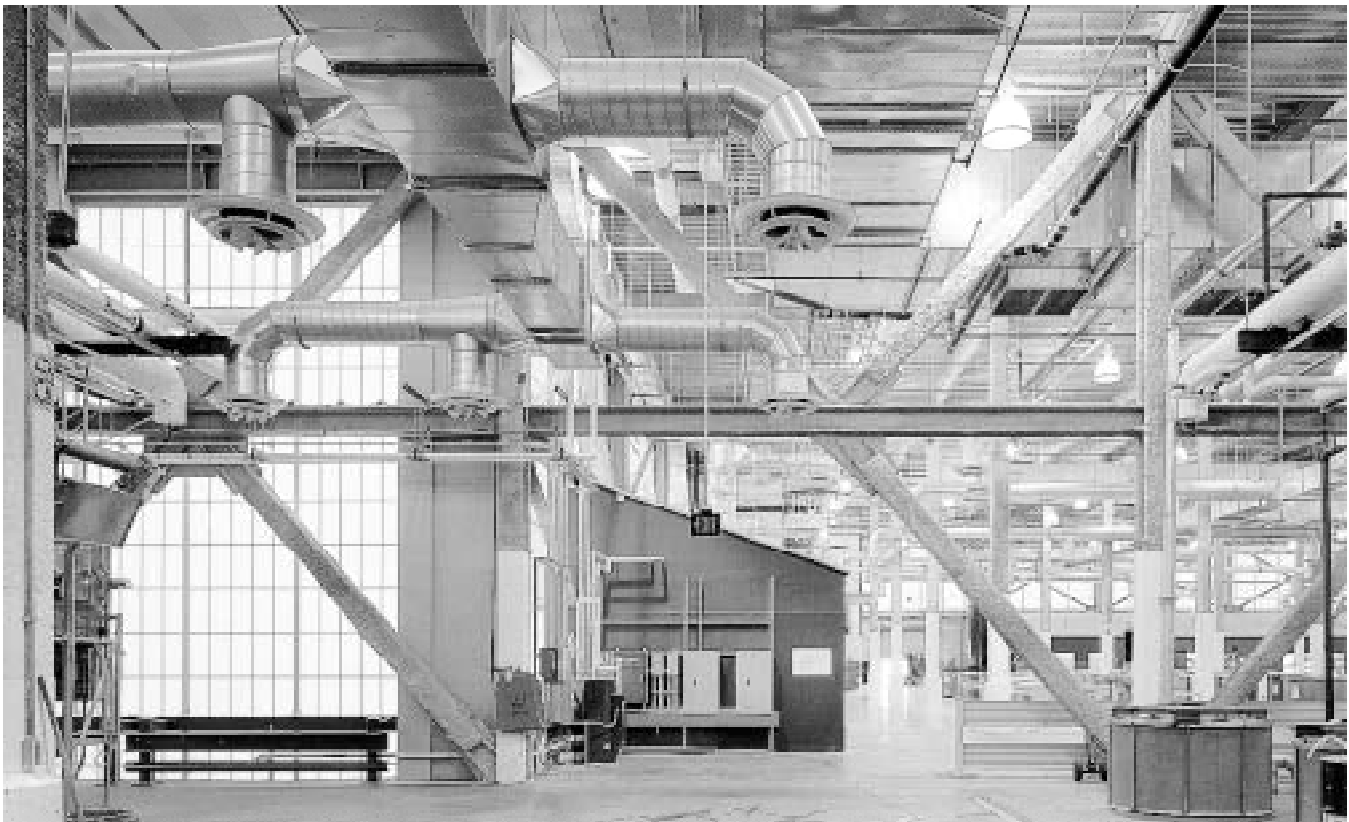
Fig. 1 Extensive use of translucent panel construction in a manufacturing plant The translucent panels provide daylighting from overhead and from the sides. Small conventional windows provide view. The bottom photo hints at the degree of daylight penetration on a lower floor. Note the placement of the light fixtures.
