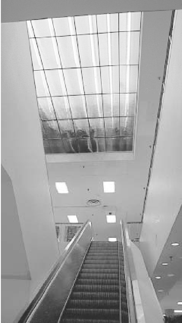
Fig. 5 Ceiling plenum lighting This escalator in a department store is illuminated by fluorescent strip fixtures located in the ceiling plenum. Grilles let some of the light escape, but this arrangement is an expensive light trap. It has no advantage over conventional fluorescent fixtures.
