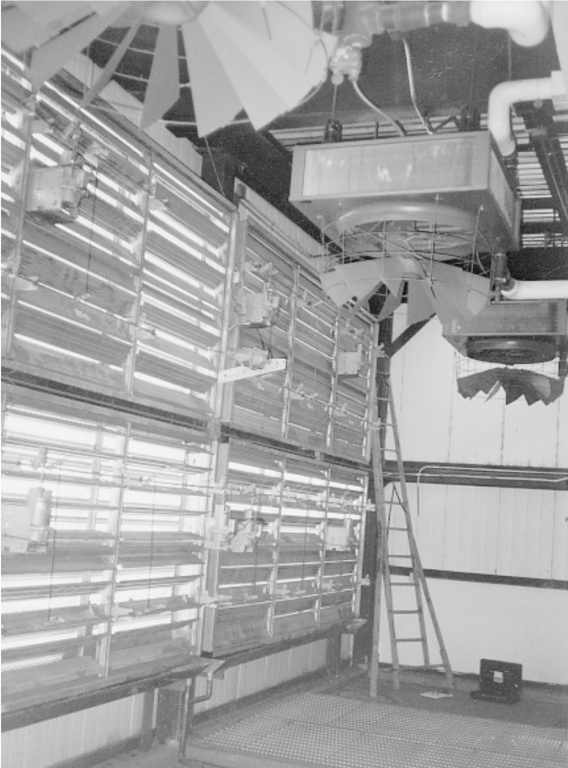
Fig. 1 Large damper array An installation like this cannot control low air flow rates reliably, and it cannot prevent major infiltration when the facility does not need outside air. Note the large unit heaters, probably installed for freeze protection. Such a high-energy alternative to good dampers is a very bad bargain.
