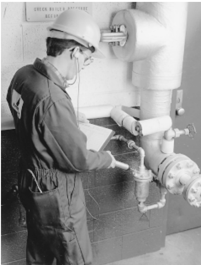
Fig. 1 Trap inspection service Consider a professional service to test and/or repair your steam traps if this approach would provide greater skills or consistency.
