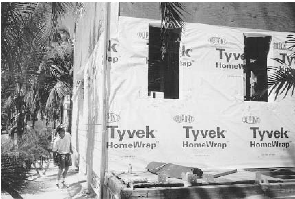
Fig. 3 This is not a vapor barrier This is a house wrap. It must be made of appropriate permeable material. Using vapor barrier material as a house wrap would cause moisture damage in the walls. The outer sheathing of this house is plywood. If the plywood is well installed, the house wrap is superfluous.
