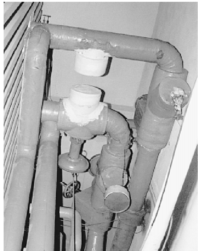
Fig. 6 A large bypass control valve converted to throttling operation The control valve for this enormous air handling unit was converted to throttling operation simply by eliminating the bypass path. Major energy savings result. However, it becomes more critical to operate the correct number of chilled water pumps.
