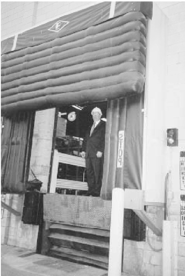
Fig. 3 Inflatable dock seal The upper part of the seal is inflated, the sides are not. Note the guide post, the bumpers to keep the trailer from backing too far into the seal, and the stoplight. Correct alignment is essential for sealing and for protecting the seals.
