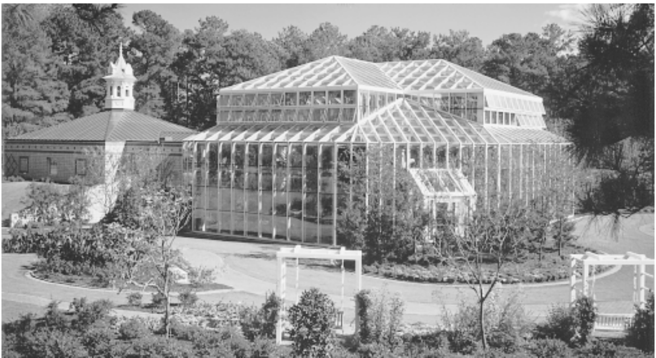
Fig. 1 Plain and fancy greenhouses The upper one is made entirely of extruded double-wall plastic. The bottom one is made of glass. All glazed enclosures should apply the lessons that have been learned from a vast number of greenhouses. In both of these, notice the extensive vents that are located at high points. Venting is necessary for free temperature control in any application.
