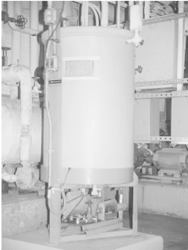
Fig. 1 Automatic boiler water chemical feeder This is simply a plastic storage bin with an injection pump installed underneath. This equipment tends to clog, so don't neglect it.
