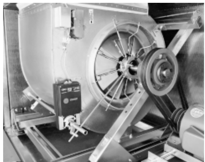
Fig. 4 Fan with inlet vortex damper This method of fan modulation is most efficient at high percentages of output. It is much less efficient than speed modulation at lower outputs. Its main attraction is low cost.
