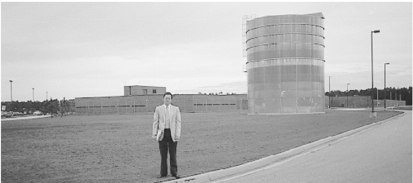
Fig. 19 Chilled water storage This system provides air conditioning for a Florida prison. The huge tank was originally designed to hold water for fire protection. It functions well in both roles.
