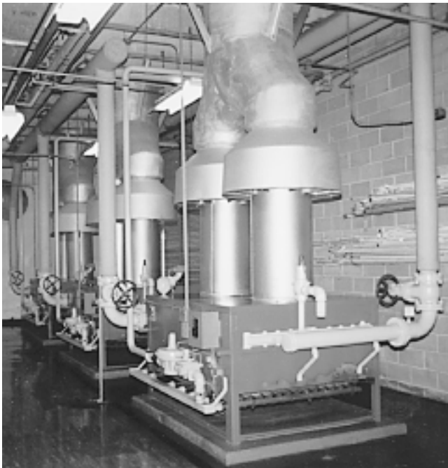
Fig. 1 Draft hoods Air from the boiler room freely enters the flues from underneath the hoods. These boilers are unusually large to have draft hoods. They are used because the boilers have atmospheric burners.
