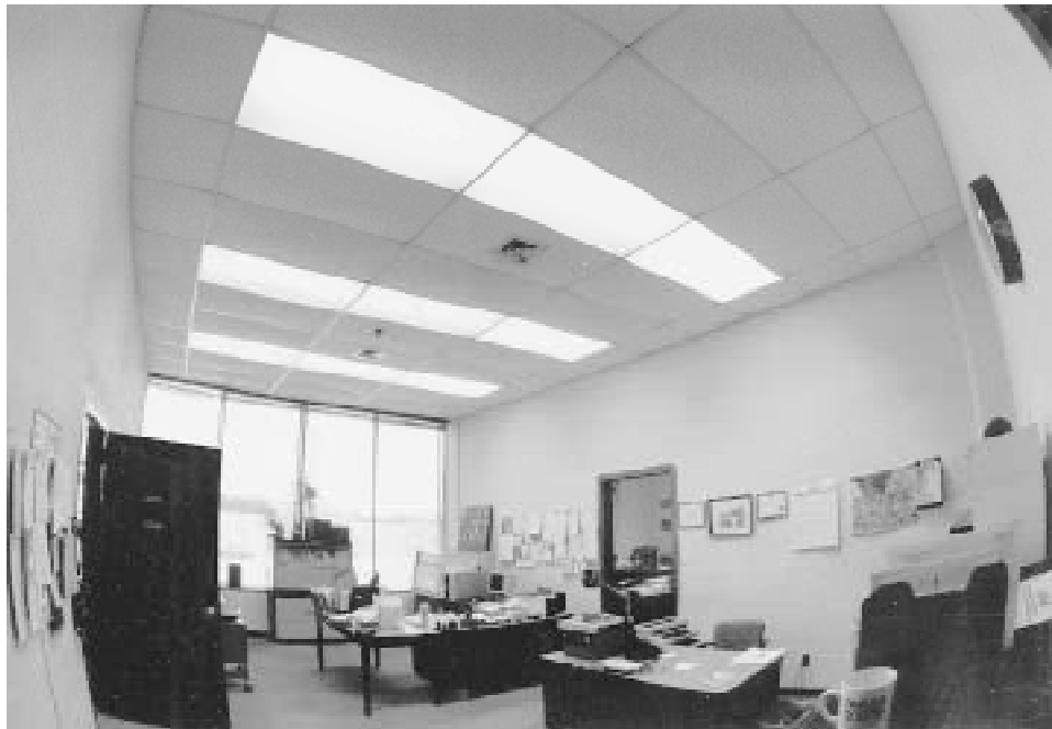
Fig. 1 Inadequate light fixture circuiting All the lighting in this office is controlled by a single switch. The row of fixtures adjacent to the windows should have a separate circuit, to exploit daylighting. The fixtures in all three rows on the same side as the door should have separate switches. Even better, they should be removed. 36 fluorescent tubes is far too many for two desks. This room needs extensive delamping, or even better, task lighting.
