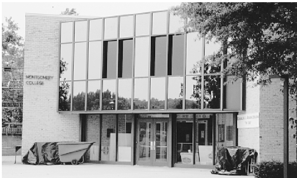
Fig. 2 Curtain wall upgrade The original exterior, above, was replaced with the one below. Although they appear similar, the new curtain wall has much better insulation value and somewhat less glazing area. The improvement made it possible to abandon the original perimeter heating units, rather than replacing them.
