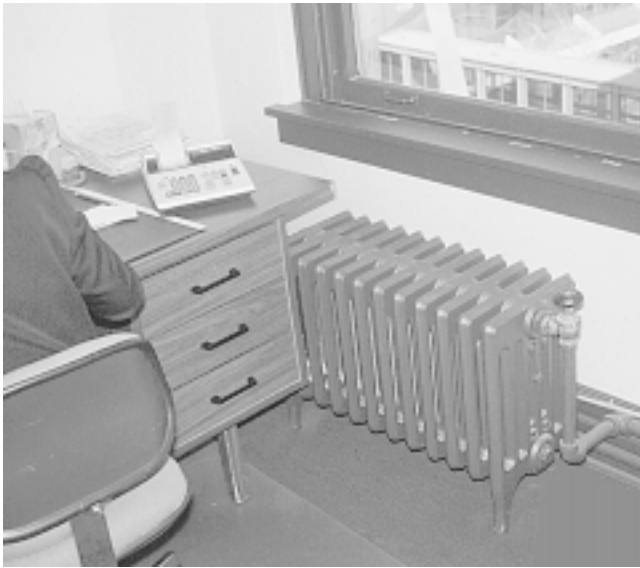
Fig. 1 Radiator with manual control valve This radiator can be retrofitted easily with a self-contained thermostatic valve. The high position of the valve and the length of hot steam pipe under the valve make it advisable to install a valve that has a remote temperature sensor.
