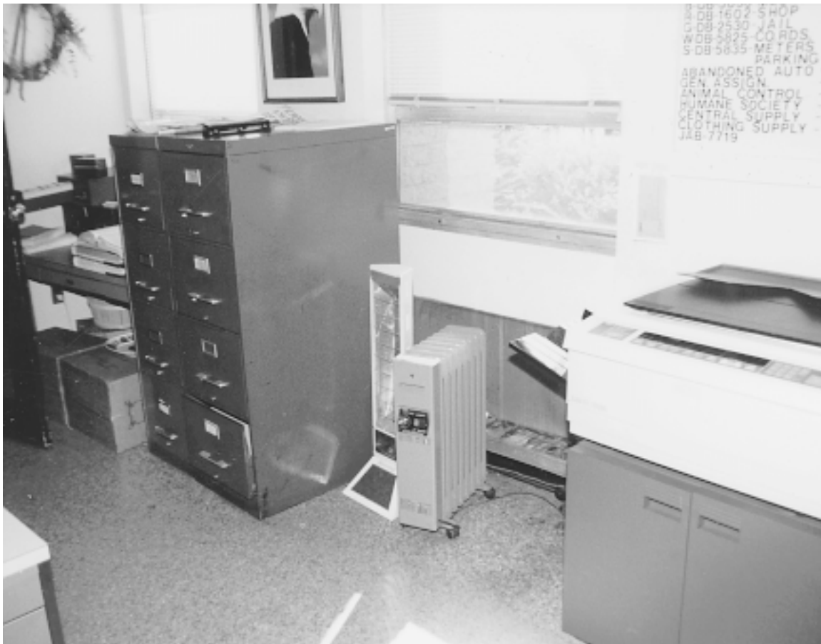
Fig. 2 Obstructed convectors Air return to the convectors is blocked by the file cabinets and copy machine. Discharge from the convectors is obstructed by the table at left and by an accumulation of debris. The heat that does escape from the convectors is first confined against the uninsulated exterior wall, through which a fraction is lost. Note the electric heaters that compensate for these problems.
