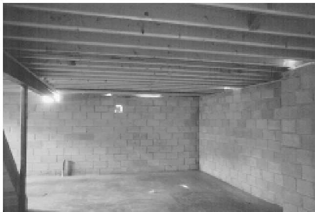
Fig. 5 Foundation plate, from inside Daylight shows where air can leak into the building. There are large gaps at the foundation plate and around the end of the center beam.
