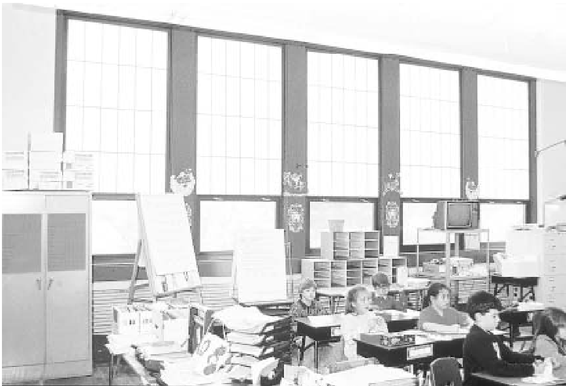
Fig. 3 Window retrofit with diffusing panels The top is the original configuration, with clear windows and roller shades. Notice that the outer row of light fixtures is turned on. The bottom shows the diffusing windows installed. These provide deeper daylight penetration and reduce heat loss. Some outside view is provided by clear hopper windows at the bottom, which can also be opened for ventilation. Notice that the children are all facing away from the diffusing windows, perhaps to avoid glare. However, the teacher must face the windows. See Figure 4 for the exterior appearance.
