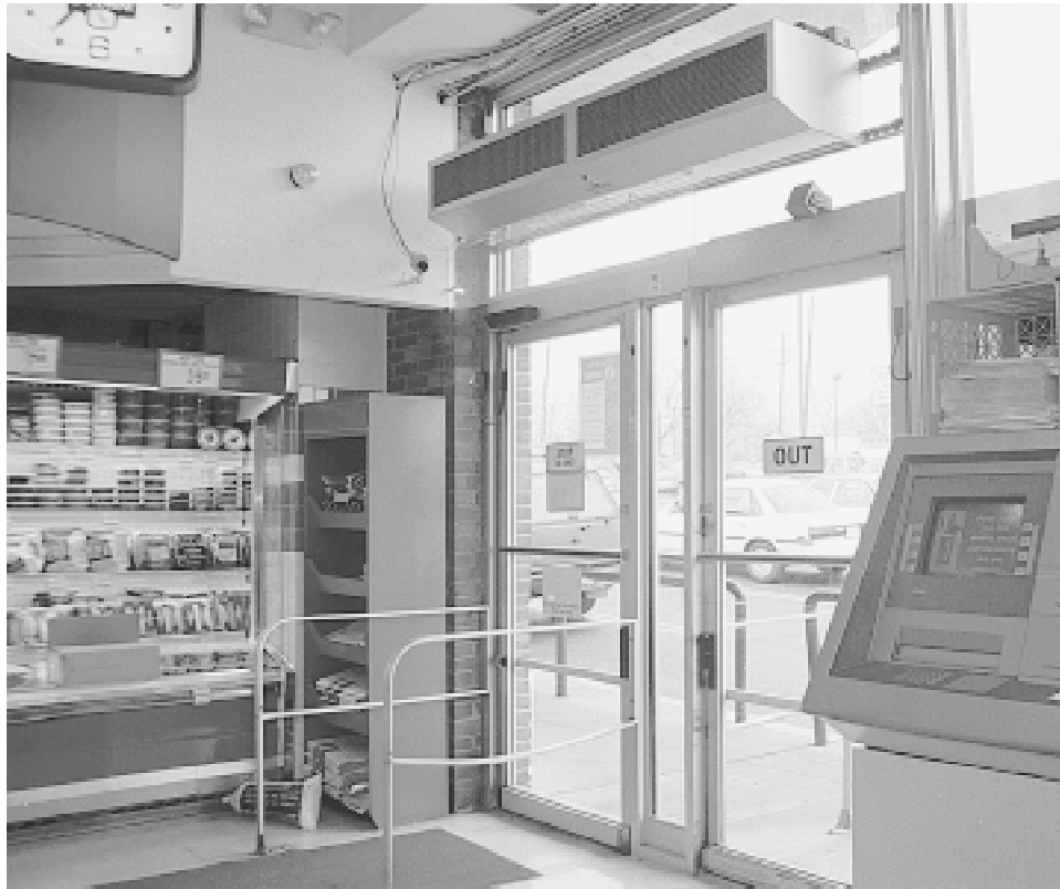
Fig. 1 Automatic swing doors This pair of doors is the main entrance for a large grocery. They operate hundreds of times per day, so they must be rugged and reliable. For safety, each door must swing away from traffic. This requires two doors. The sensors that open each door should be triggered only by traffic from the correct direction. These doors are activated by ultrasonic sensors, which are small, inexpensive, and easy to install. The air curtain installed here plays no significant role in reducing infiltration. It discourages insects.
