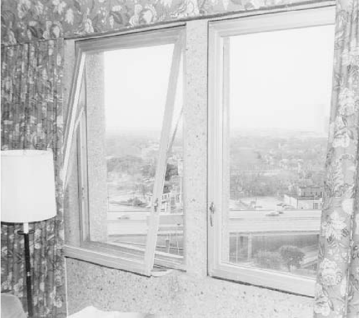
Fig. 1 These windows need switches to turn off the conditioning. This luxury hotel is located in a climate that encourages guests to open the windows, and the ability to do so is an attraction of the hotel. The rooms are conditioned to maintain a precise temperature, so opening the windows can waste a large amount of energy.
