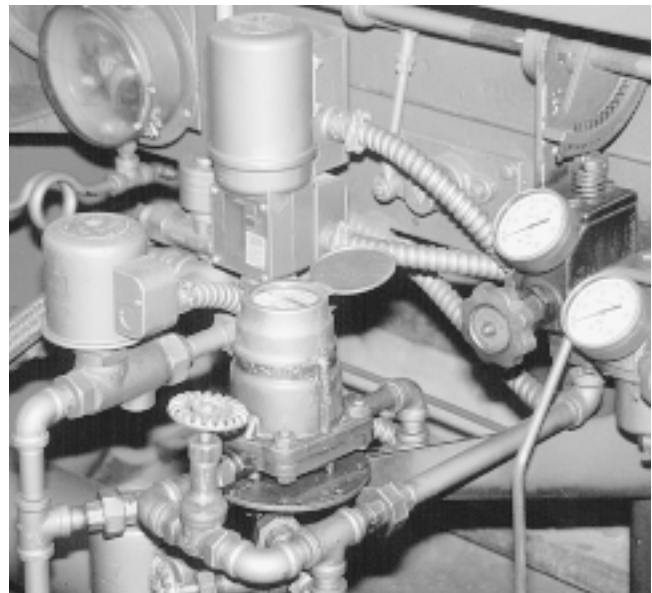
Fig. 3 Fuel meter This accurate, inexpensive device, installed in the fuel oil line to the burner, tells you how much energy is going into your boiler. If combined with an accurate measurement of heat output, it also tells you the average efficiency of the boiler.
