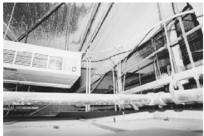
Fig. 3 Inside a soffit over a loading dock The bottom surface, exposed to the outside, is loose fitting ceiling tile. The air space connects to the ceiling plenums and curtain wall spaces of the building. Several heaters are installed to keep water pipes in the space from freezing.
