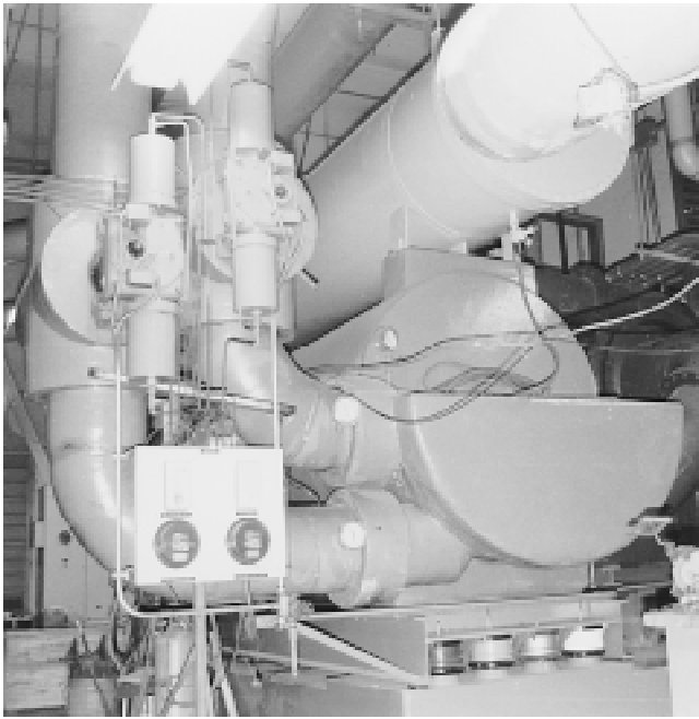
Fig. 7 Automatic evaporator isolation valves These greatly increase the reliability of efficient operation. They are not cheap, but with chillers this size, they pay back quickly.
