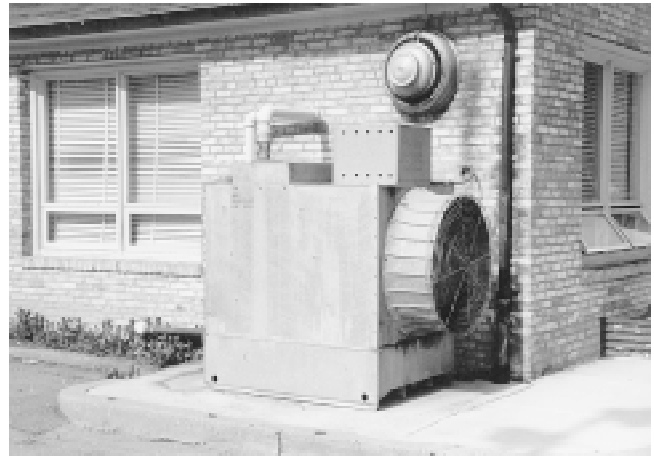
Fig. 1 Horizontal-flow cooling tower If wind blows opposite the direction of discharge, a certain amount of recirculation will occur. Recirculation is aggravated by the location of the tower alongside a wall. This type of tower causes serious recirculation to any other heat rejection units located in the general direction of the discharge.
