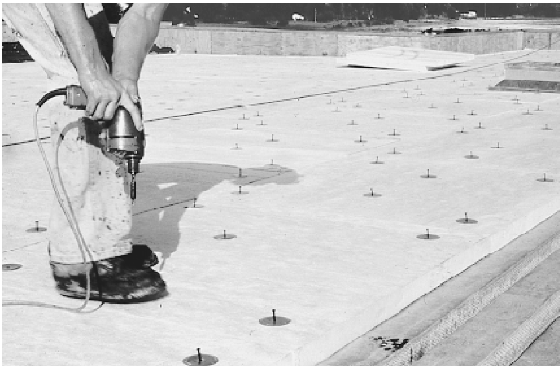
Fig. 1 Rigid insulation applied to a flat roof This insulation is applied in layers. Snug fit is essential, and it is achieved by using many fasteners. The top layer is tapered to provide drainage. However, the small amount of slope provided by tapered insulation does not provide reliable drainage unless the top surface membrane is applied carefully. Even then, the roof drains must collect all water reliably, or the water will work its way underneath the bottom layer of insulation.
