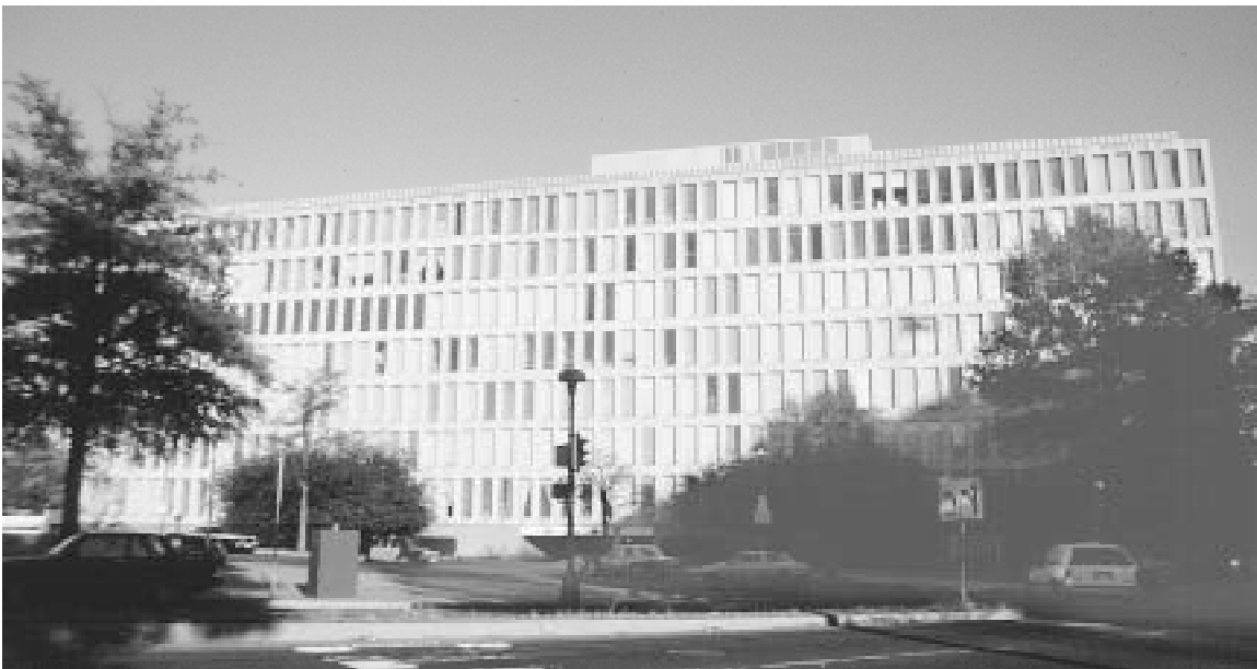
Fig. 1 Typical interior window shading The first effect of most interior window shading is to abolish the window's original purpose, which is to provide a view and daylighting. Almost every occupied space on this side of the building has blocked out daylight completely. However, the windows still cause greatly increased heat loss and heat gain. The light color of the windows indicates that a considerable amount of sunlight is being reflected, but much is still trapped.
