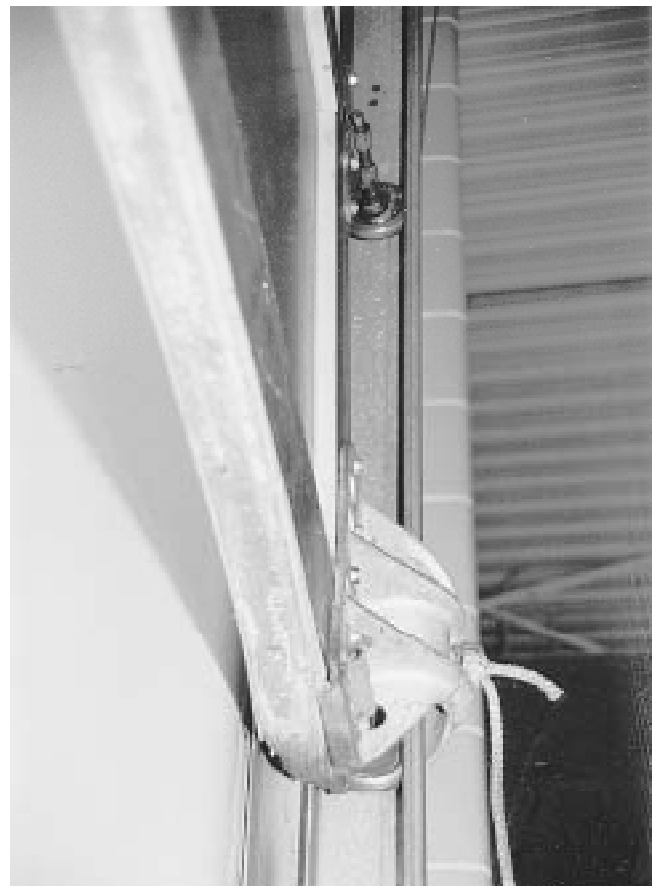
Fig. 1 Track for an overhead door The rollers hold the edge of the door away from the wall. You can seal the sides of this door with a fixed seal that slides against the face of the door opposite the rollers. Sides seals must be very flexible to accommodate looseness in the track and to minimize resistance to opening and closing.
