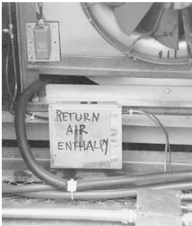
Fig. 1 The trouble with enthalpy control All the control lines have been disconnected from this enthalpy control unit, disabling the economizer cycle. The staff could not understand it, so they abolished it. In this case, much more information is required than simply labeling the control.
