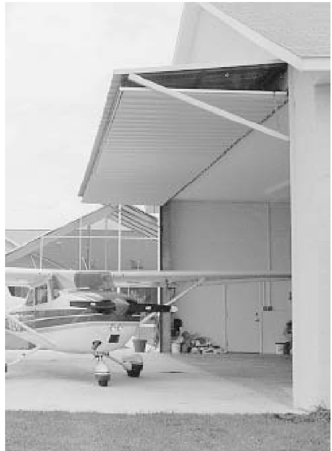
Fig. 4 A bi-fold door that wastes a minimum of height This proprietary design allows the door to open almost completely by using integral jacks at each side of the door. Most bi-fold doors cannot open fully because the lower panel must act as a brace against the door frame.
