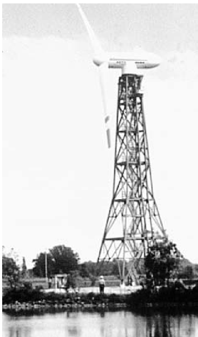
Fig. 7 Large wind generator This unit has a maximum capacity of several hundred kilowatts. The pitch of the blades is varied to maintain a fixed rotation speed when operating. The average output of this expensive machine is only a small fraction of its capacity. The placid water of the lake reveals a human weakness of wind power, which is a tendency to build windmills where there is insufficient wind to justify them.
