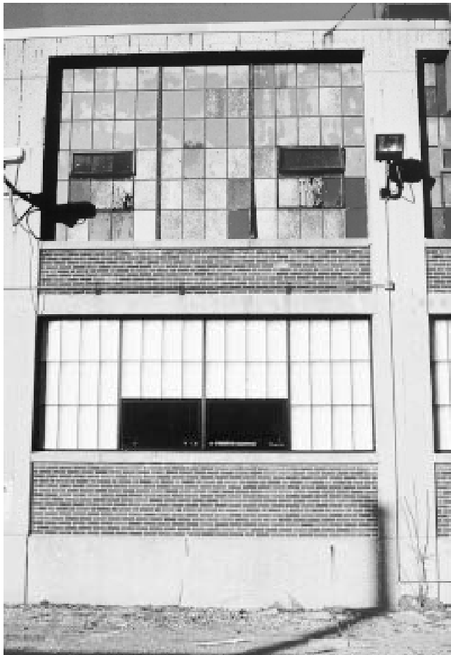
Fig. 1 Reduction of window area Most of the bottom window has been replaced with translucent insulated panels.
