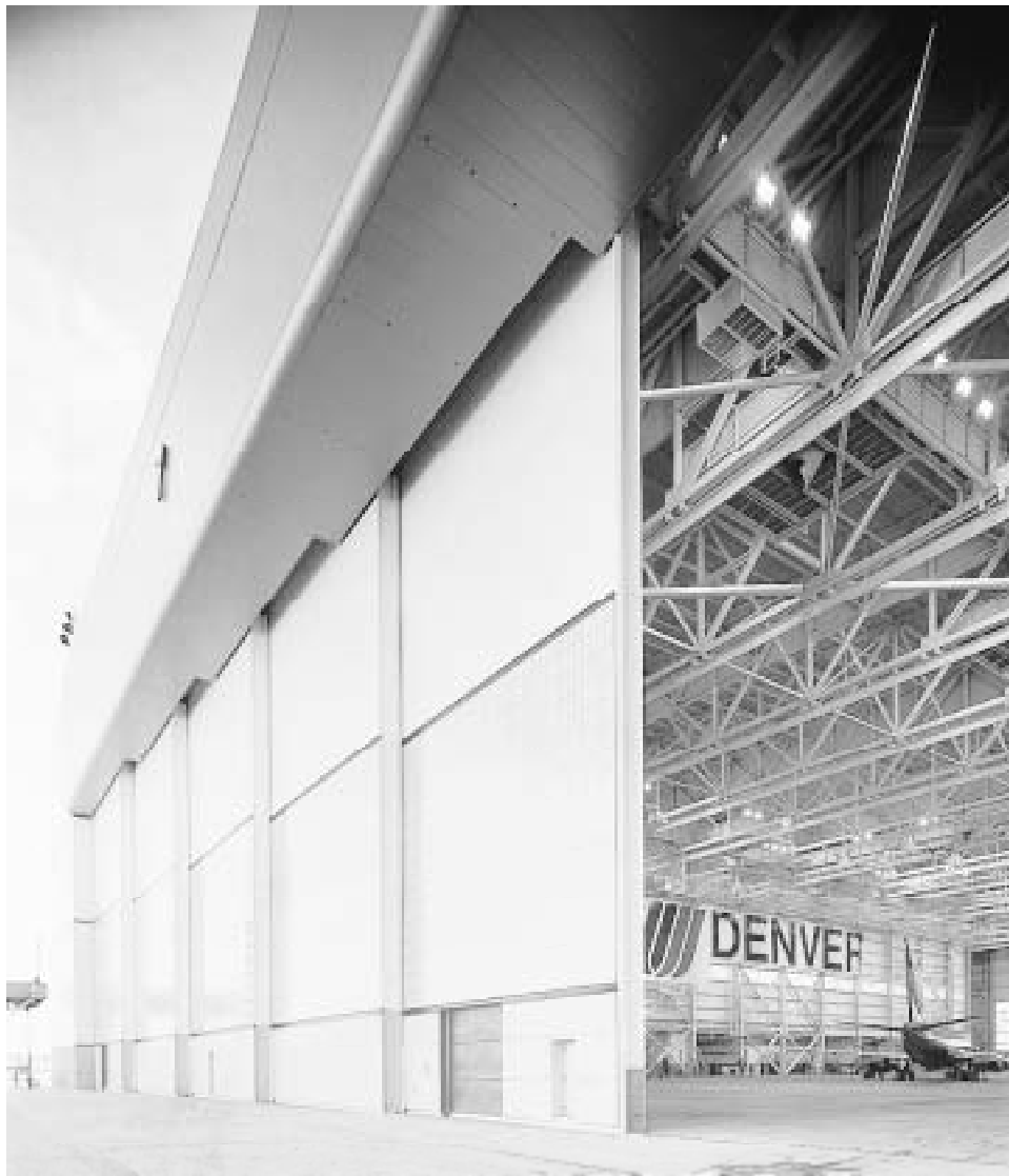
Fig. 1 Sliding doors At the top of the size range, sliding doors are about the only choice. In large sizes, it is easier to provide them with effective weather sealing and powered operators. Note how the structure at the top of the door is designed. This door is so big that it has two sizes of smaller doors at the bottom. The center panels in this door are box structures made of translucent material.
