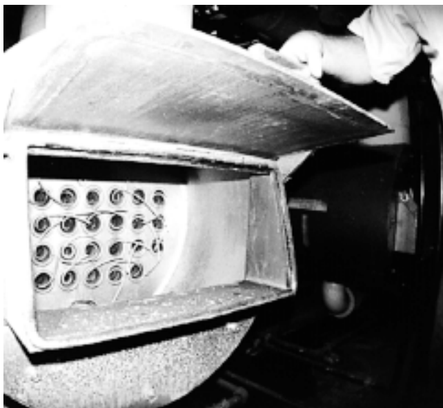
Fig. 2 Turbulators installed in a firetube boiler These turbulators are in the form of coils. They are kept from sliding into the tubes by pigtails that extend outside the tube sheet.
