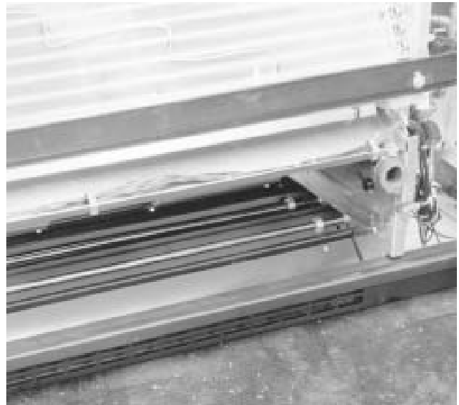
Fig. 4 Outside air dampers in a unit ventilator The long, slender blades are vulnerable to damage. Be sure that dampers operate freely and that they close tightly.
