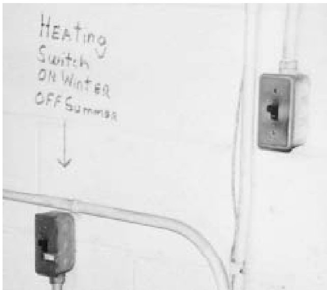
Fig. 2 Much better than nothing This sign is probably well attuned to the staff. It identifies the switch, and spells out the essential action. It should be more specific about time. It will survive until the next paint job.
