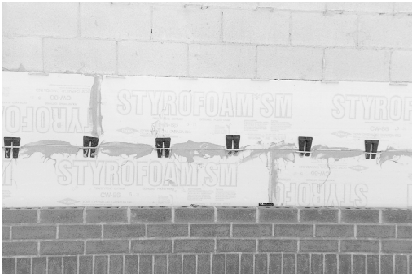
Fig. 3 Details matter The long-term reliability of this insulation job depends on holding the boards snugly against the concrete block wall. Note the clips installed for this purpose. Also, note the sealant that is installed between the joints. We hope that the sealant was installed between the boards, not just skimmed over the top.
