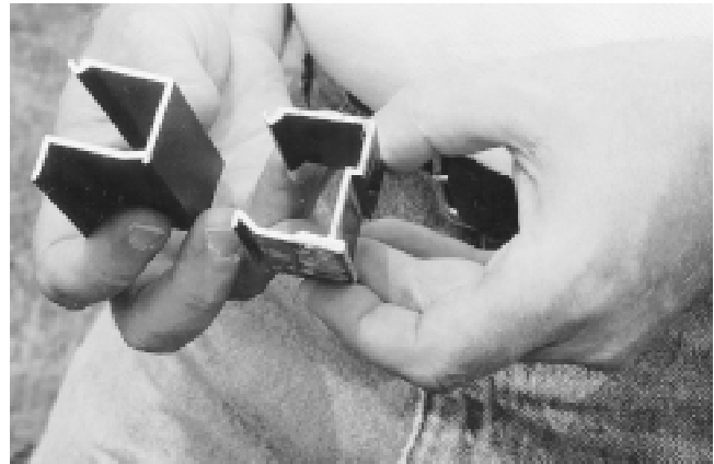
Fig. 3 Curtain wall clips The clip on the right held the original curtain wall panels in Figure 2. The clip on the left is for the new panels. There is a mature industry that is capable of making all the necessary components for replacement curtain walls.
