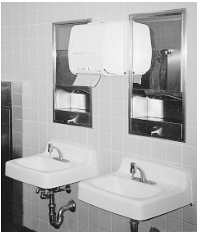
Fig. 2 An efficient type of faucet that is awkward to use These faucets require the user to push on a valve rod under the spigot. Foolproof in terms of water conservation. But, unfamiliarity and fear of contamination by other users discourage people from washing their hands.
