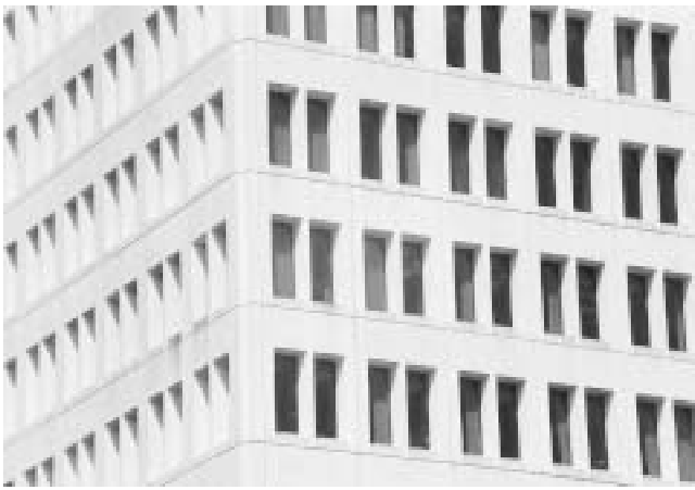
Fig. 6 Inset windows The shadow patterns show that deeply inset windows reduces solar heat gain. However, it cannot create satisfactory daylighting by itself.
