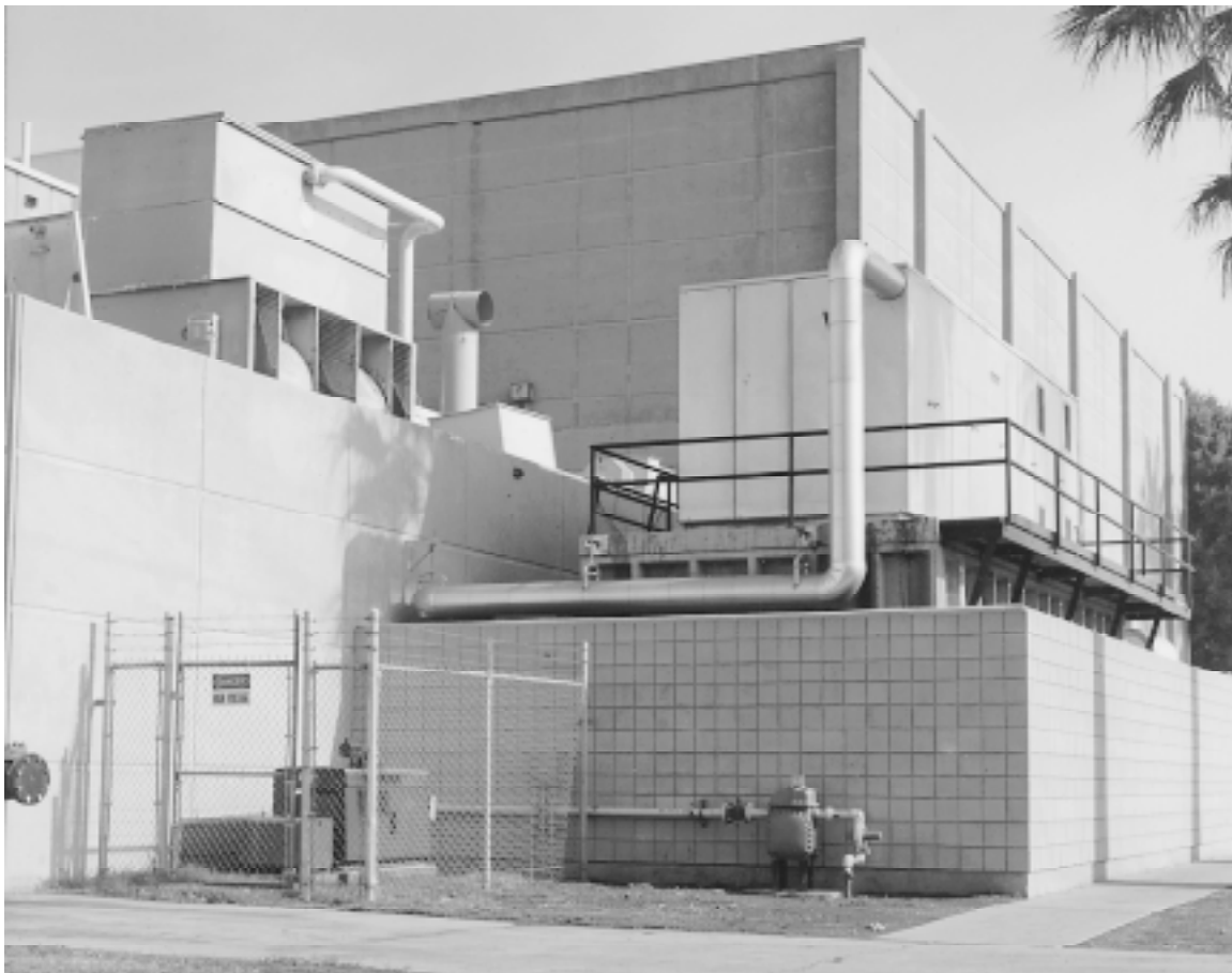
Fig. 5 Ice shedder system for a military club in Florida The compressor and evaporator unit, surrounded by the railing, sits atop a rectangular concrete ice tank. The cooling tower for the unit is at upper left.
