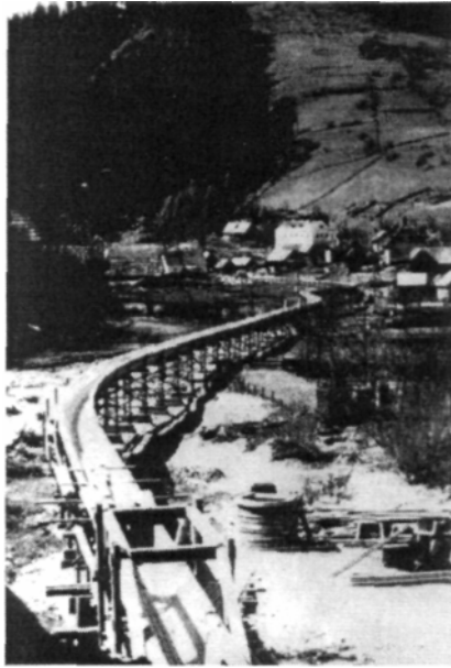
Figure 1.2: One of Schauburger's log flumes. Note the egg-formed section, and how the flume meanders like a stream. The Krampen-Neuberg flume in Austria, 1930s.
