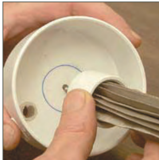
The pleated and rolled negative electrode, ready to install in the bottom cap.
