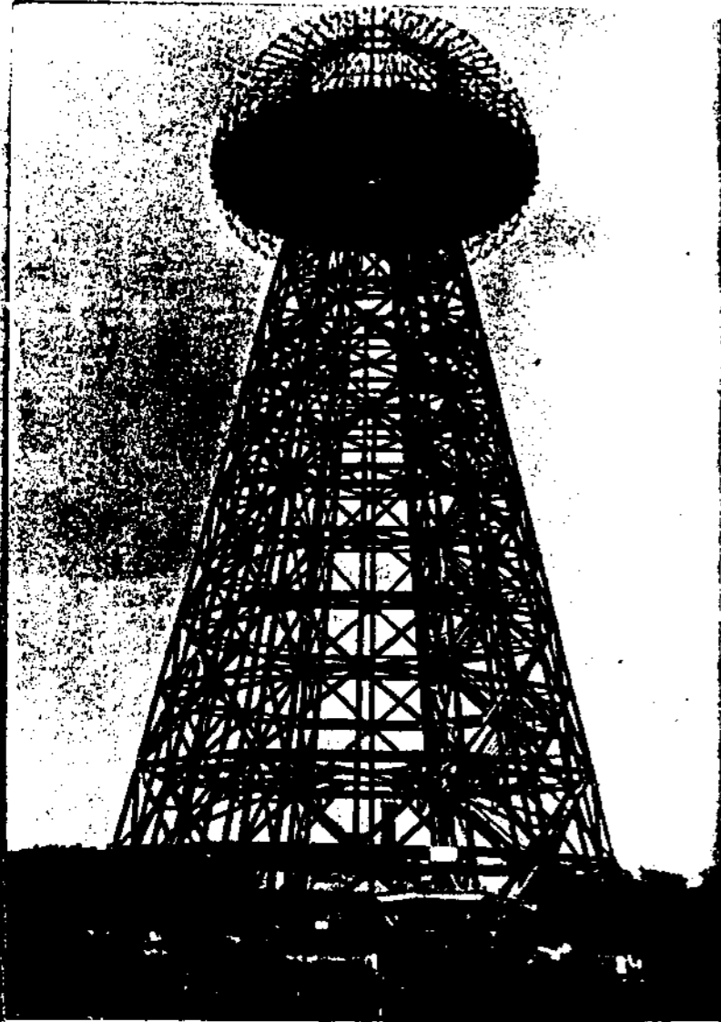
The ill-fated Wardencliffe tower built in 1901-03. It was intended for radio broadcasting and wireless transmission of power across the Atlantic. (Courtesy L. Anderson, after photo by Lillian McChesney)
