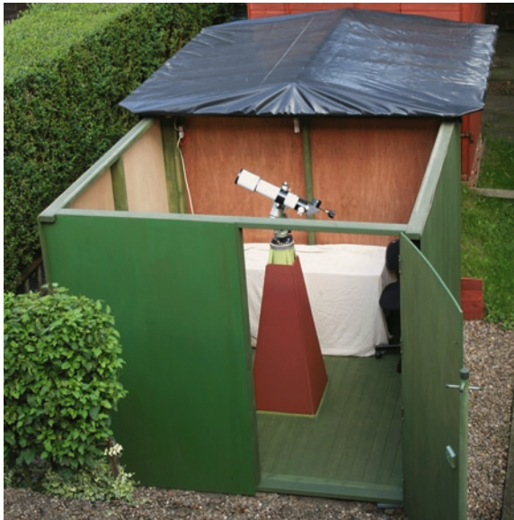
Fig. 7.3. Michael Clarke's roll-off roof observatory (Credit: Michael Clarke).
