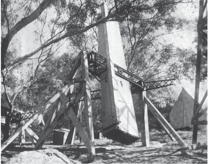
FIGURE 4-3. The wooden mount for a large camera used in photographing the 1922 eclipse from Australia.
