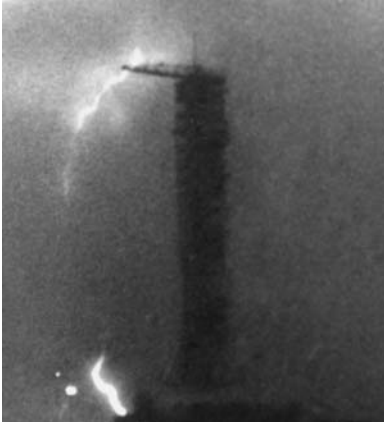
The launch tower hit by the same lightning discharge that disrupted Apollo 12.
