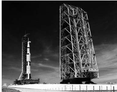
The mobile service structure near the Apollo 4 space vehicle.
