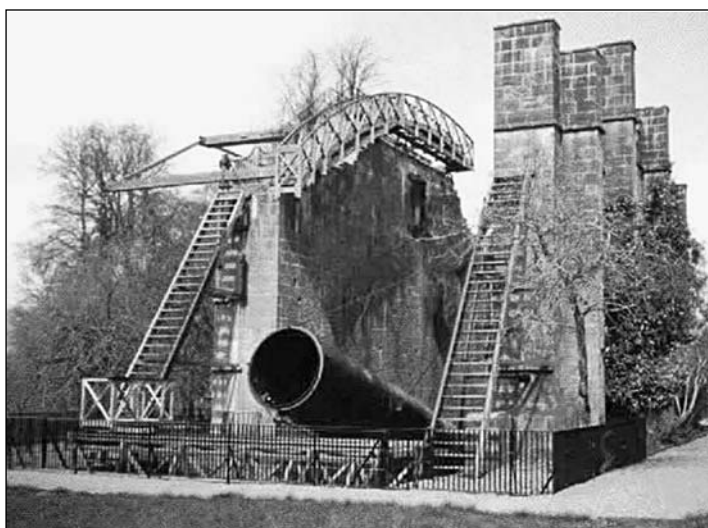
Figure 12. The “leviathan” was built by Irish aristocrat and amateur astronomer William Parsons, the third earl of Rosse. Parsons used it to discover several hundred star clusters and nebulae. It was not surpassed in size for seventy-five years, until the Hooker hundred-inch reflector was built on Mount Wilson in southern California.
