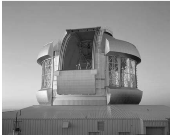
Figure 2.15. The Gemini North Telescope on Mauna Kea, in Hawaii, showing the open sides which help to minimise local turbulence. (Reproduced by permission of Neelan Crawford, courtesy of Gemini Observatory/AURA)
