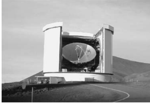
Figure 2.12. The James Clerk Maxwell Telescope, operating at sub-mm wavelengths, is located on Mauna Kea in Hawaii at an elevation of 4200 m. Although this is a radio telescope, it is housed in a dome and, under normal operating conditions, the dome opening is covered by a protective cloth membrane that is transparent at the operating wavelengths. Contrast this image to the Arecibo radio telescope that operates at longer wavelengths, shown in Figure 2.6.a, which is at an altitude of only 497 m. (Reproduced by permission of Robin Phillips)
