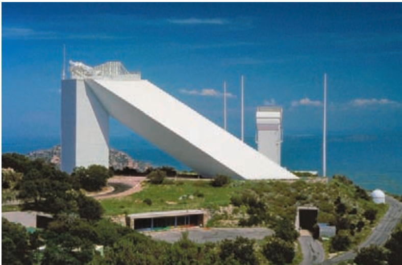
Fig 6.6. Solar telescope on Kitt Peak (operated by NOAO). The telescope has a very long focal length, so that two can produce a large image and study the detailed appearance. Since the tube is so long, it is not reasonable to move it. Instead, the large mirror at the top (the objective) is moved to keep the sunlight directed down the tube. [NOAO/AURA/NSF]
