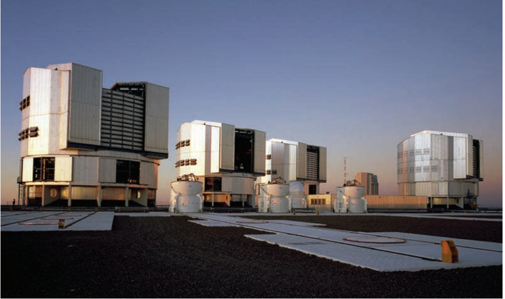
Figure 5.17 The four 8.2-m telescopes of the VLT, with the four 1.8-m auxiliary telescopes in the foreground. Image: Courtesy of the European Southern Observatory.
