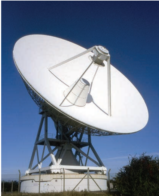
Figure 5.22 The 32-m Cambridge Telescope – a Cassegrain design. The cone houses a carousel supporting four receivers. Image: Ian Morison.
