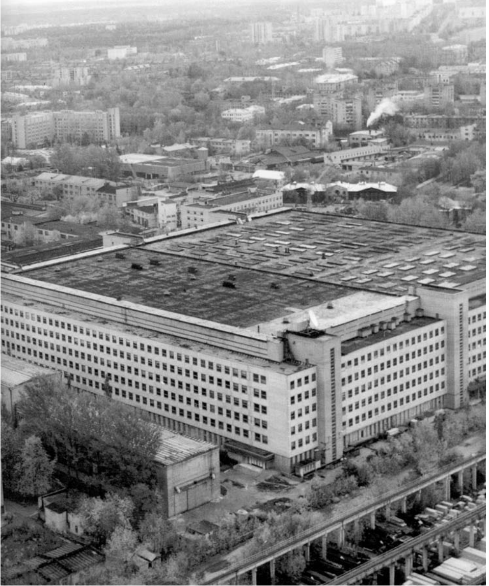
The TsKBEM building at Kaliningrad, Moscow.
