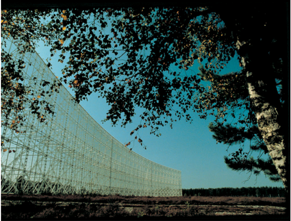
Figure 8.11. The spherical array of the great Nançay (Sologne) radio telescope, which is used for both transmission and reception in the search for extraterrestrial civilisations. (Courtesy J. Bérezné, CNRS.)
