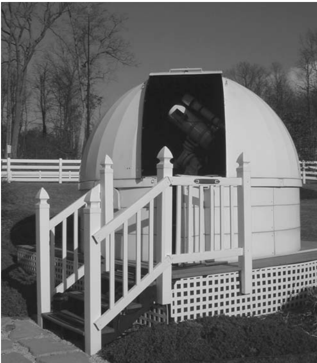
Figure 9.47. Platform and steps.
