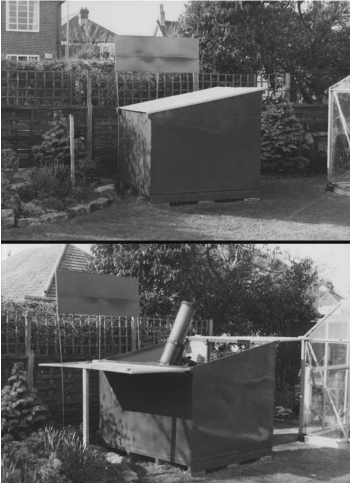
Figure 3.7. My first observatory, a 1.5 m (5 ft) square hinged roof structure, built in 1981 (The board at the back was to screen a streetlight).
