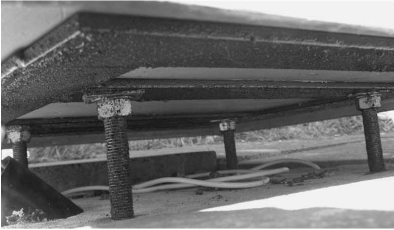
Figure 9.58. Steel baseplate supported on bolts.
