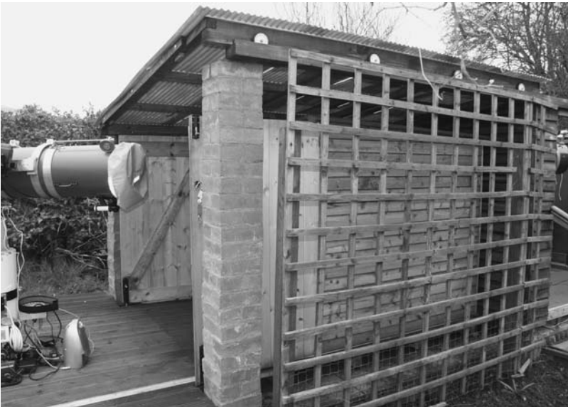
Figure 9.31. With both telescope sheds open, the run-off shed, behind the trellis, fits under the roof of the run-off roof shed
