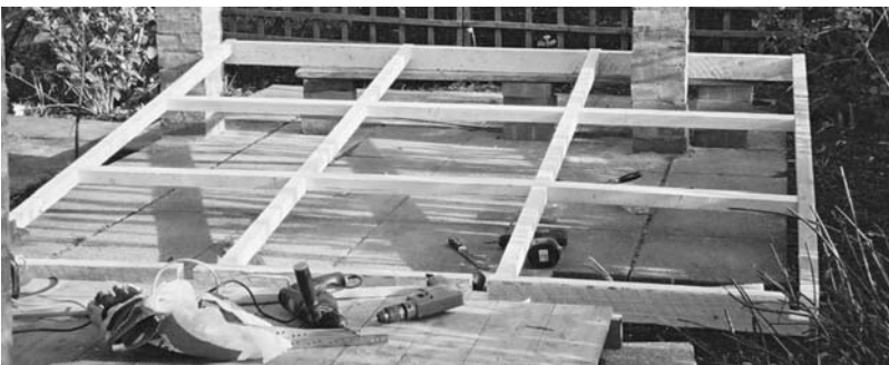
Figure 9.23. Constructing the roof framework.
