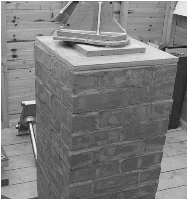
Figure 5.2. Earlier brick pier in my observatory.
