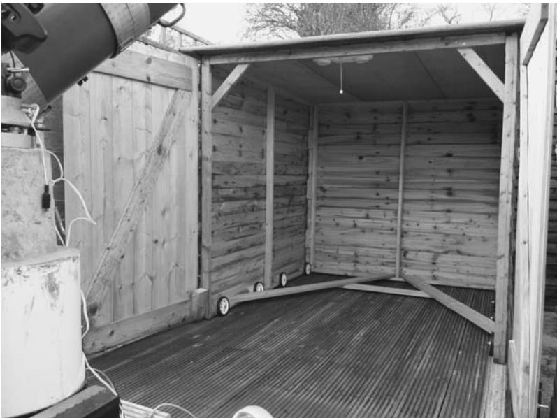
Figure 9.33. Looking into the run-off shed, showing diagonal bracing.
