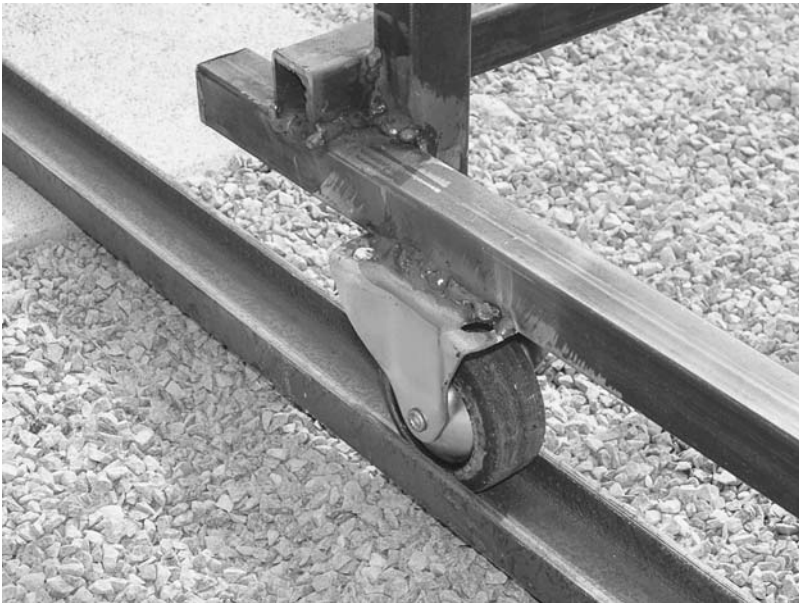
Figure 5.4. Jointing in a welded-steel run-off shed framework.
