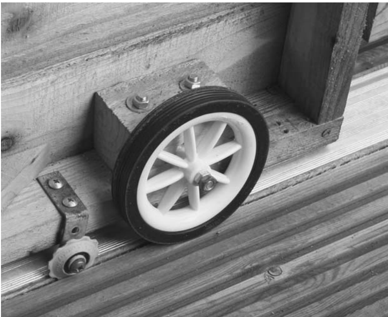
Figure 9.32. Detail of the run-off shed, showing one of the running wheels, one of the jockey wheels, and the aluminium strip.
