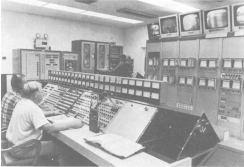
FIGURE 20-3. Control room (inside a reinforced concrete blockhouse) for test operators, instrument recorders, and controls. Note the control console, closed-circuit television, radio and telephone, direct read-out meters, strip charts, high-speed tape recorders, oscilloscope, air-quality alarm, and emergency lights. (Courtesy of U.S. Air Force Phillips Laboratory.)
