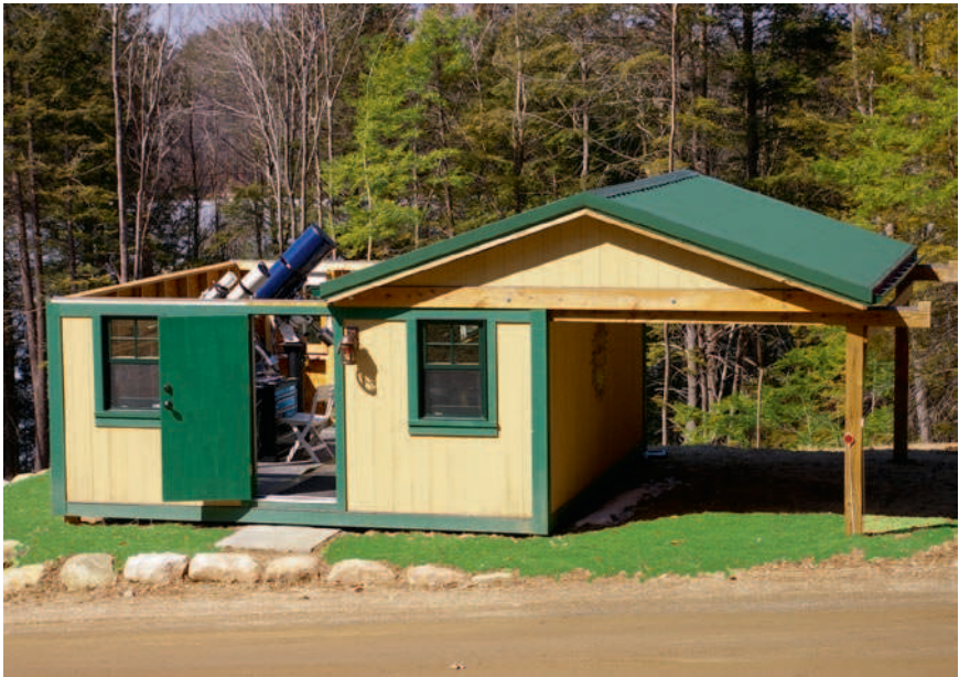
Fig. 14.2. Backyard observatories built this roll-off roof observatory for the author in 4 days. The open area contains two piers. A small warm room is on the right.
