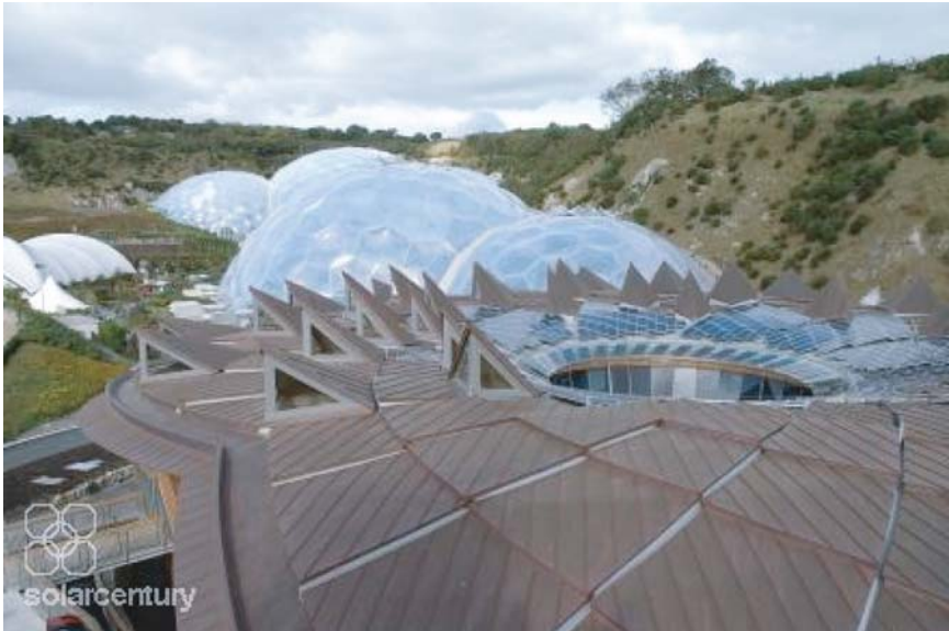
Fig. 8.5 The Core, Eden Project, Cornwall, UK. The solar energy roof has a Fibonacci Series design embodying 40 and 80 W PV panels and producing an estimated 20,000 kWh a year (Courtesy of solarcentury)
