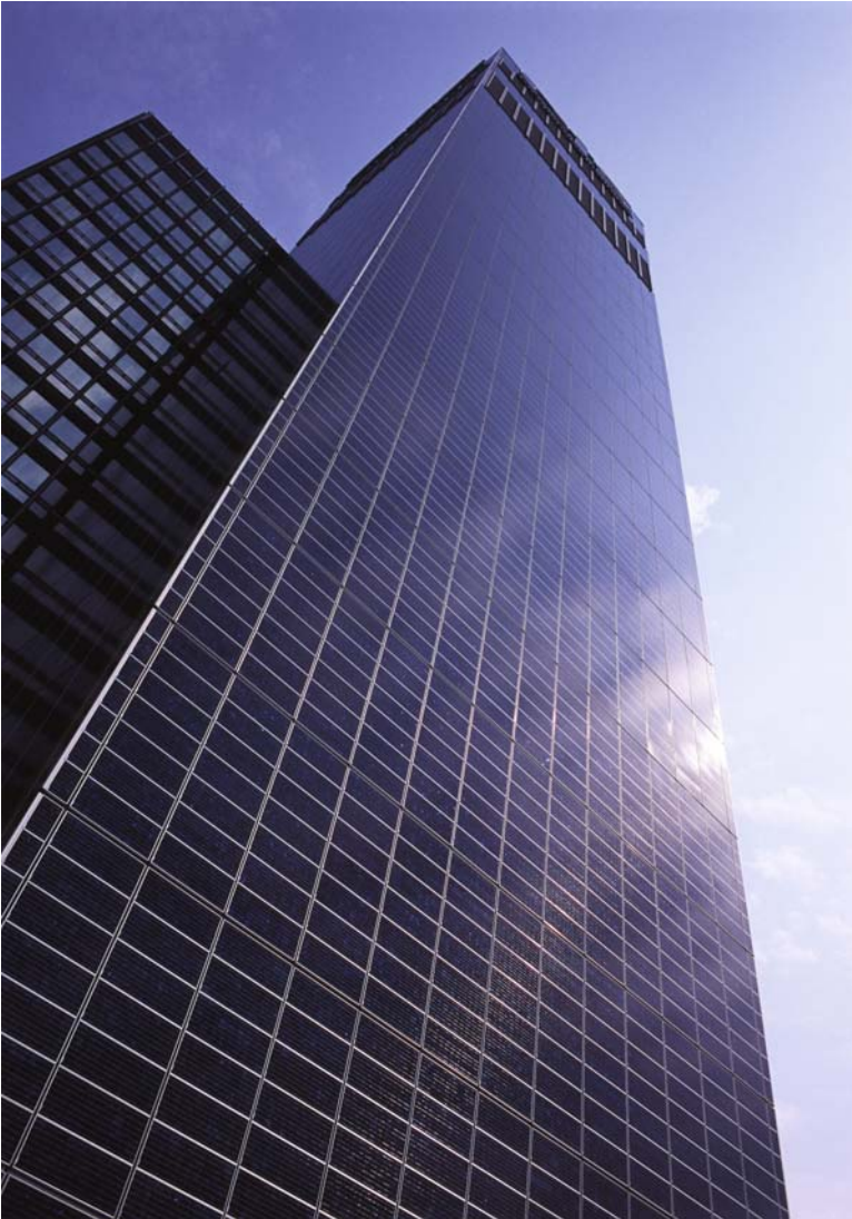
Fig. 8.6 The south façade of the CIS Tower in Manchester, UK, resurfaced in 2005 in PV panels which generate over 180,000 kWh a year (Courtesy of solarcentury)
