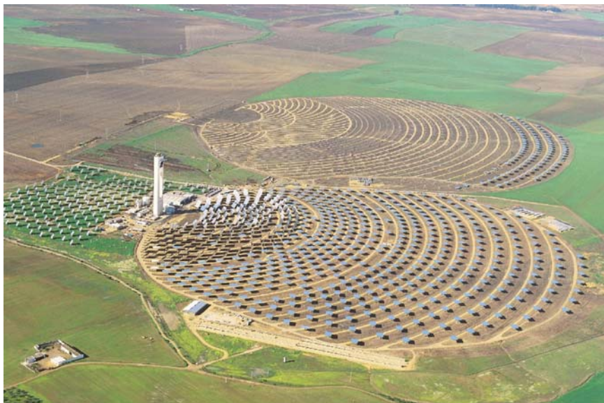
Fig. 8.4 11 MW Solar Platform at Sanlúcar la Mayor, Spain, first part of a 300 MW installation using a wide range of solar technologies, to be completed in 2013
