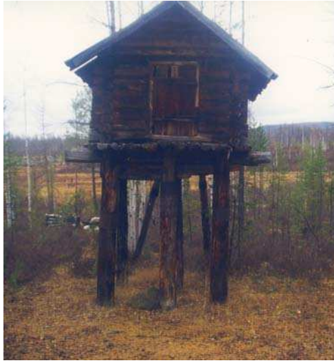
FIGURE 3.6. A labaz (storehouse on poles) built in the course of the second Kulik expedition (1928) (Credit: Dr. Gottlieb Polzer, Lichtentanne, Germany.).
