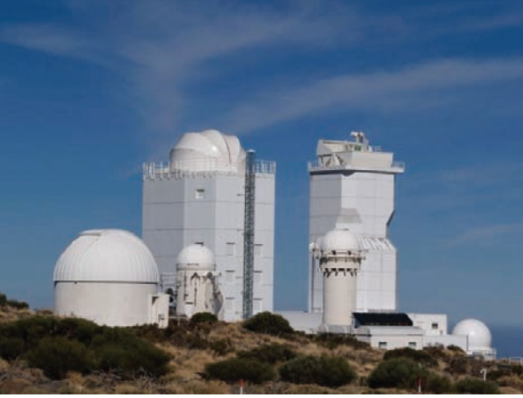
Fig. 3.11 The Observatorio del Teide in Spain, Tenerife. The coelostat mirrors have a diameter of 80 cm, the main mirror in the vertical evacuated tank 70 cm. The telescopes are operated by Germany (KIS, AIP, Göttingen) and Spain (IAC)
