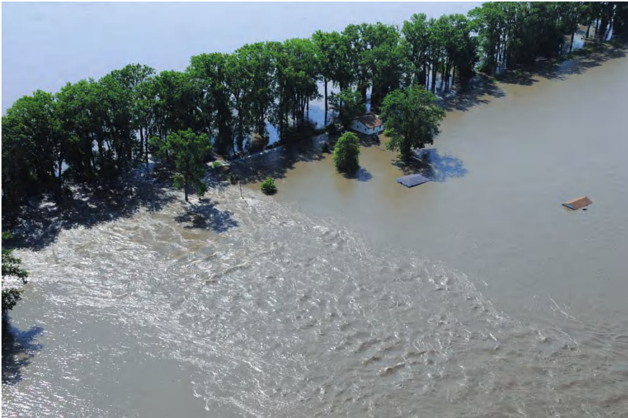
A levee on the Mississippi River being overtopped, with water flooding farmlands in Winfield, Missouri, during Midwest floods of summer 2008 (T. Kusky)
