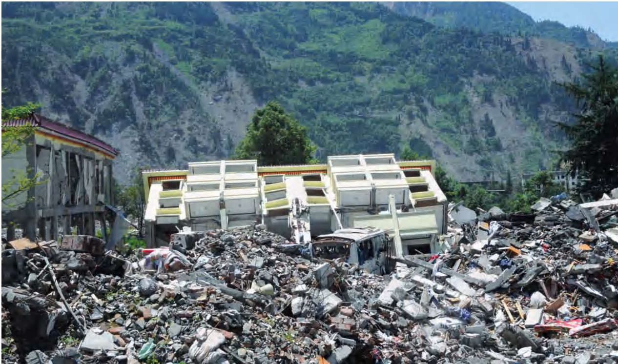
Damage from ground shaking and liquefaction in Yingxin, Sichuan Province, China, causing buildings to collapse on their sides, from May 12, 2008, magnitude 7.9 earthquake ( T. Kusky )
