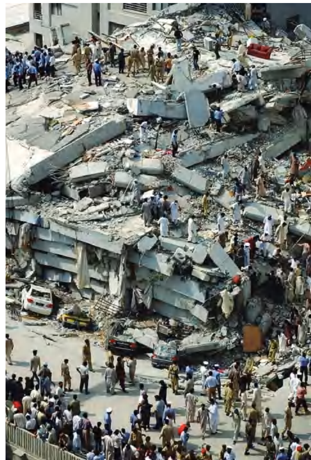
Collapsed 10-story apartment building in Islamabad, Pakistan, after earthquake October 8, 2005: The building pancaked as one floor fell, thereby causing each lower floor to collapse. (AP images)
