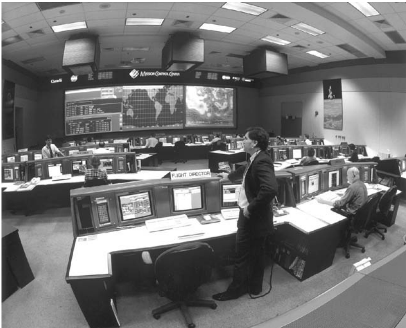
Figure 9. The Control Room in Building 30S layout is functionally very similar to the earlier MCC (shown here for Shuttle operations). The Flight Director's console is typical of the new MCC, and it features CRT displays with color graphics and a digital intercom control panel (photo courtesy of NASA-JSC#S95-11222). This figure is available in full color at http://www.mrw.interscience.wiley.com/esst .
