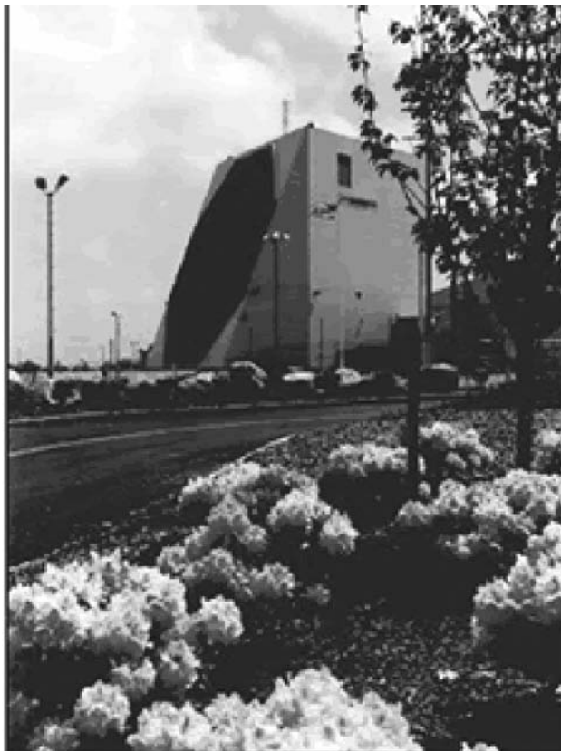
Figure 10. The Space Surveillance Network is composed in part of ground-based radars, like this precision acquisition vehicle entry and phased array warning system (PAVE PAWS), which detects and tracks sea-launched and intercontinental ballistic missiles. Their secondary mission is to track objects in space. Figure courtesy USAF Space Command. Picture can be found at http://www.peterson.af.mil/hqafspc/library/FactSheets/FactSheets.asp?FactChoice=15 . This figure is available in full color at http://www.mrw.interscience.wiley.com/esst .
