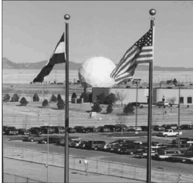
Figure 11. PIKE, a Remote Tracking Station at Schriever AFB, Colorado, looks like a giant golf ball to casual observers. PIKE is operated by the 22nd Space Operations Squadron. Figure courtesy USAF Space Command. Picture can be found at http://www.peterson.af.mil/hqafspc/Library/almanac/pg12/almanac_12.htm . This figure is available in full color at http://www.mrw.interscience.wiley.com/esst .
