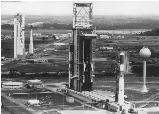
Figure 5. ELA 1 and ELA 2 launch sites. ELA 1 site (foreground): Ariane 3 launcher during third-stage fueling tests on day D – 9. At rear: Ariane 4 launcher recently arrived on the ELA 2 pad. Note the double rail track between the pad and the preparation zone (background). The white circle midway down the rail track is a turntable, used to allow two launchers to pass each other if necessary. This figure is available in full color at http://www.mrw.interscience.wiley.com/esst .
