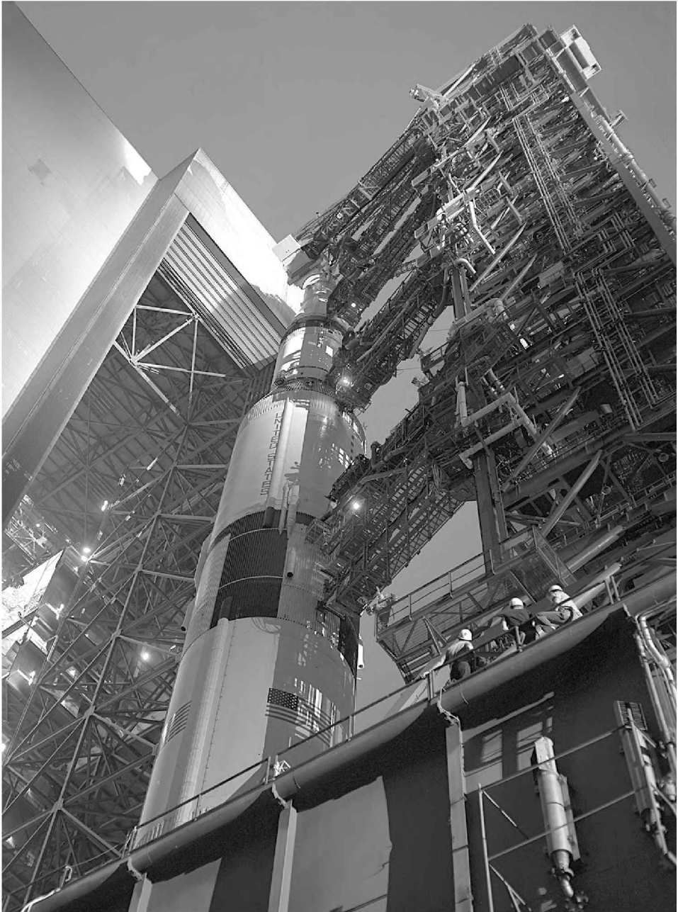
The largest rocket ever brought to operational status, the Saturn V departs the world's largest single-story structure, the Vehicle Assembly Building. The sheer enormity of both is amply illustrated by the technicians at the centre-right of the image.
