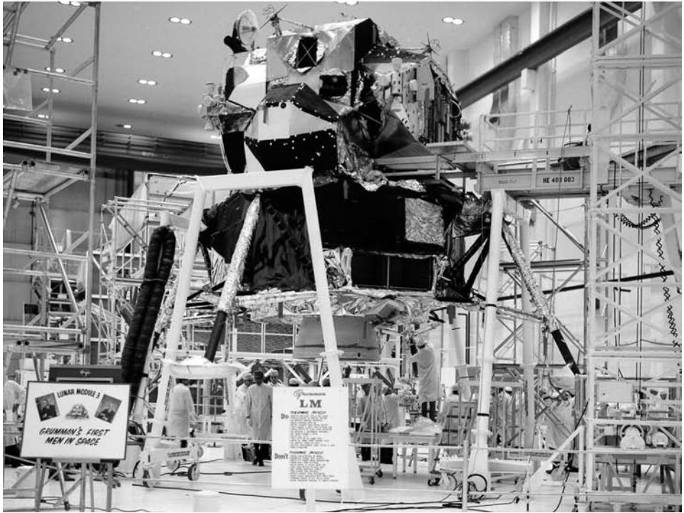
Preparing the CSM-104 and LM-3 spacecraft for the Apollo 9 mission.
