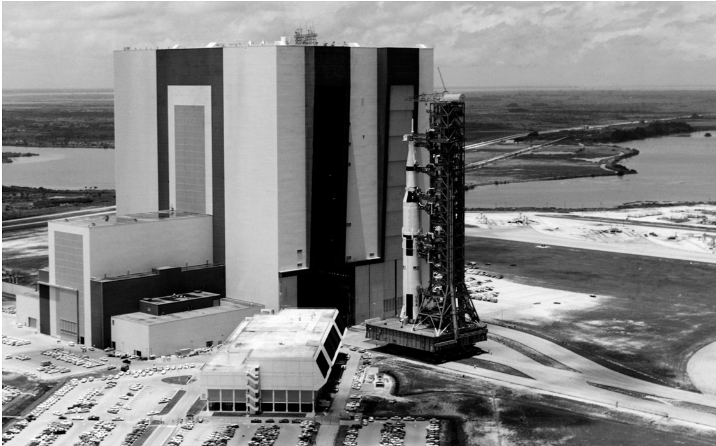
On 20 May 1969 the Apollo 11 space vehicle emerges from the Vehicle Assembly Building.
