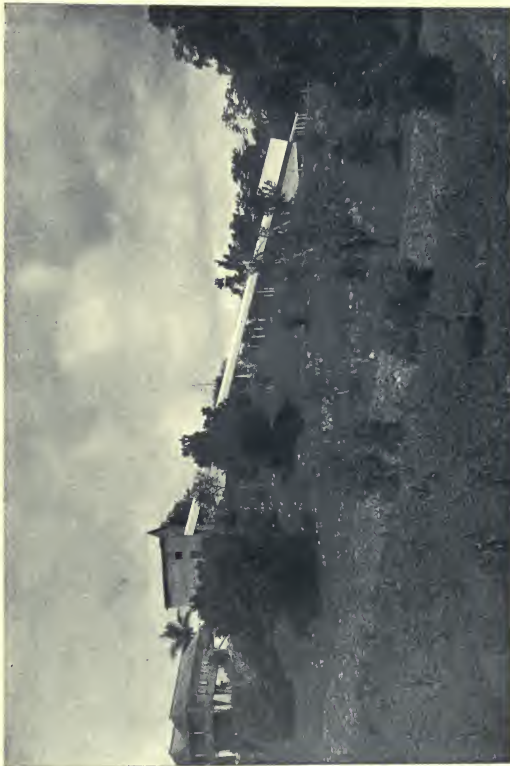
THE JAMAICA TELESCOPE The instrument with which the photographs and many of the observations were made. The observer, seated in the small upper building, looked down through the white tube toward the lower building, where the Moon appeared to him
