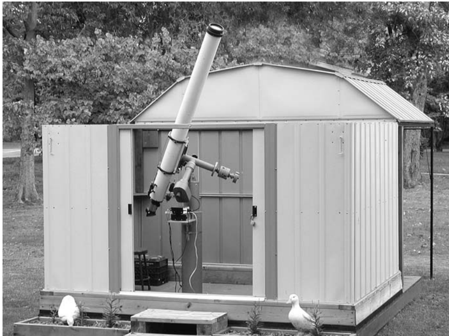
Figure 2.6. A suitable alternative to domed observatories, which tend to offer poor daytime seeing, is the roll-off roof design.
