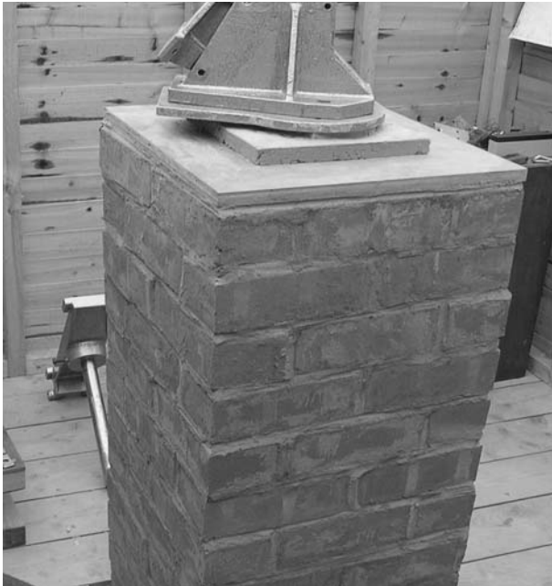
Figure 5.2. Earlier brick pier in my observatory.
