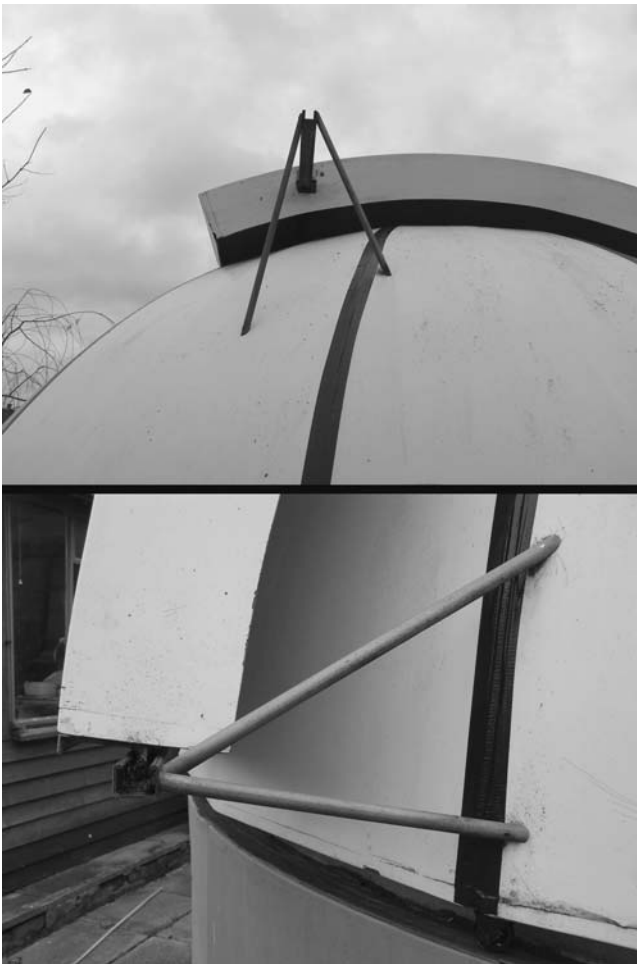
Figure 9.37. The struts for the dome tracks at the top and bottom of the shutters.
