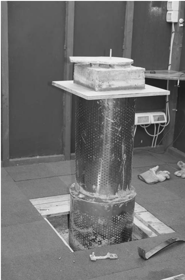
Figure 5.1. Telescope pier in my observatory, cast in concrete in two stainless steel cylinders (bins), with plywood shelf, and aluminium platform set in the top.
