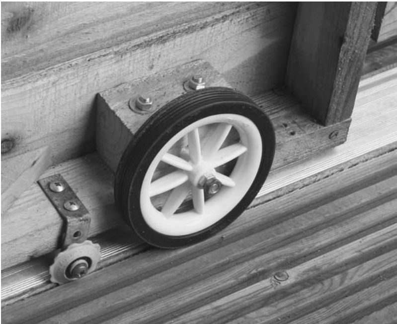
Figure 9.32. Detail of the run-off shed, showing one of the running wheels, one of the jockey wheels, and the aluminium strip.
