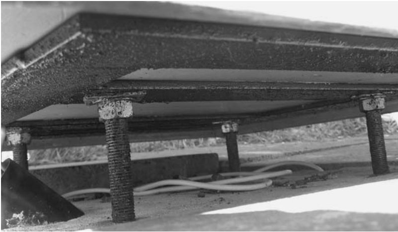
Figure 9.58. Steel baseplate supported on bolts.
