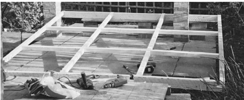
Figure 9.23. Constructing the roof framework.
