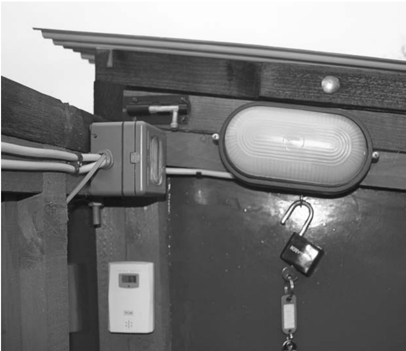
Figure 7.2. External sealed light fitting and switch.
