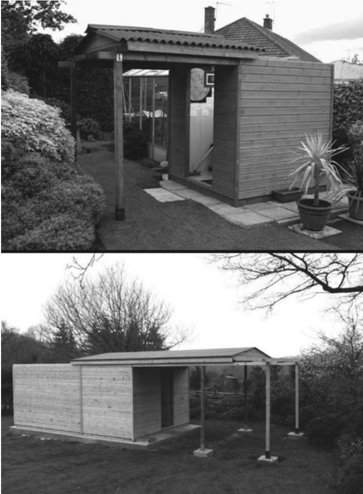
Figure 3.6. Two run-off roof designs manufactured by Alexanders Observatories of England, a small 2 m (6 ft) square example, and a large 4.8 × 3 m (16 × 10 ft) observatory with a warm room.
