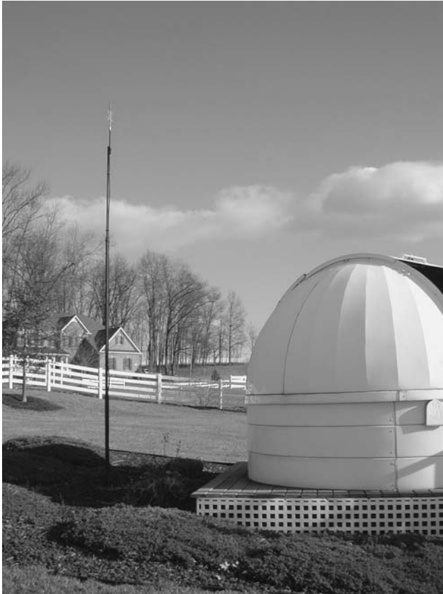
Figure 9.48. Lightning conductor.
