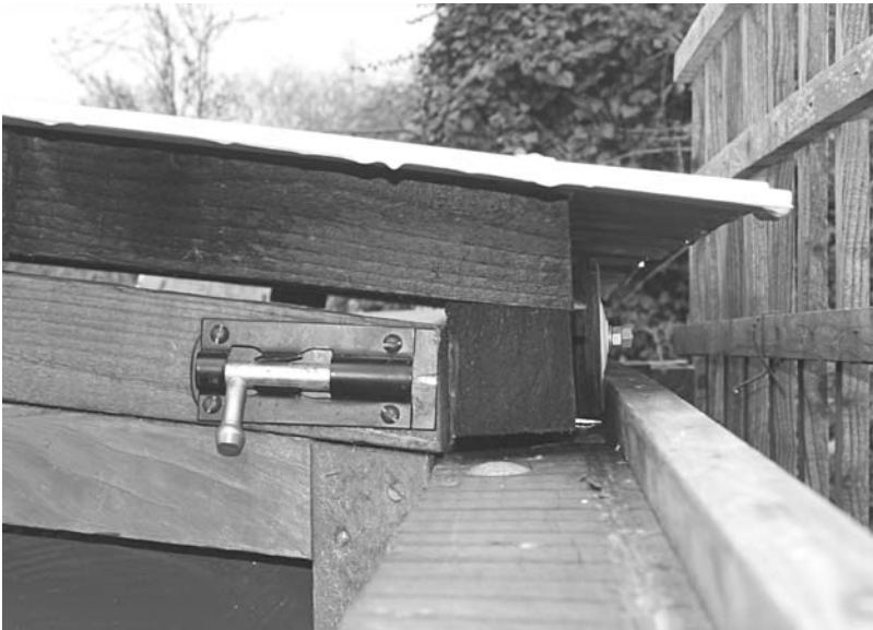
Figure 9.21. Detail of the run-off roof and rail construction, with one of the securing bolts.
