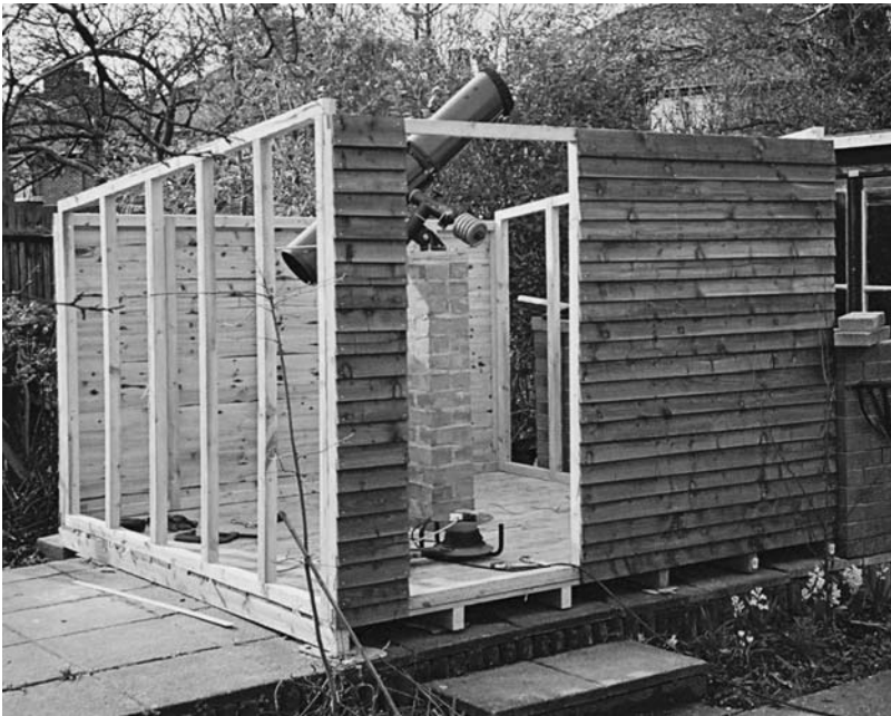
Figure 9.22. Shed partially assembled, showing unclad wall-frames, and 6.25 in. telescope experimentally in place on the first, unsuccessful, pier.
