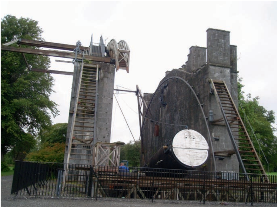
Fig. 6.14. Restoration almost complete, August 2008.
